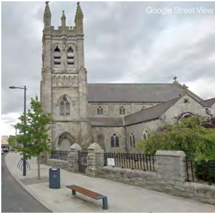
View of entry point via Bridge Street.
