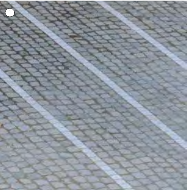
LOW CONTRAST GRANITE PAVING BANDS
