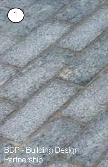
GRANITE PAVING USED IN PHASE 1 SCHEME
