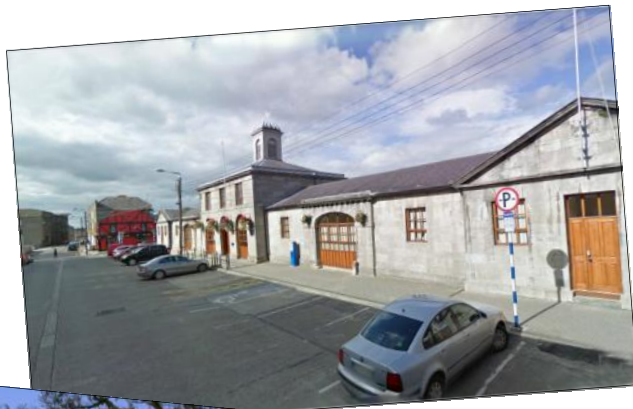
▲ Civic Centre, Fair Street, Drogheda, County Louth.
