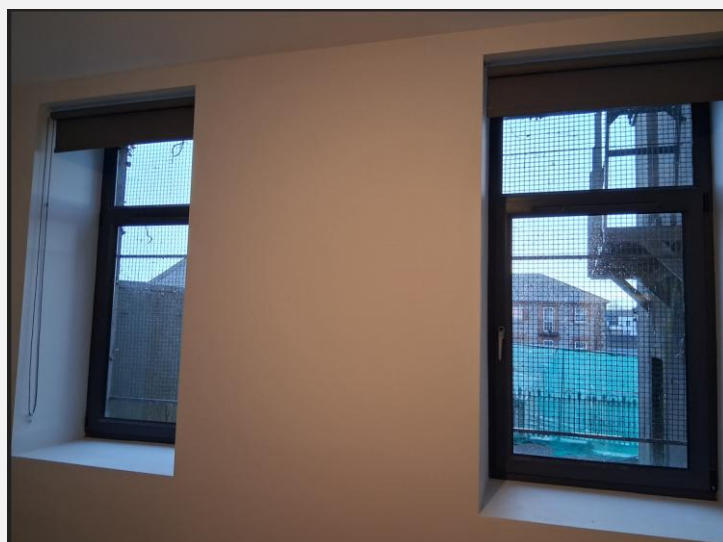
Interior as existing
