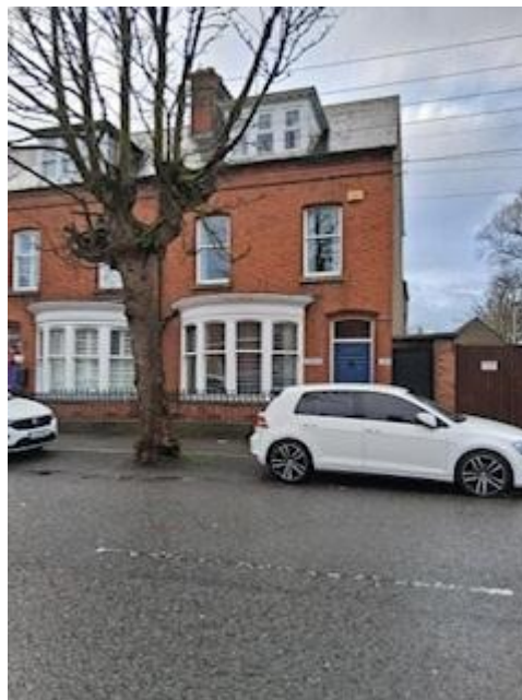
Figure 2: Existing property exterior
