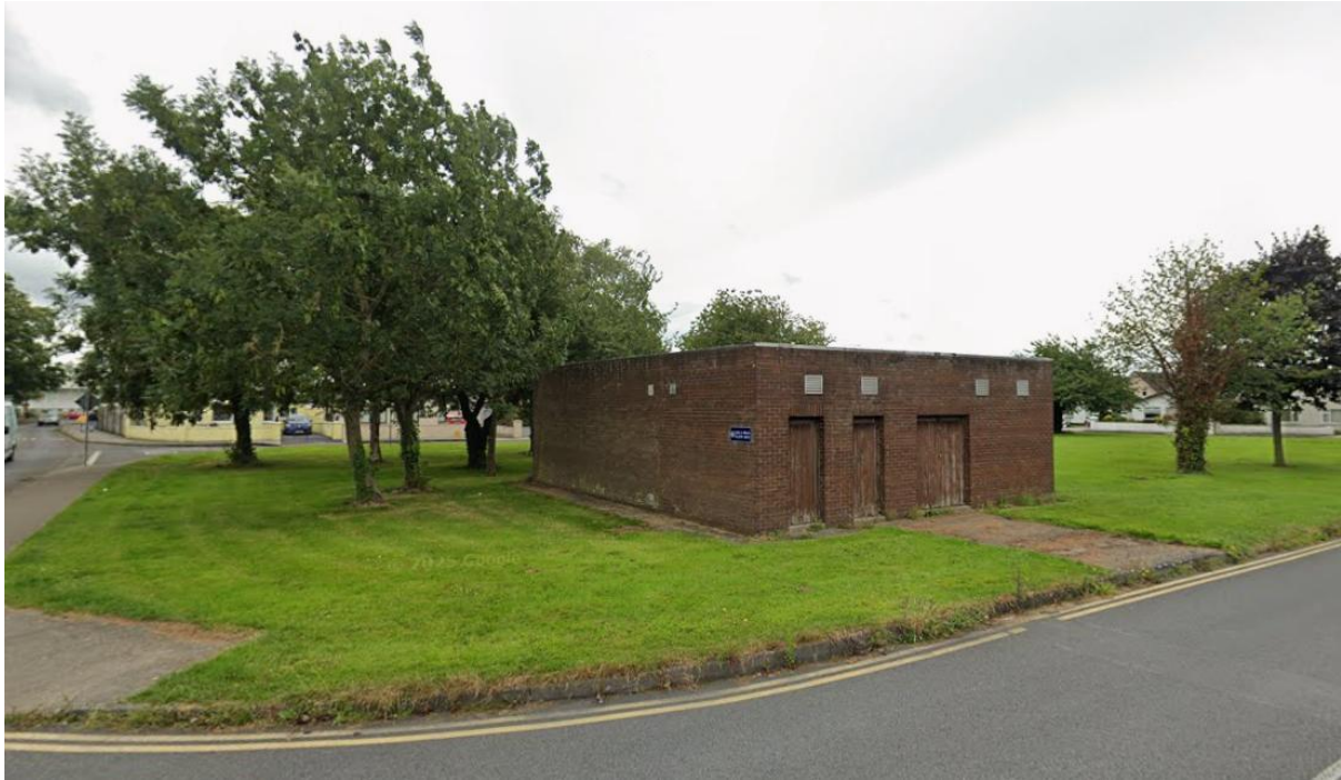
Existing view of the disused pumping station.
