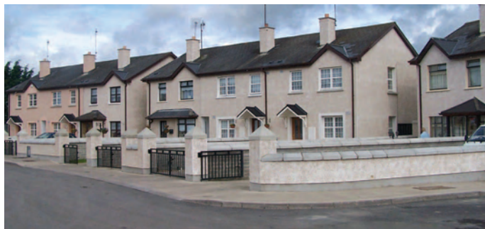
Remedial Works Scheme at St. Finians Park, Drogheda
