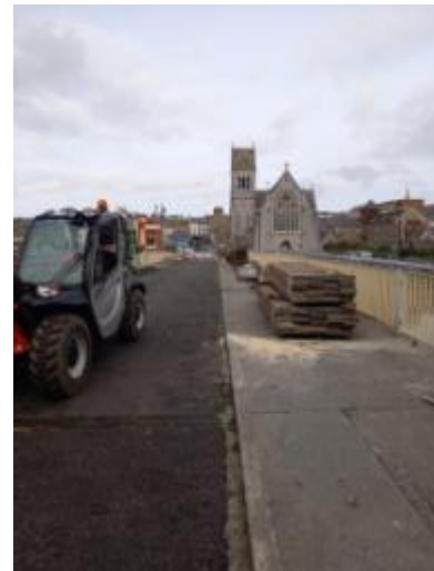
St. Dominick's Bridge - Contractor setting up on site
