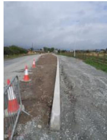
Footpath & cycle lane construction progress
