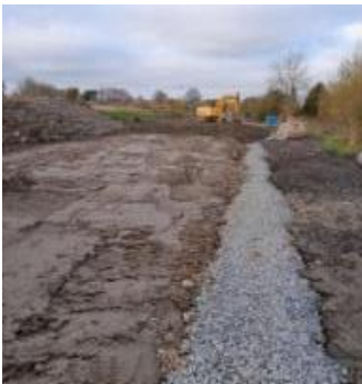
Backfilling of Pipeline
