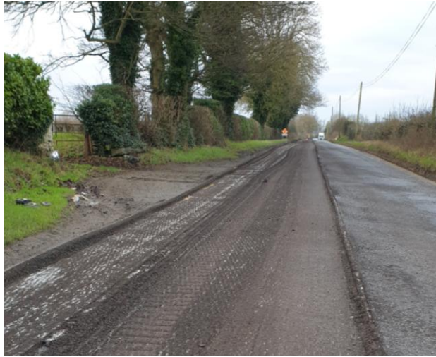
N52 Ardee to Kells Road 800m of resurfacing works underway
