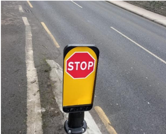
Flexi Stop Bollard installed at Cromwell Lane
