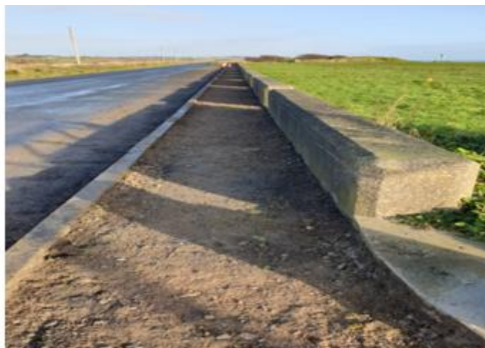
New footpath under construction at Port Beach
