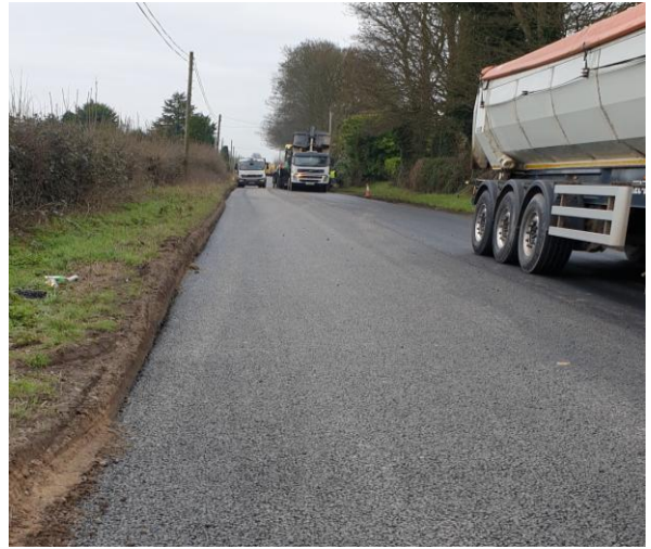
N52 Ardee to Kells Road 800m of resurfacing works final completion
