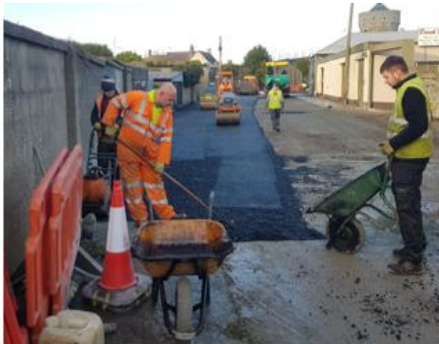
Drainage works at Sarah Gibney Lane
