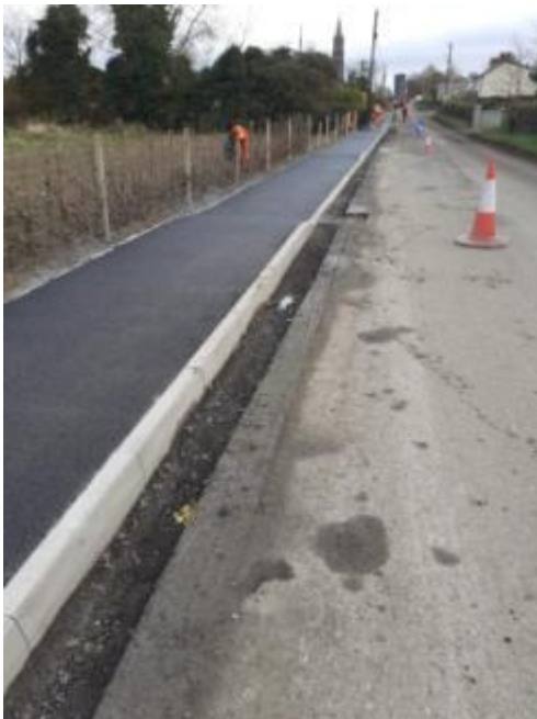
Stabbannon Footpath- Works in Progress
