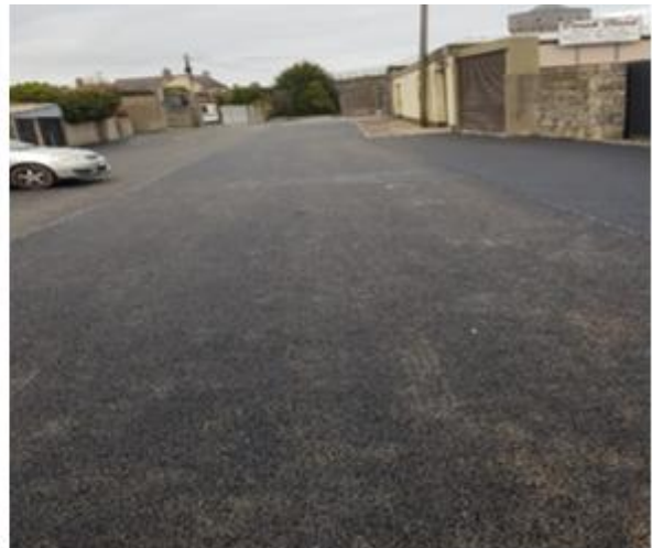
Completed works at Sarah Gibney Lane
