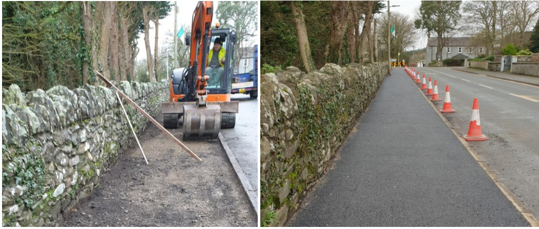
Footpath construction and completion at Termonfeckin Village
