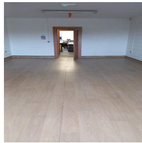
Capital Works at Lourdes Stadium
