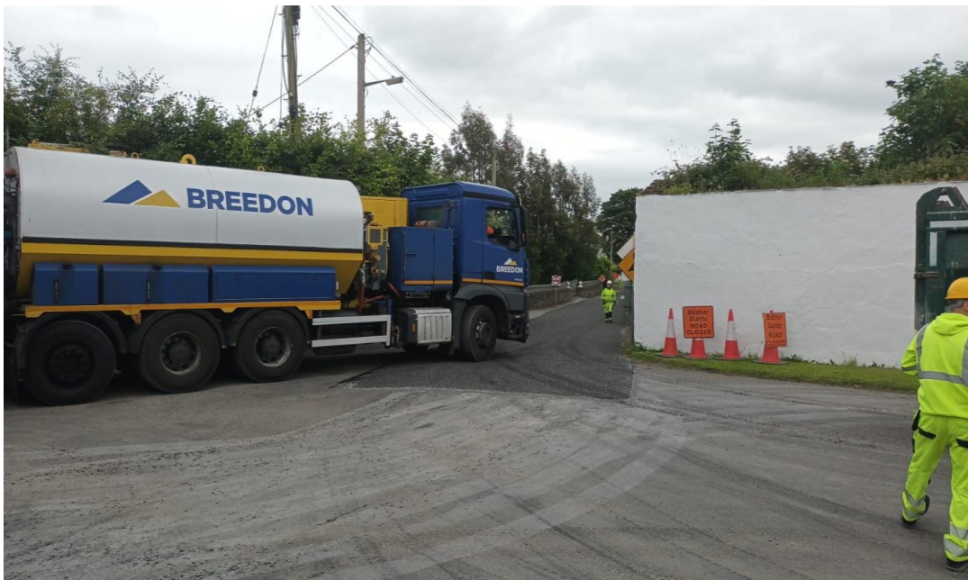
Resurfacing works at Kilkerry
