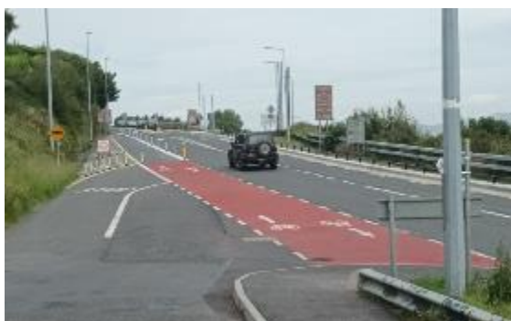
Section of Greenway at Back Lane Carlingford.
