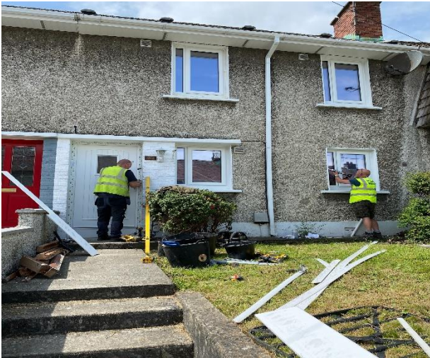
Energy Retrofitting works taking place at Ascal a Haon, Yellowbatter, Drogheda
