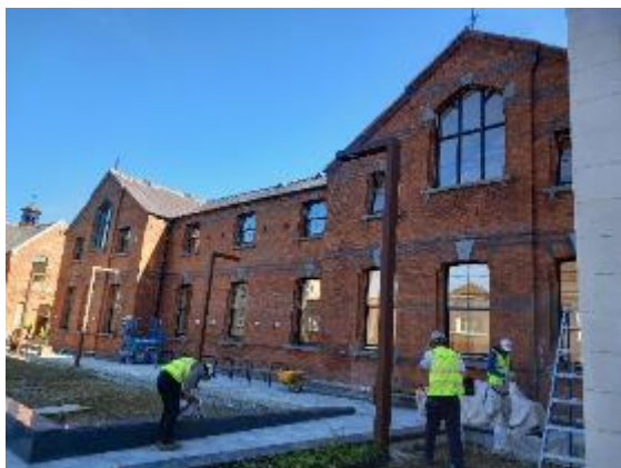
Block Community Services Building
