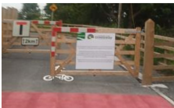
Greenway access control point and signage
