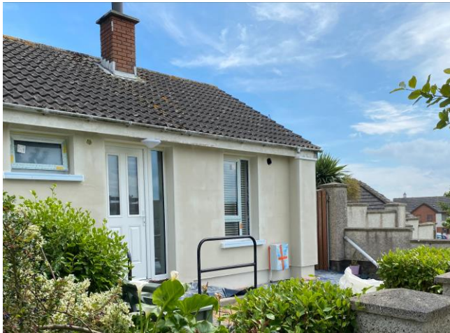
External wall insulation at John Kirk Park, Clogherhead
