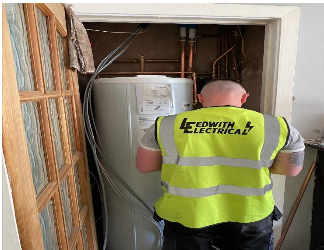
Heat pump installation at Ascal a Haon, Yellowbatter, Drogheda in June
