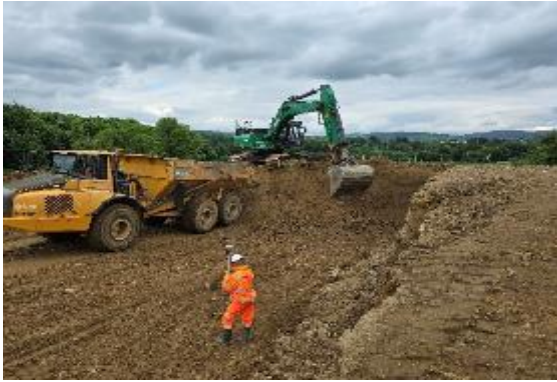
Earthworks Cut commencing.
