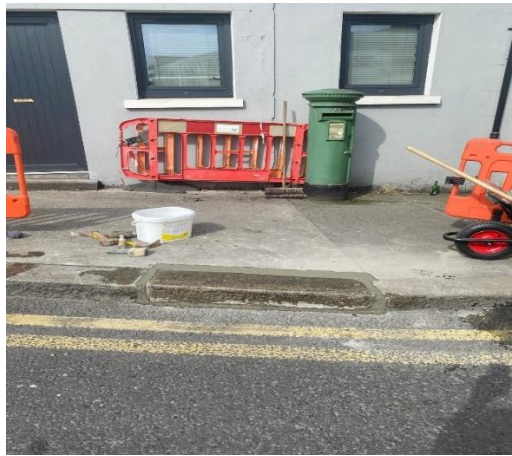
Footpath repairs at St. Mary's Street
