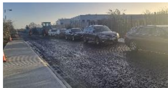
New carriageway with footpaths
