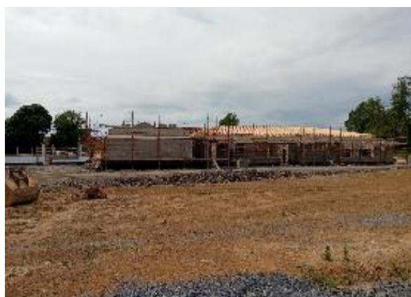
Roof structure commencement
