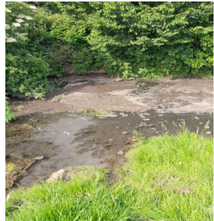
Slurry in a drain
