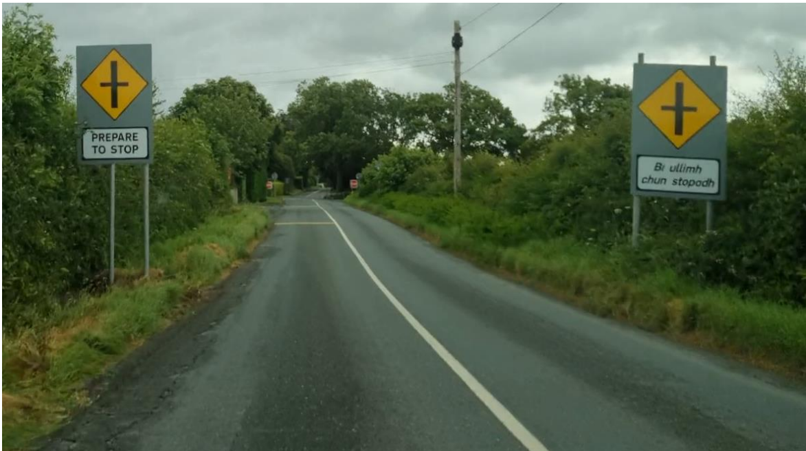
New Junction signs on the LP-2308-24 Cockle Road
