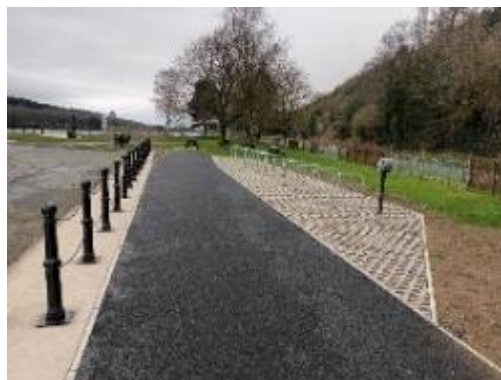
Works Complete in Victoria Lock in NI
