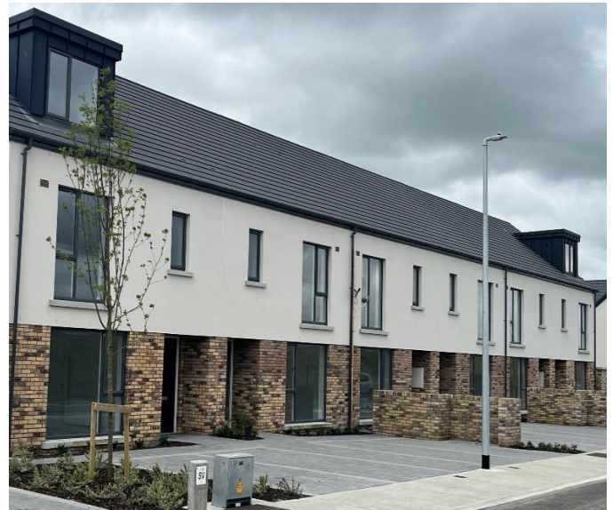
New housing units delivered in Ballymakenny Park, Drogheda, through the Part V planning process
