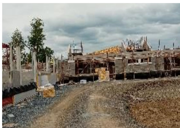
Ongoing brick and block work
