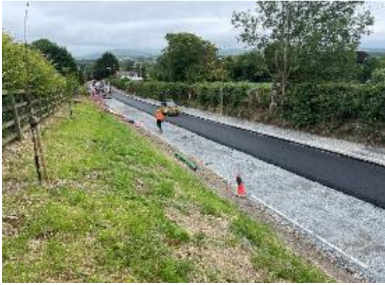
Works south of Castletown Cross
