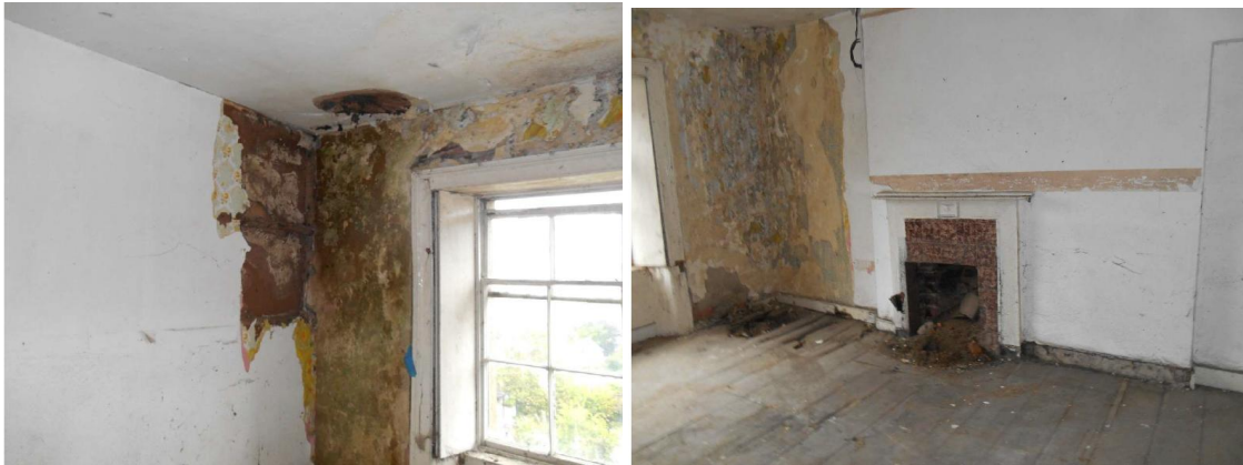
Fig.7-8: 2nd Floor front room
