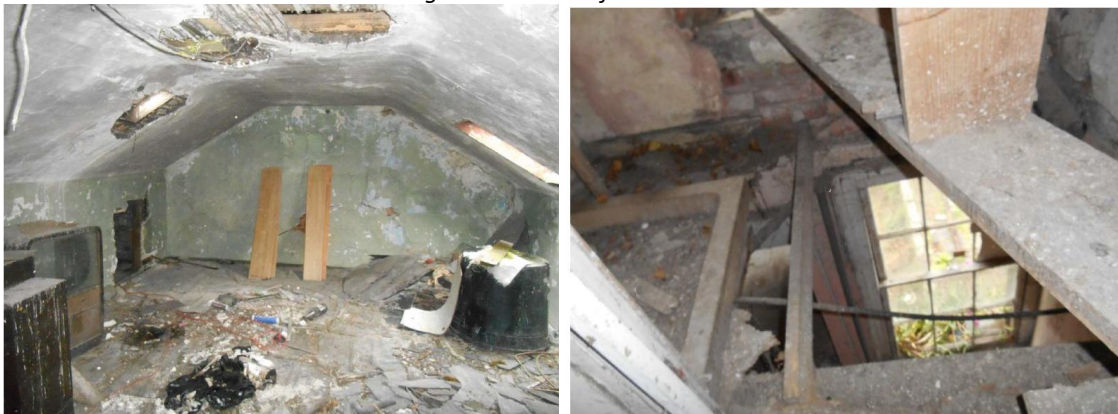
Fig.9-10: 3 rd floor / attic space / 3 rd floor bathroom
