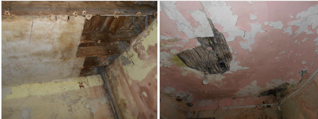
Fig 5-6: 2 nd floor ceiling
