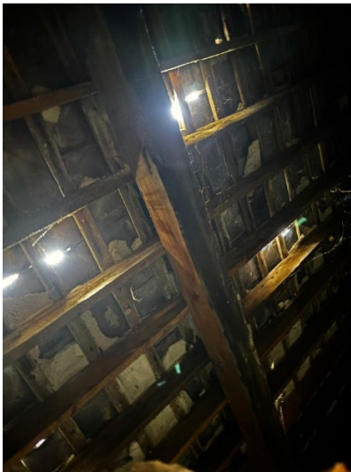
Condition of roof
