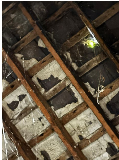
Condition of roof
