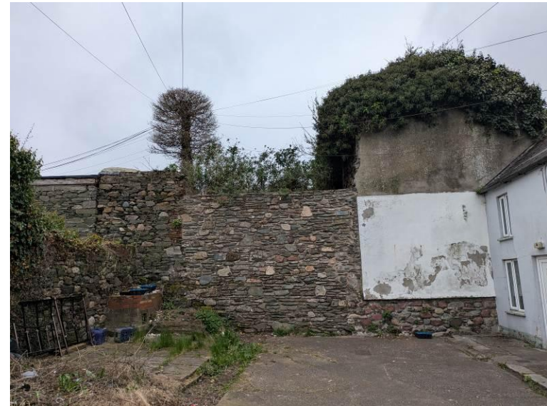
Plate 4: Masonry wall at end of Meeting House Lane, facing west
