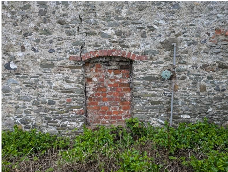
Plate 7: Blocked door opening, facing west
