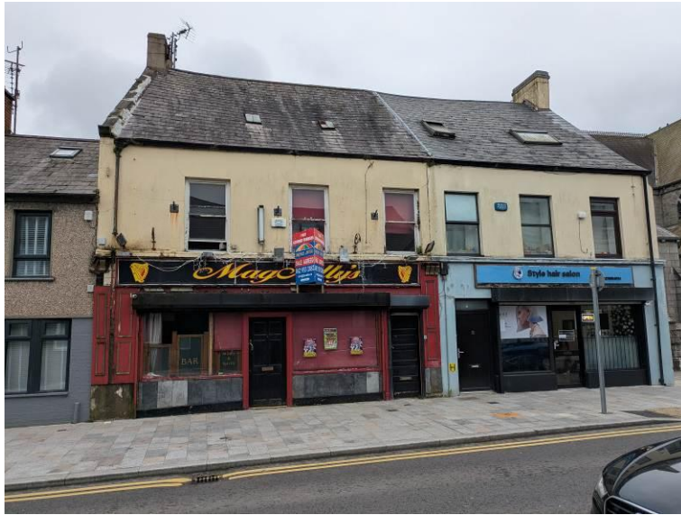
Plate 9: Nos. 2 (right) and 3 (left) Bridge Street, facing east
