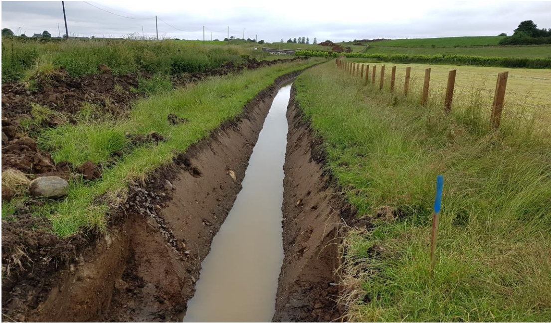
Figure 2 Example of cut-off ditch
