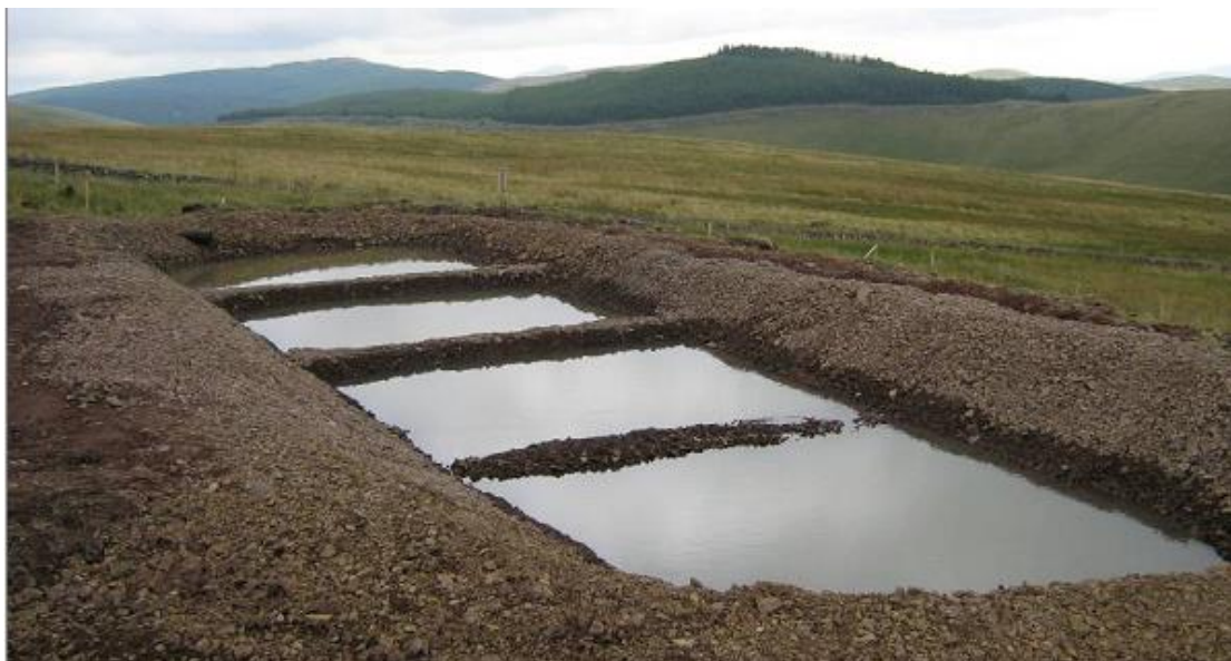
Figure 4 Typical temporary settlement pond/lagoon
