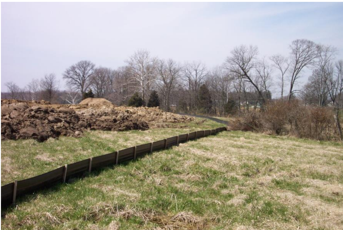
Figure 3 Typical silt fence usage
