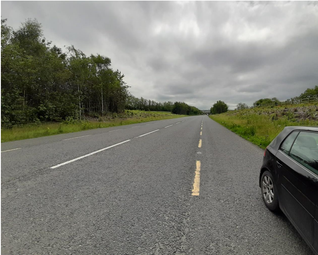
Figure 10-30 View from the N2 road at Glebe looking southeast towards Ardee.
