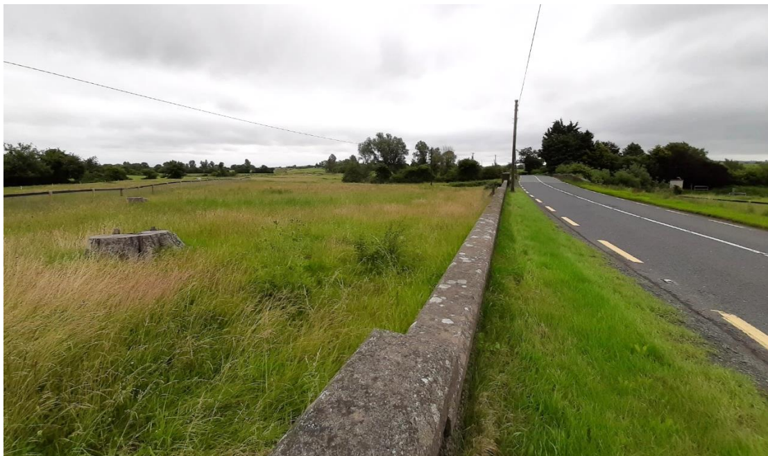
Figure 10-13 From the N52 road at Mandistown near River Dee looking northeast onto the farmland containing a section of the N52 Ardee Bypass
