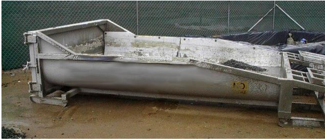
Figure 7 Typical washout facility
