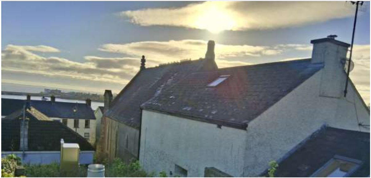
Figure 4: View of the northern side and roof of existing building
