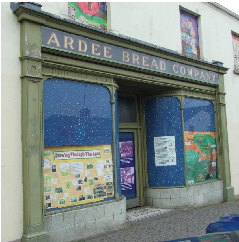
Fig. 123: Elaborate shopfront on Castle Street
