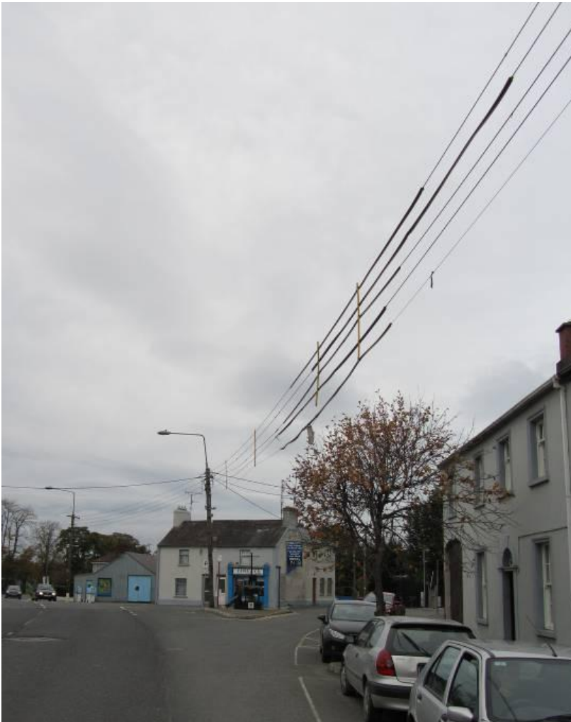
Fig. 137: Obtrusive overhead cables on Irish Street
