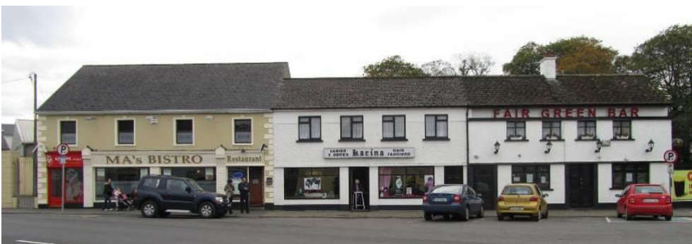
Fig. 35: Buildings south of the Fair Green intersection
