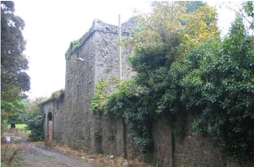
Fig. 10: 14th century tower house within farmyard of Ardee Demesne.
