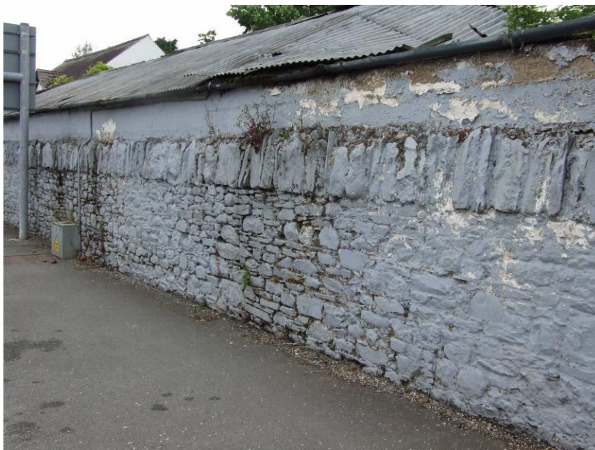
Fig. 104: Traditional stone masonry wall on Dundalk Road
