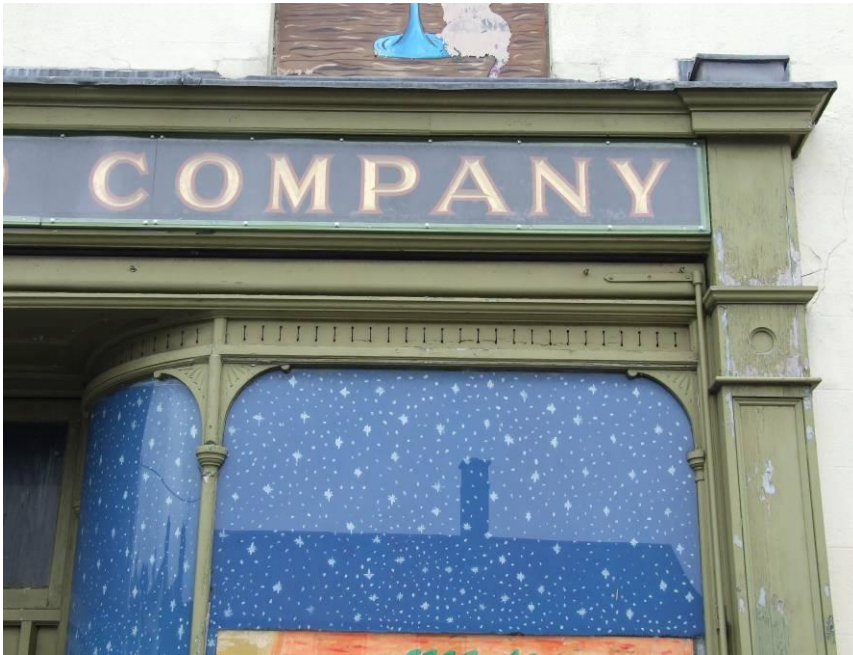
Fig. 25: Detail of shopfront on Castle Street
