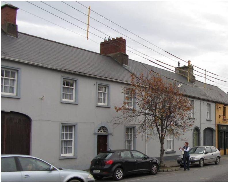
Fig. 23: Houses to east side of Irish Street
