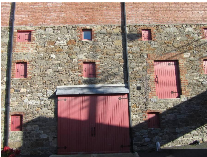
Fig. 112: Exposed brick and rubble stone wall
