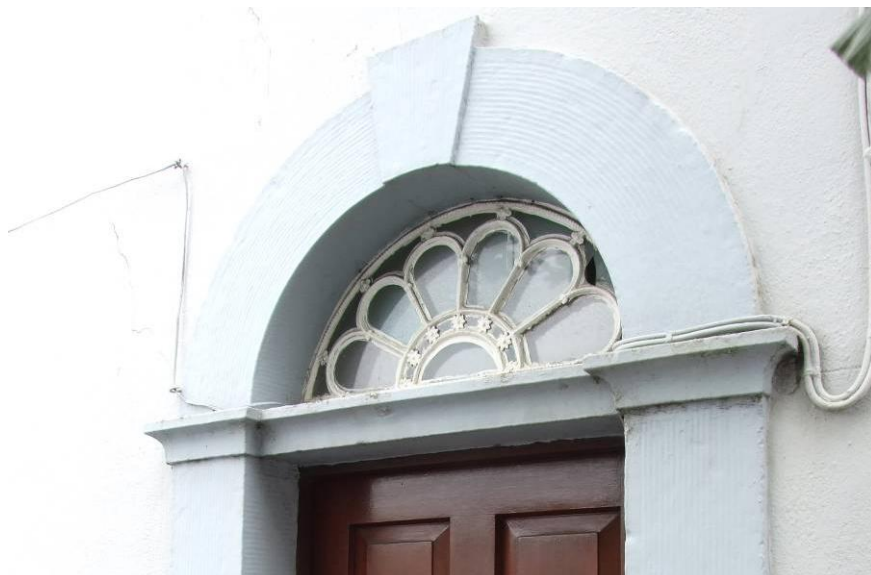
Fig. 116: Decorative fanlight on Irish Street
