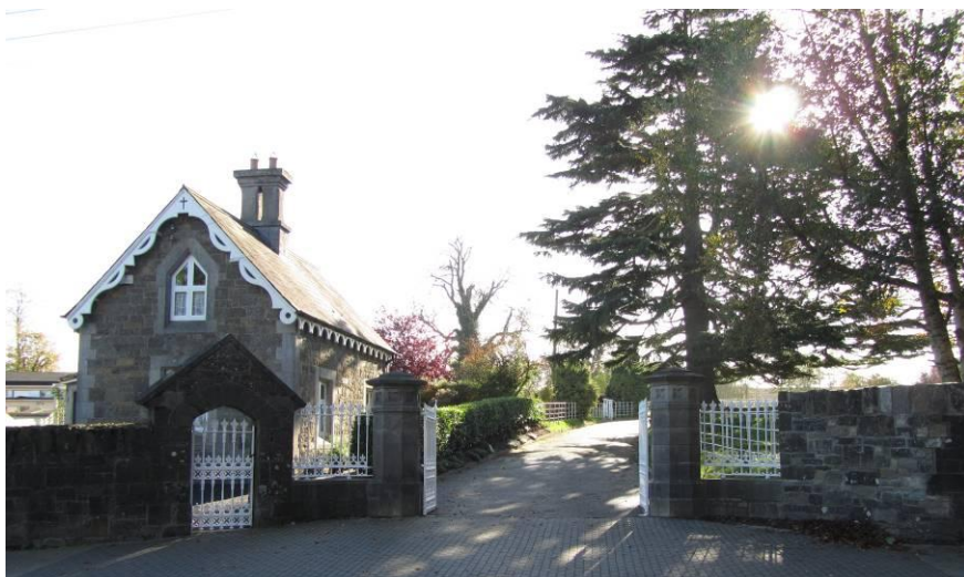
Fig. 89: Gate lodge and trees to the Convent of Mercy
