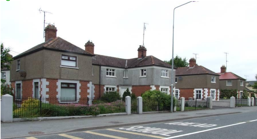
Fig. 31: Paired houses on the west side of Dundalk Road
