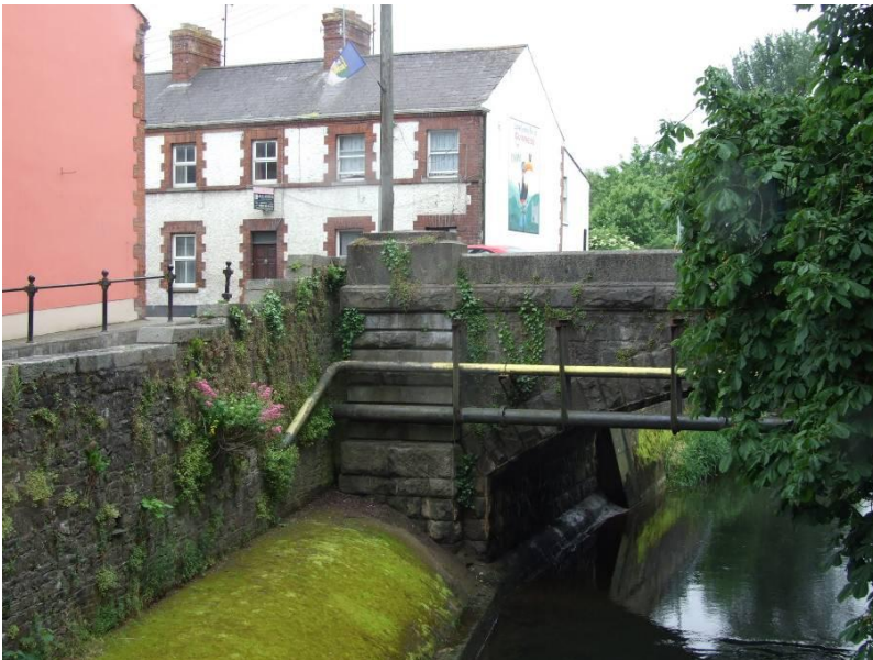
Fig. 82: Historic stone bridge in Bridge Street seen from the west
