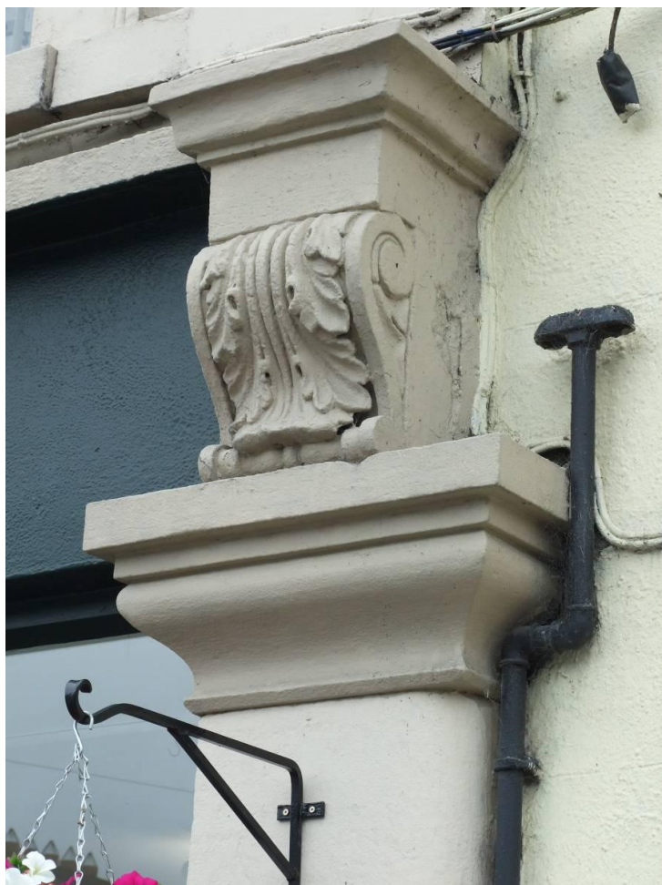
Fig. 102: Decorative stucco bracket to shopfront on Castle Street
