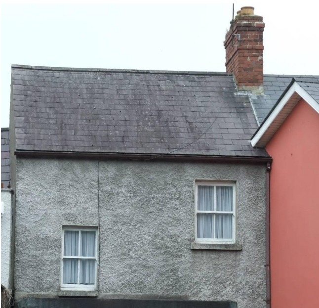
Fig. 114: Rear of house on Bridge Street seen from Moorhall
