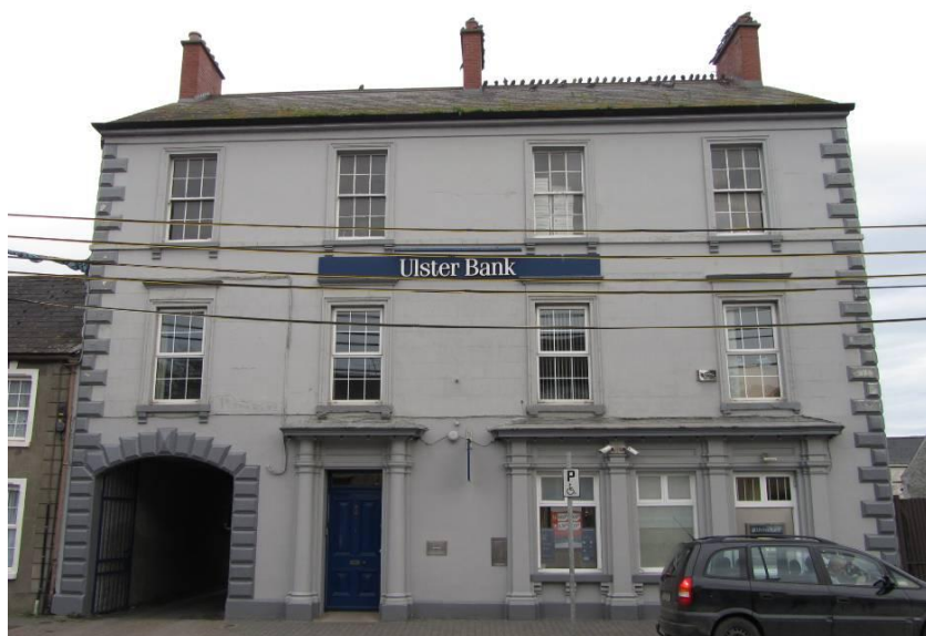
Fig. 39: Ulster Bank building
