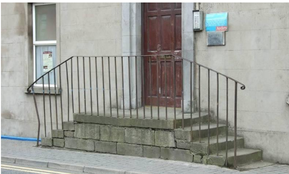
Fig. 128: Railings and steps on Bridge Street
