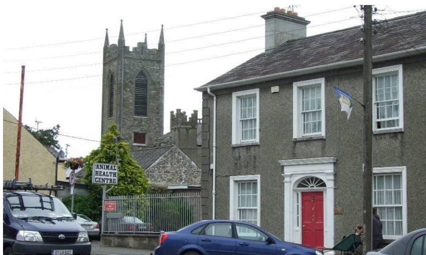
Fig. 49: St Mary's Church Tower over railings to former Methodist Church
