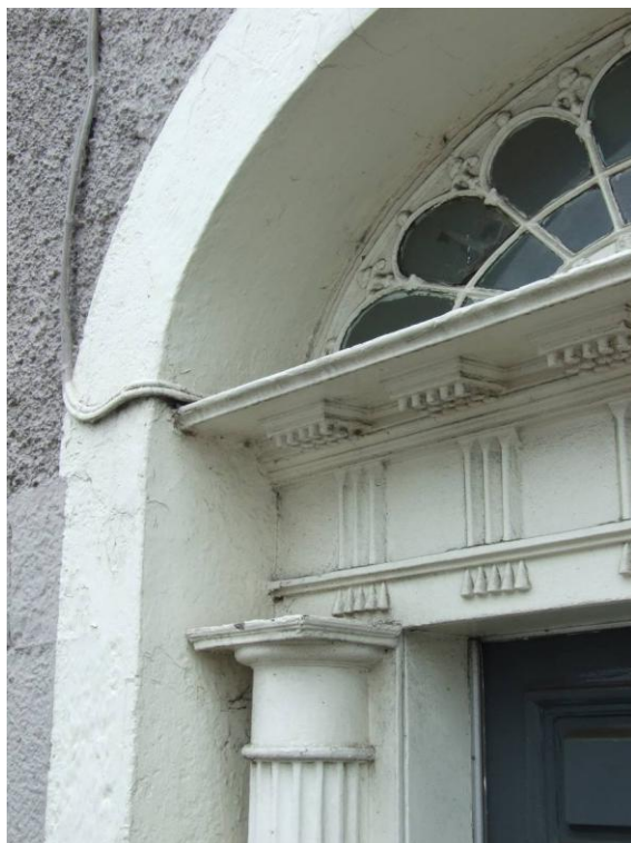
Fig. 103: Ionic detail to doorcase on William Street
