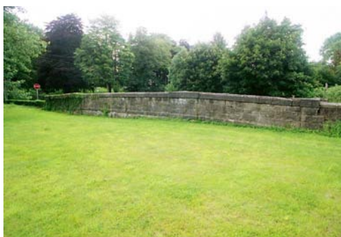
07226_01 FWH 16/08/2007 South-west elevation.
