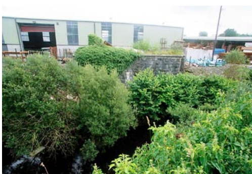
07224_01 FWH 16/08/2007 South abutment, from north.
