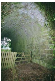
07324_01 FWH 07/10/2007 Looking south through arch from north end.
