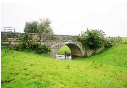
07103_01 FWH 11/08/2007 East elevation, from SE.
