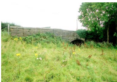
07422_01 FWH 23/08/2007 West elevation, from NW.
