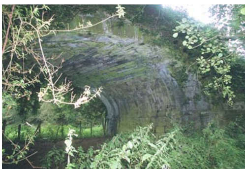
07331_01 FWH 07/10/2007 Looking through arch from west side.
