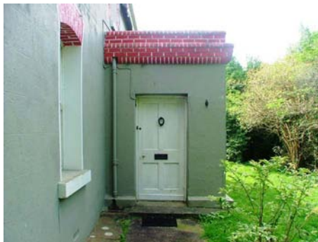
07201_54 AR&R 27/08/2007 Station house: entrance porch to front (west) elevation.
