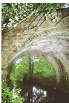
07109_01 FWH 11/08/2007 Downstream (east) elevation.
