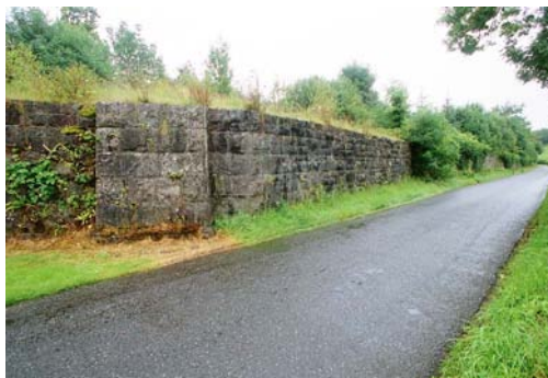
07102_01 FWH 11/08/2007 Abutment from NE.
