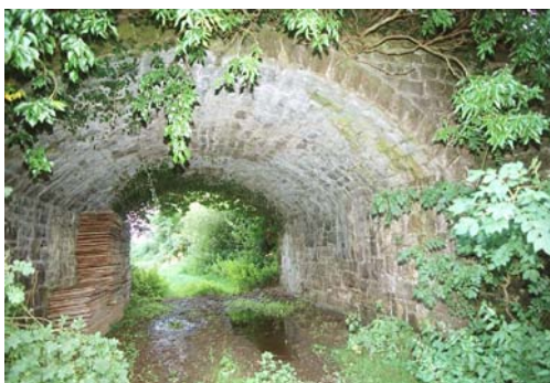
07411_01 FWH 23/08/2007 North-west elevation.
