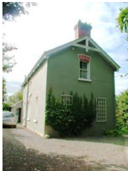
07201_52 AR&R 27/08/2007 Station house: north gable.
