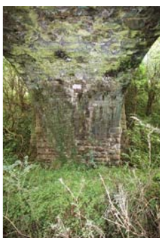
07519_01 FWH 23/08/2007 East abutment and arch soffit detail.
