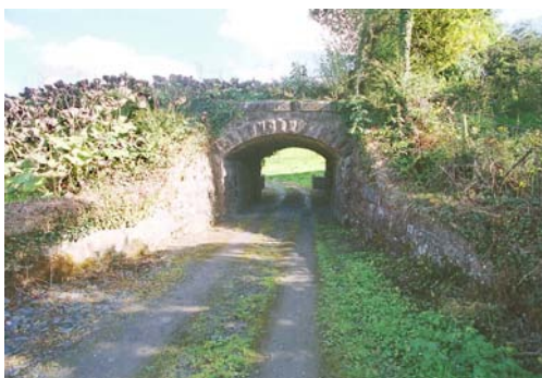
07315_01 FWH 03/09/2007 North-west elevation.
