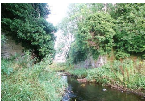
07310_01 FWH 03/09/2007 East abutment, from south.
