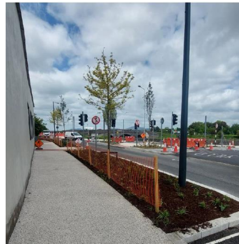
Footpath and planting along An Tain apartments.
