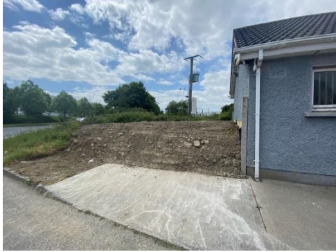
Remedial works undertaken at Woodlands Halting site to prevent future dumping
