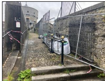
Photos: Millmount, Drogheda and locations where wall repairs are proposed
