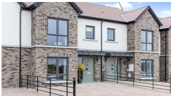
Ballymakenny Park – Affordable Housing Scheme
