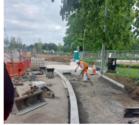
Fairgreen Road, installation of new footpath ongoing.
