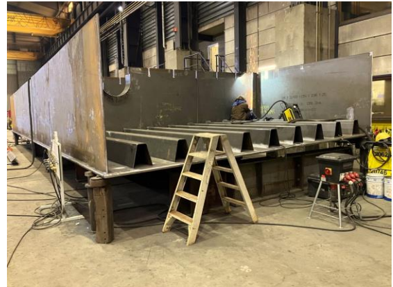
Commencement of Fabrication of Bridge Components
