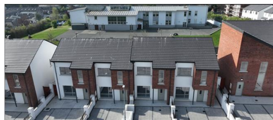
Boice Court, Mell, Drogheda – delivery of 13 new housing units
