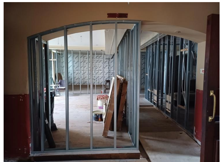
Interior works already commenced
