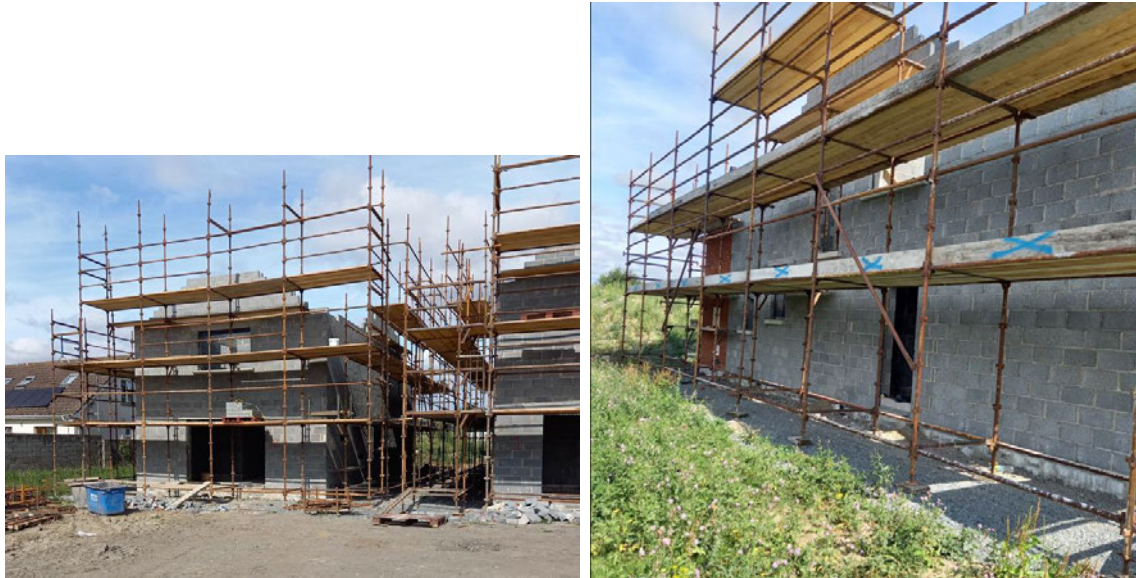
Fig.2-3: structures under construction and dwelling no. 2 southwestern gable elevation as of 14 th August 2026.
