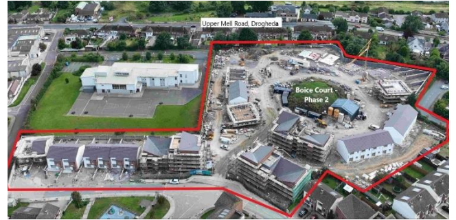
Boice Court (Phase 2), Mell, Drogheda – 72 Residential Development under construction
