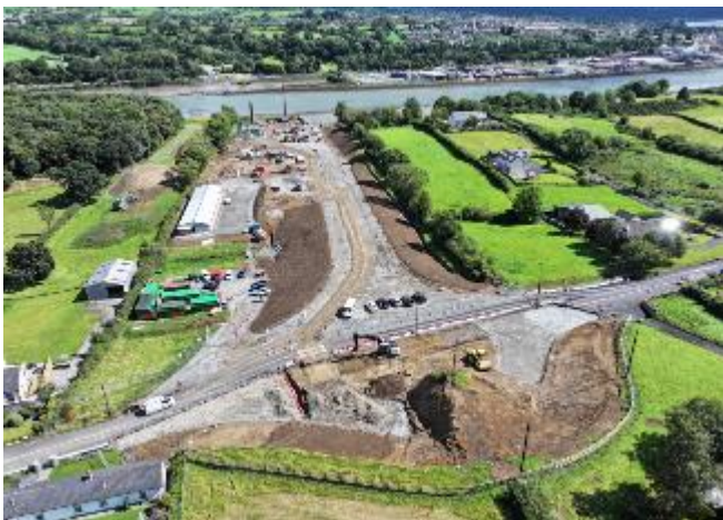
Roadworks Southern Approach.
