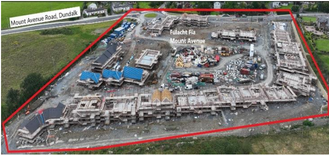
Fulacht Fia, Mount Avenue, Dundalk – 93 Residential Development under construction
