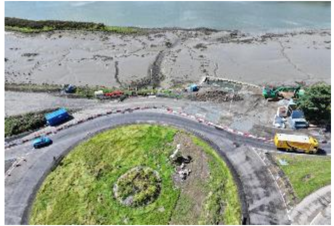
Culvert Works Northern Approach.
