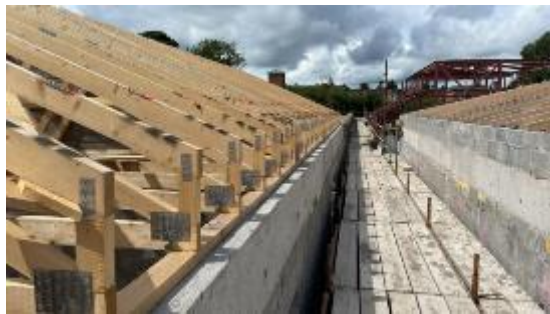
Roof Trusses installation
