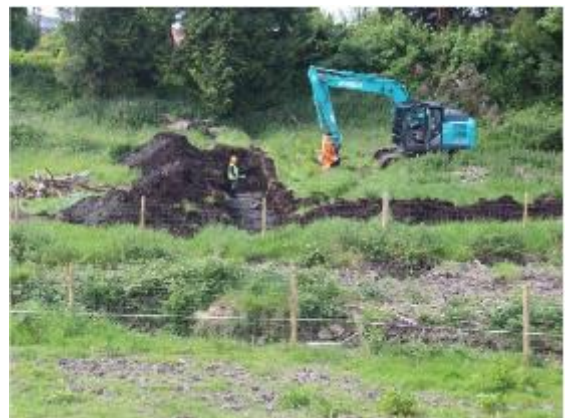
Archaeology Trenching Monitoring
