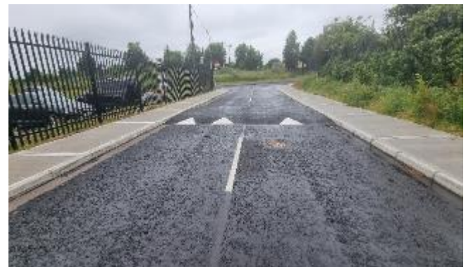
Section of New Road
