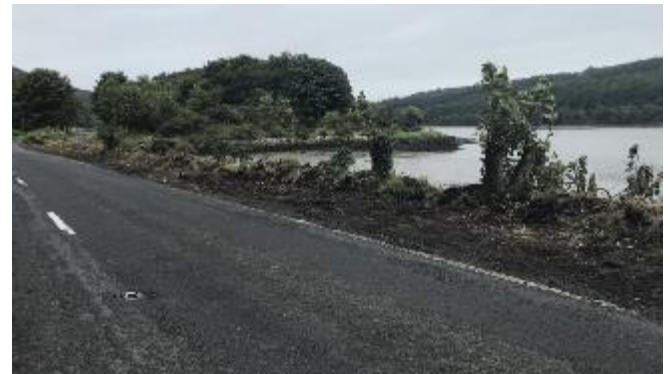
Site clearance for piling
