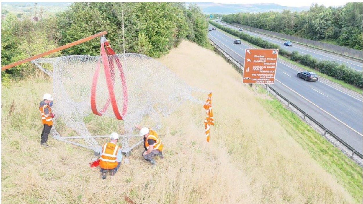
The Cooley Bull being restored to the M1 By-Pass
