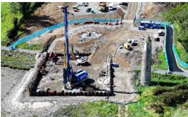
Piling Works Southern Abutment
