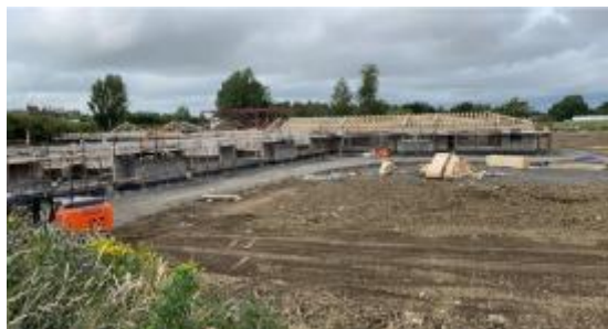
Overall site Progress
