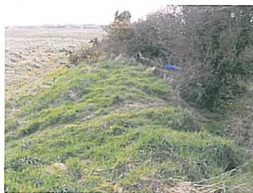
Photo 24 – chainage 653 Pedestrian path crossing the embankment
