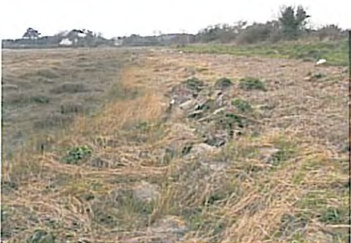
Photo 51 – chainage 1875 Larger berm in front with rock toe
