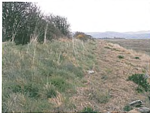
Photo 55 Front face of the embankment
