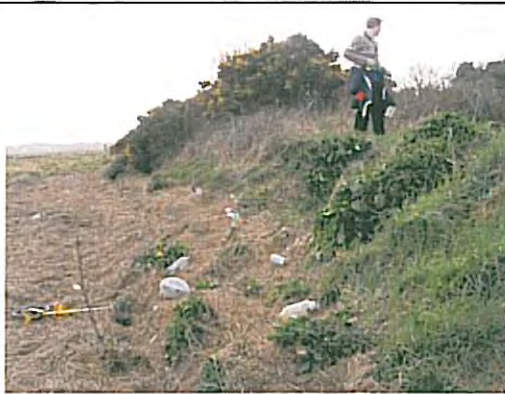
Photo 5 Front face of the embankment
