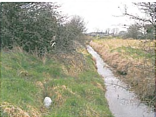
Photo 79 – chainage 1975 Typical section drainage ditch
