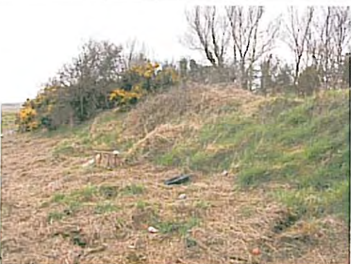
Photo 13 – chainage 408 Vulnerable spot
