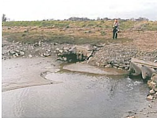
Photo 32 – chainage 1275 Front of embankment at outfalls
