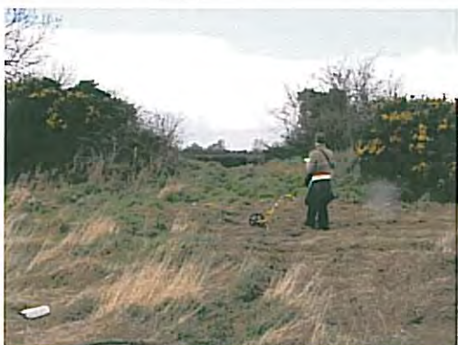
Photo 14 – chainage 572 Low spot on the embankment
