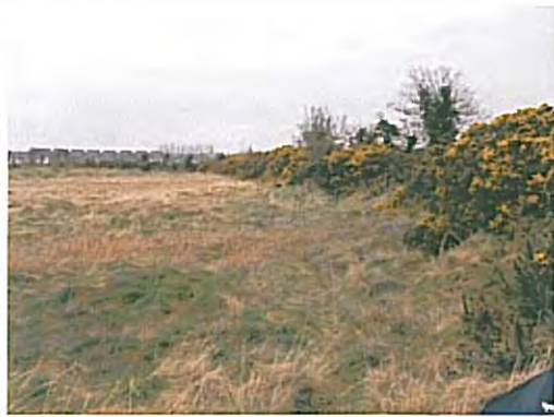
Photo 59 Front face of the embankment
