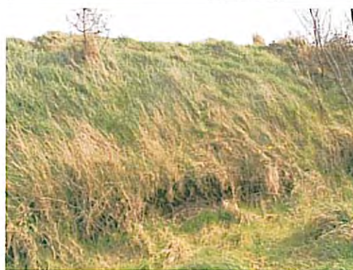
Photo 38 Vertical toe back face of the embankment
