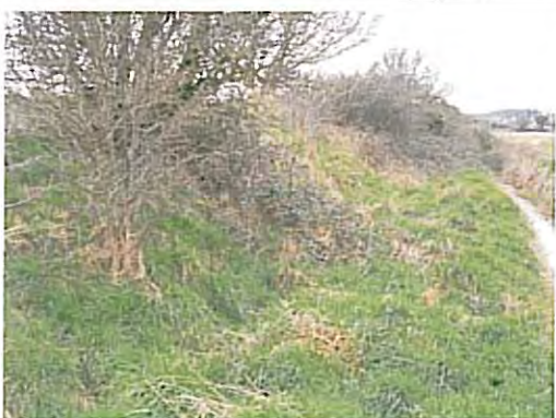
Photo 47 Back face of the embankment
