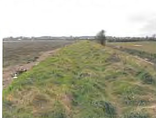
Chainage 1300 looking south
