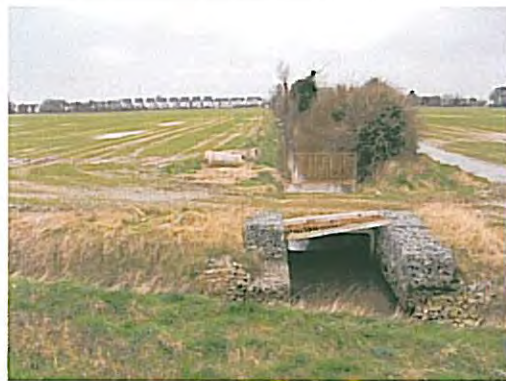
Photo 78 – chainage 1680 Perpendicular ditch joining and bridge
