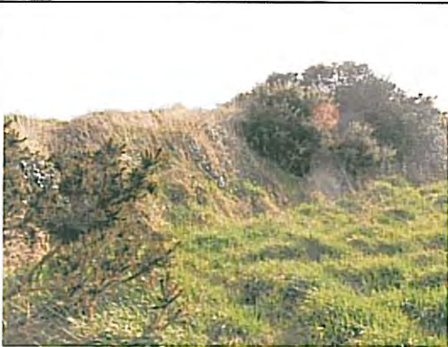
Photo 17 Back face of the embankment
