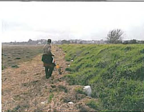
Photo 35 Front face of the embankment
