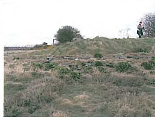
Photo 56 End of the embankment and toe
