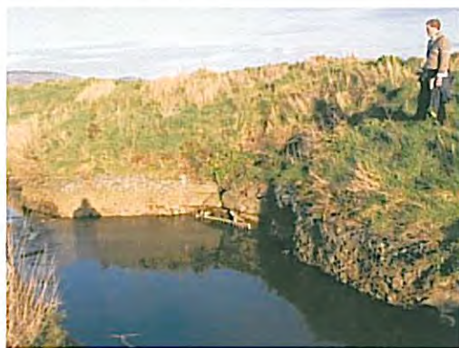
Photo 74 – chainage 1275 inlet structure outfalls
