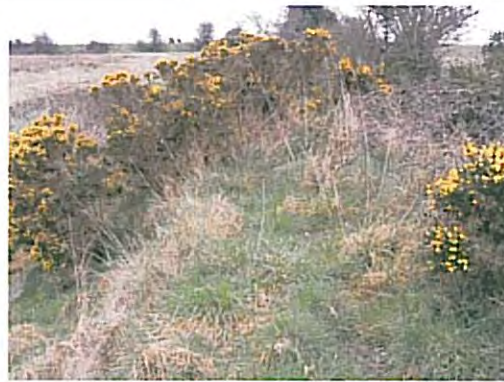
Photo 60 Crest of the embankment
