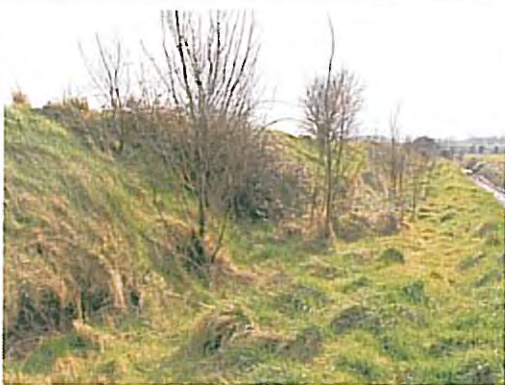
Photo 37 Back face of the embankment
