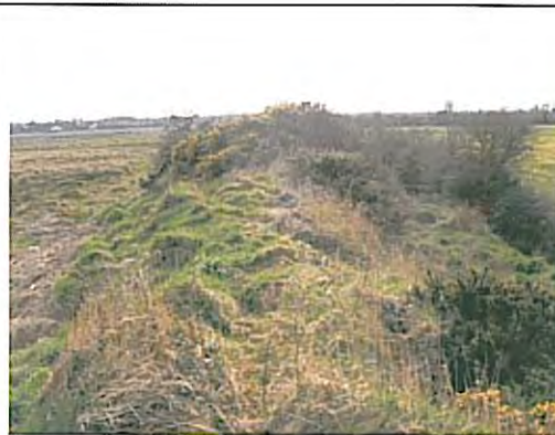
Photo 16 Crest of the embankment
