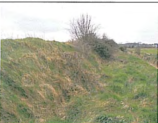
Photo 43 – chainage 1680 Start of vegetation back face
