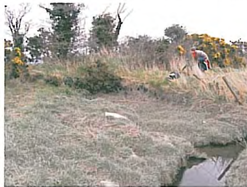
Photo 64 – chainage 2346 Trench ending against embankment
