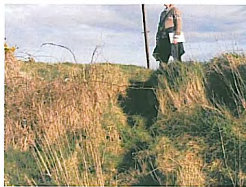
Photo 30 – chainage 1093 Pedestrian path crossing the embankment
