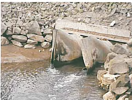
New outfall pipes
