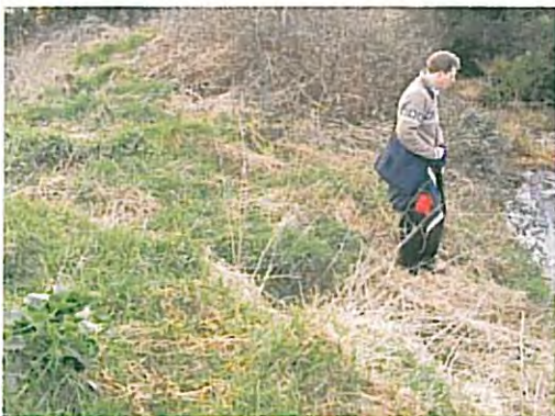
Photo 7 Back face of the embankment
