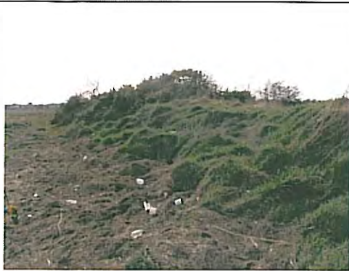
Photo 15 Front face of the embankment
