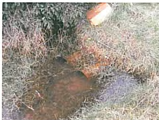
Pipes running under blockage
