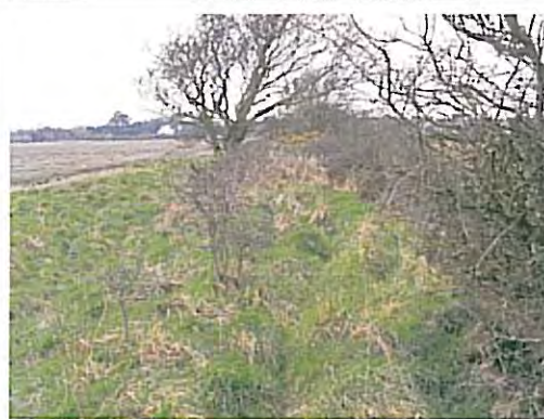
Photo 46 Crest of the embankment
