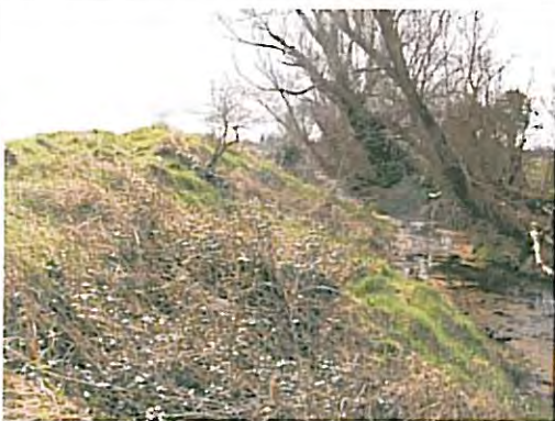
Photo 3 Back face of the embankment
