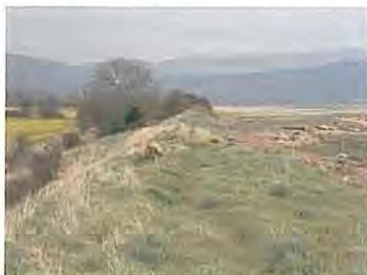
Chainage 1300 looking north
