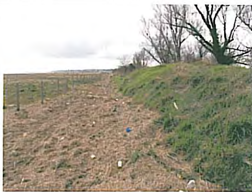
Photo 1 Front face of the embankment
