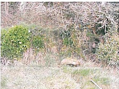
Photo 67 – chainage 2475 Masonry end of embankment
