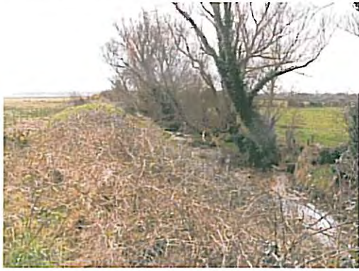
Photo 69 – chainage 0077 Ditch around start inspection
