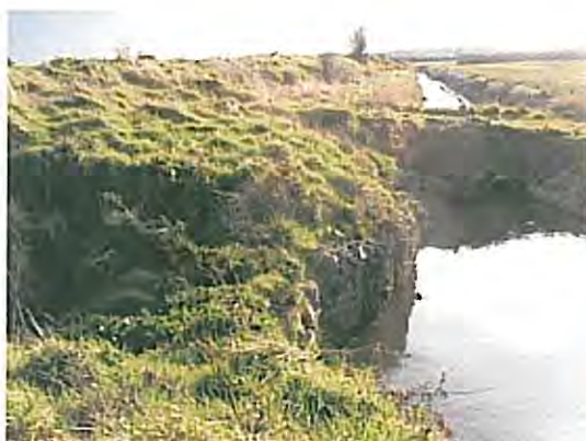
Land bridge with culvert
