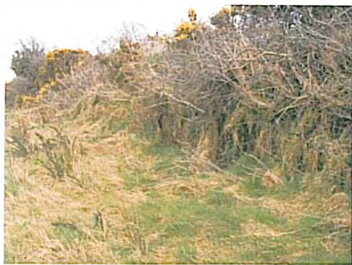
Photo 23 – chainage 835 Steep toe back face
