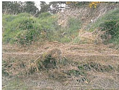
Photo 10 – chainage 47 Steep toe front face of the embankment
