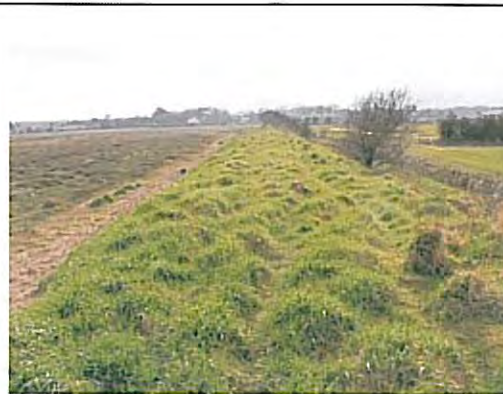
Photo 36 Crest of the embankment
