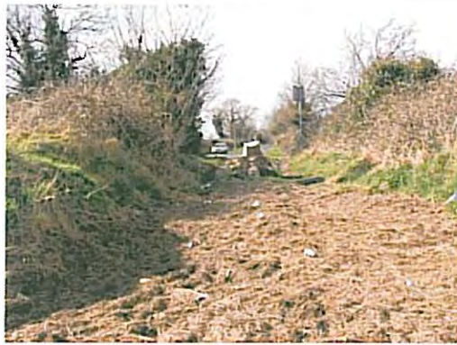
Photo 9 – chainage 0 Access gap at the bottom of Shore Road
