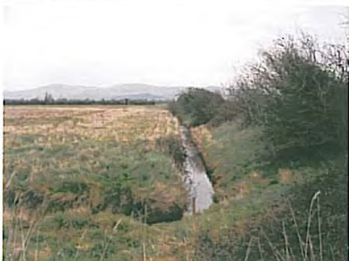
Photo 57 Back face of the embankment
