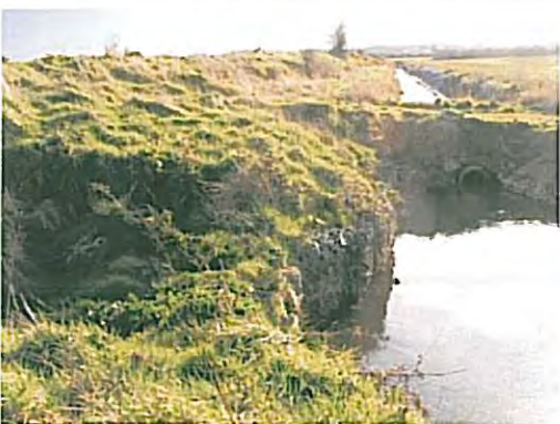
Photo 73 – chainage 1275 Ditch at outfalls
