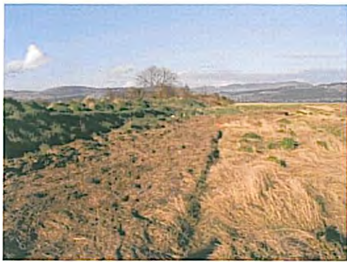
Photo 19 Front face of the embankment
