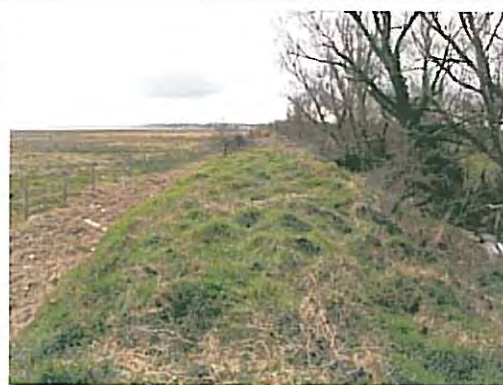
Photo 2 Crest of the embankment looking South
