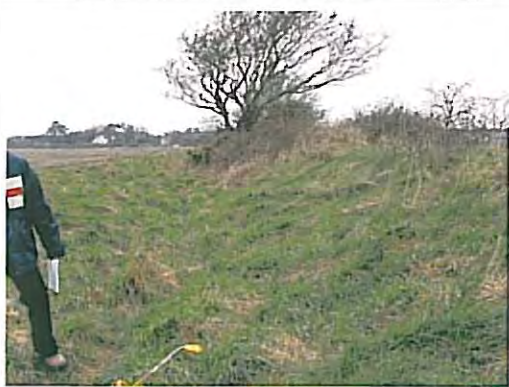
Photo 45 Front face of the embankment
