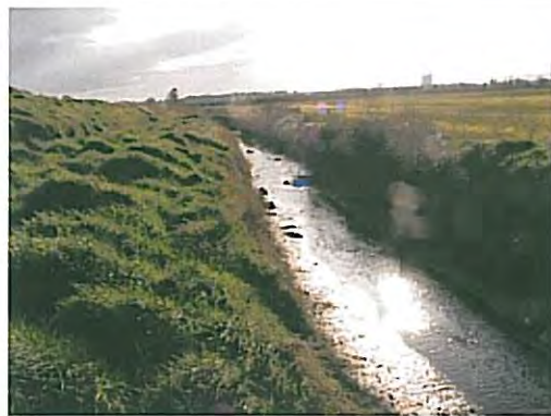
Photo 72 – chainage 1211 Typical section of ditch
