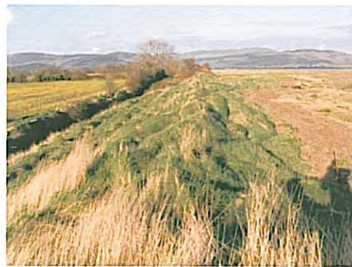
Photo 20 Crest of the embankment
