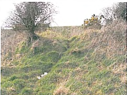
Photo 25 – chainage 785 Path crossing over the embankment
