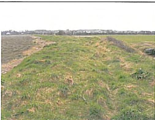
Photo 41 – chainage 1450 Widest part of the embankment
