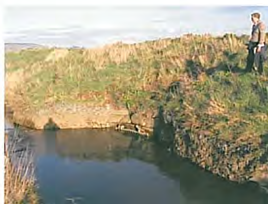
Outlet drainage ditch
