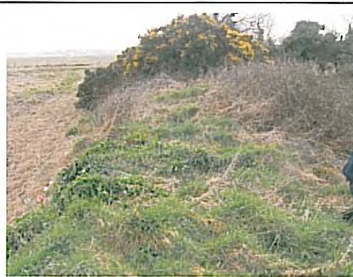
Photo 6 Crest of the embankment
