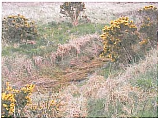
Photo 61 Back face of the embankment
