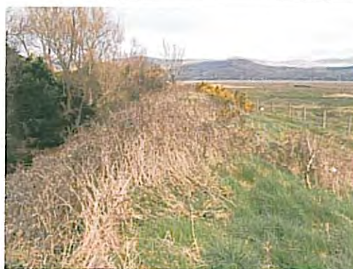
Photo 4 Crest of the embankment looking North
