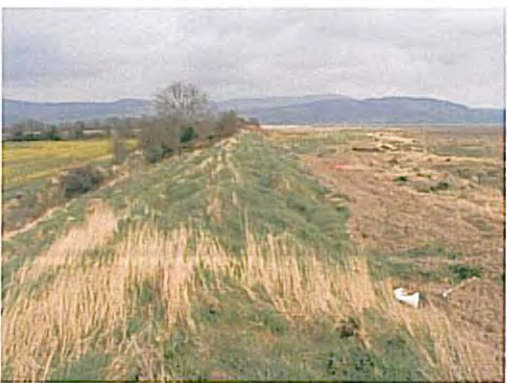
Photo 33 – chainage 0932 Crest of embankment at outfalls
