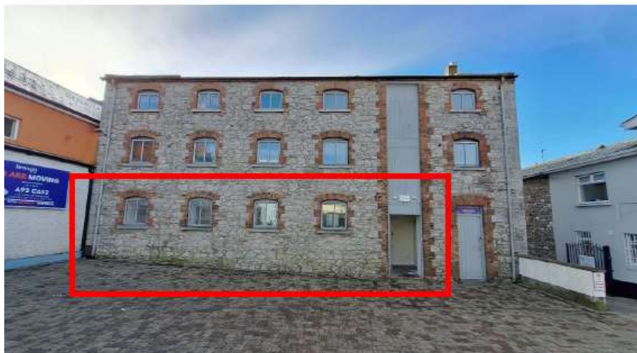
Figure 2: Shows the front elevation of the existing building, with the area that relates to this application outlined in red (ground floor and lower ground floor).
