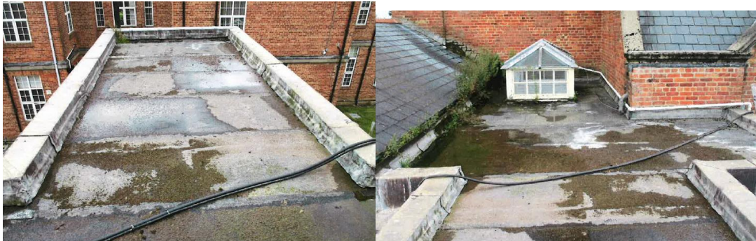
Current condition of roof 2.
