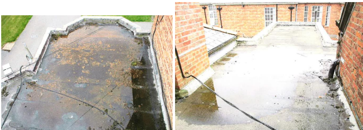
General view of roof no. 1 and no. 3 above
