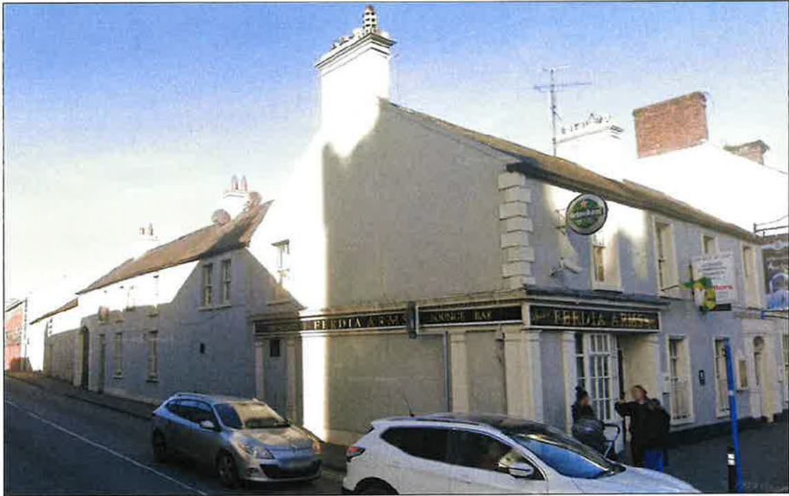
Figure 2.0 Streetview image of the subject site as viewed from the southeast.
