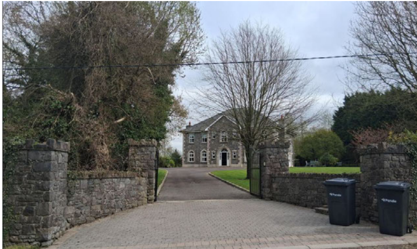
Fig.1: Existing Dwelling (photo taken 08/04/2026.)
