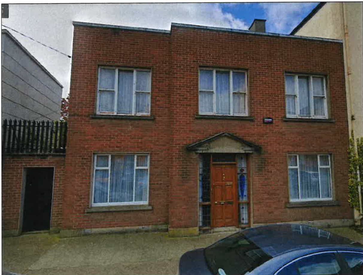
Figure 3.0 Image of the existing building on Fair Street.
