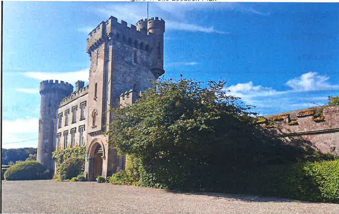
Existing Castle (taken 16/07/2025.)
