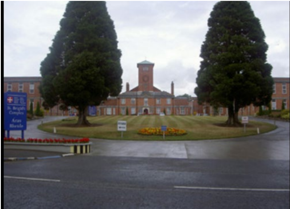
Roadside elevation of the Hospital
