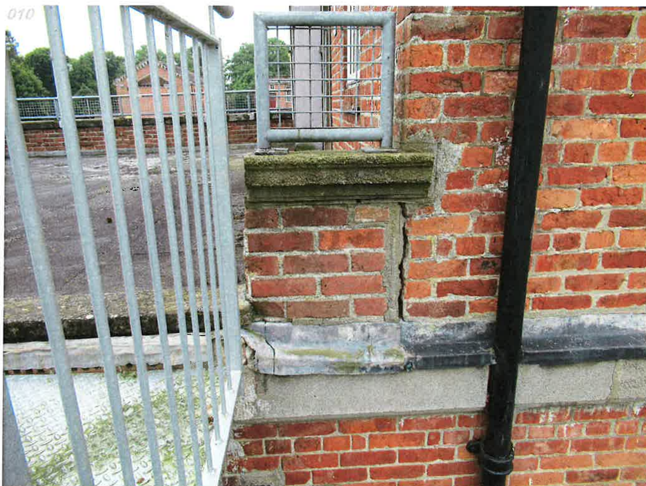
Structural cracking along front of building
