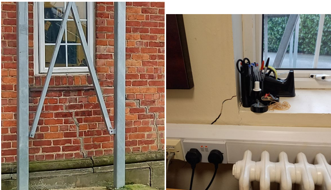
Above: photo of exterior wall and the interior of same wall
