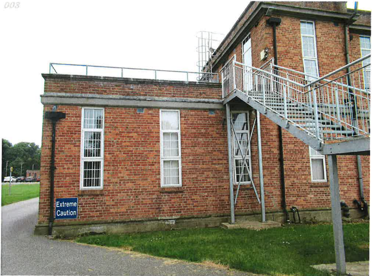
Rear elevation view of building wing
