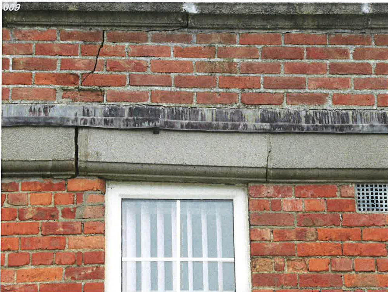
Structural cracking along front of building
