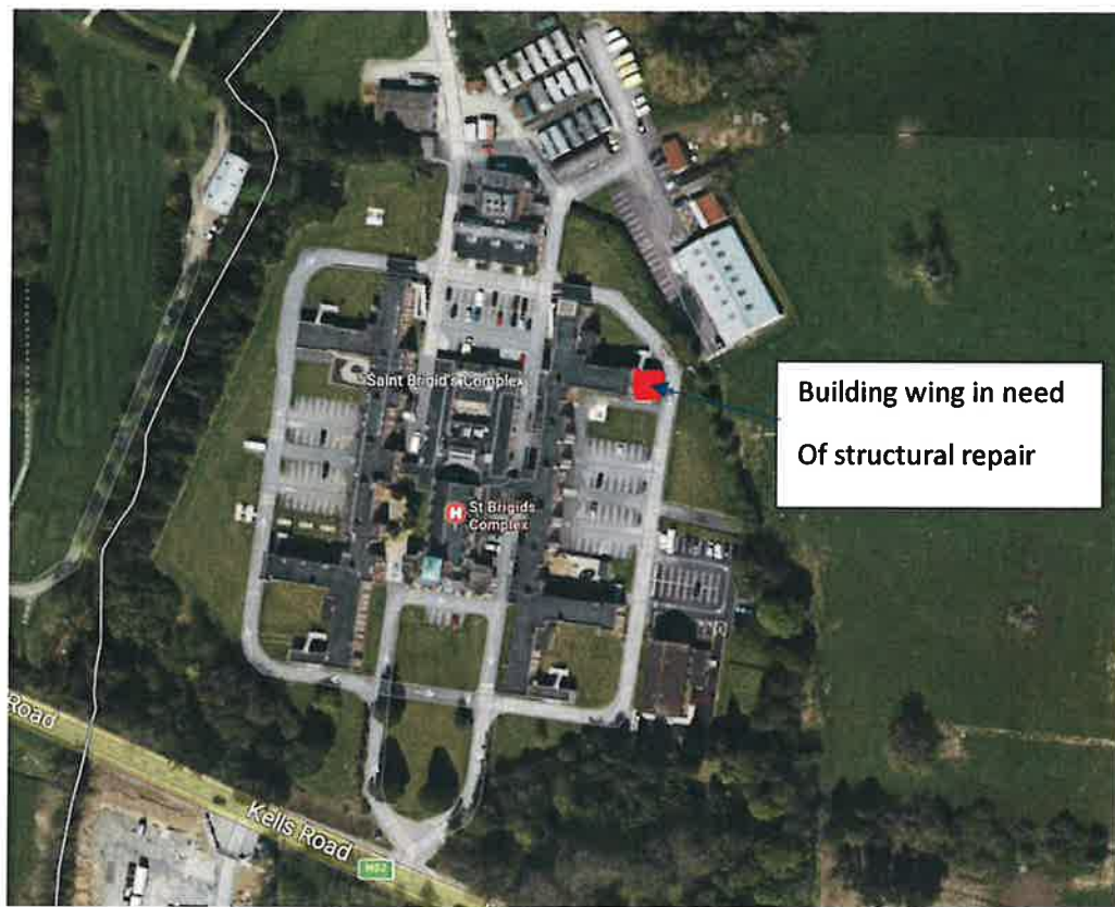
Aerial view of St. Brigid's Campus, Ardee, Co. Louth.
