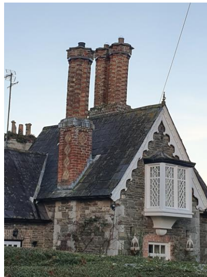
chimneys & fascia at adjacent dwelling
