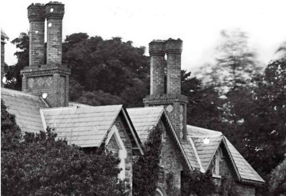
Original chimneys and fascia detailing - Lawrence Collection, National Library of Ireland
