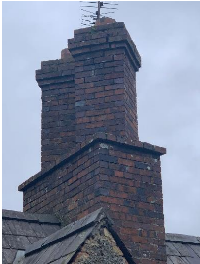
existing chimneys, not original
