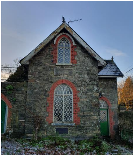
Timber fascia with lath & plaster soffit
