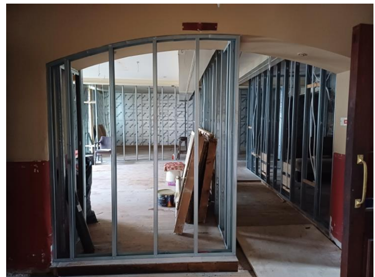
Interior works already commenced
