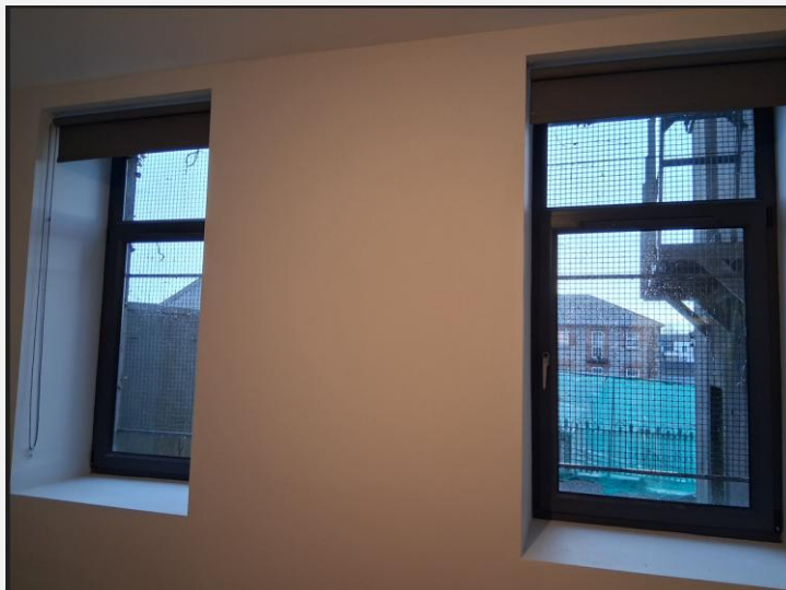
Interior as existing
