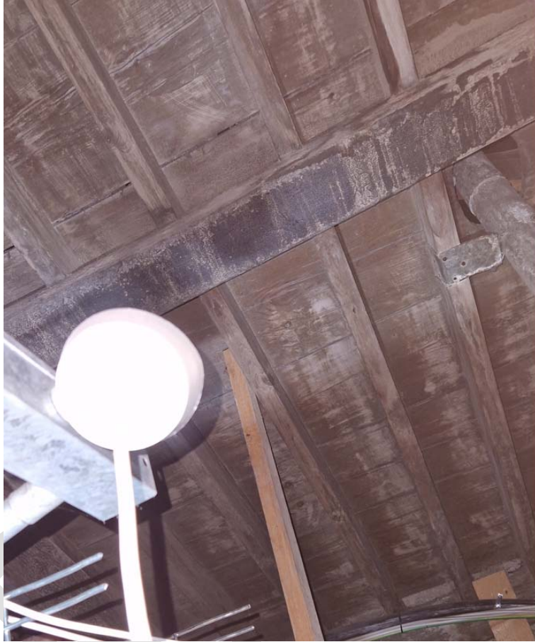
Photograph 27 – Timber sarking
