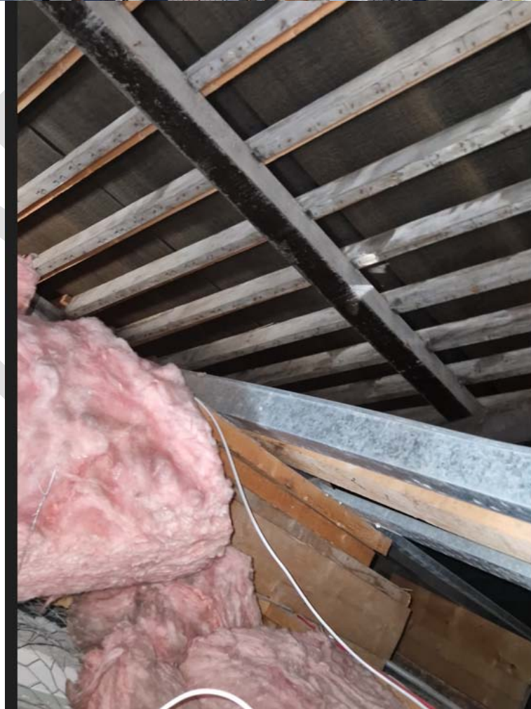
Photograph 19 – Insulation to attic
