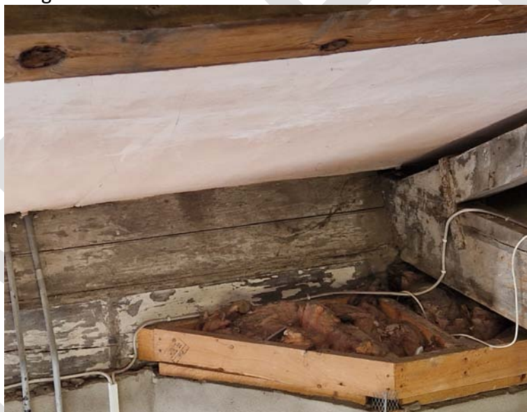
Photograph 4 – Metal and timber treatment to be provided
