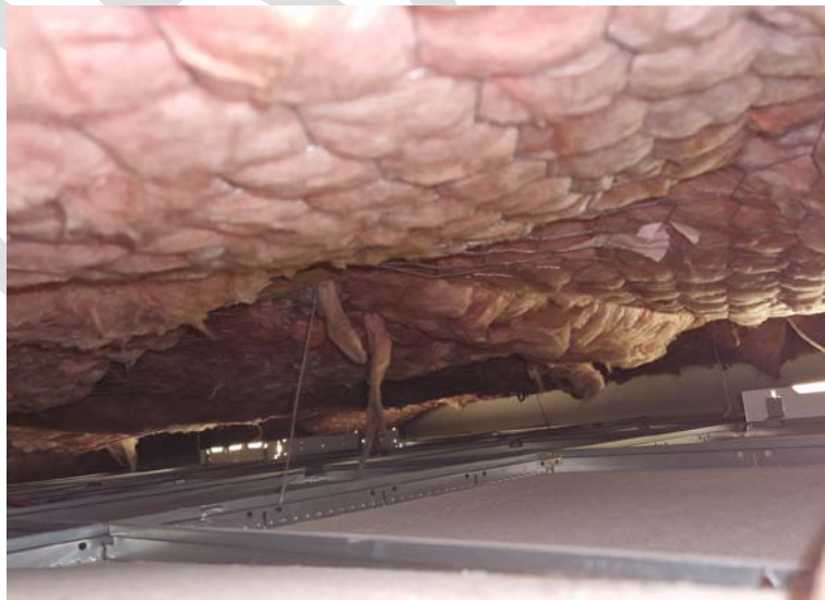
Photograph 17 – Insulation and chicken wire
