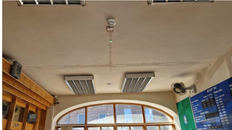
Photograph 25 – cracked ceiling
