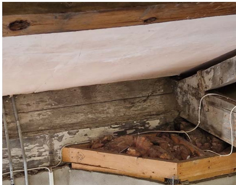
Photograph 3 – Metal and timber treatment to be provided
