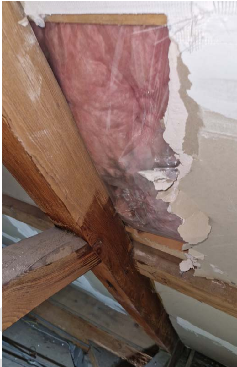
Photograph 12 – Insulation to underside of roof
