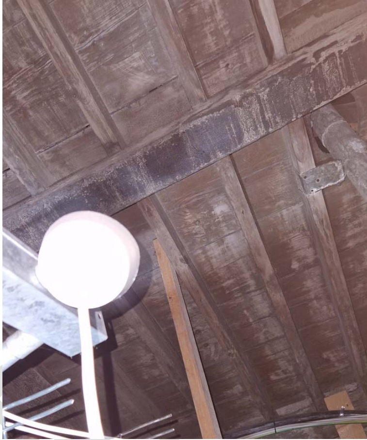
Photograph 27 – Timber sarking
