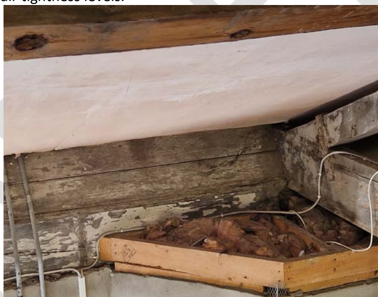
Photograph 4 – Metal and timber treatment to be provided
