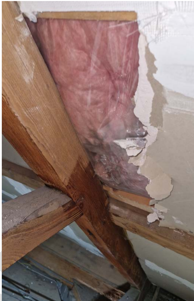
Photograph 12 – Insulation to underside of roof
