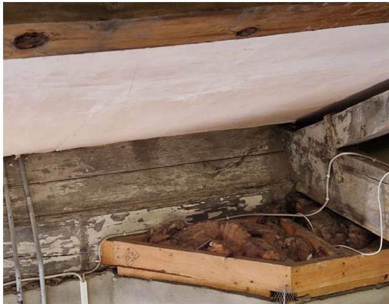
Photograph 3 – Metal and timber treatment to be provided
