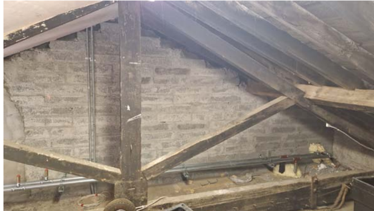
Photograph 1 – King Post and party wall
