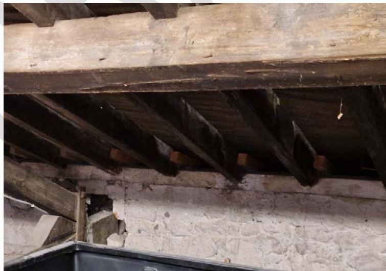
Photograph 9 – Repairs to existing rafters
