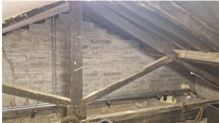
Photograph 1 – King Post and party wall
