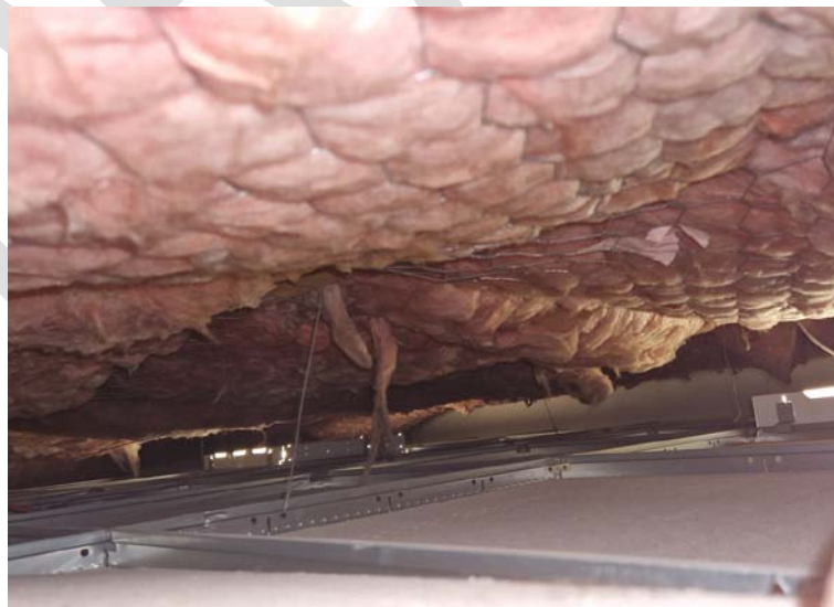
Photograph 17 – Insulation and chicken wire
