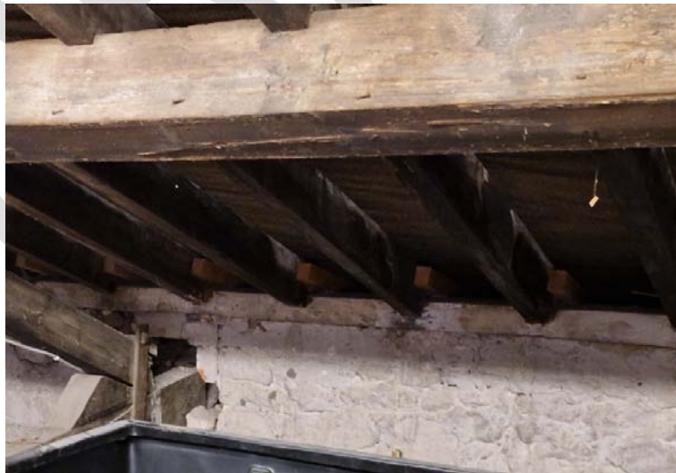
Photograph 9 – Repairs to existing rafters
