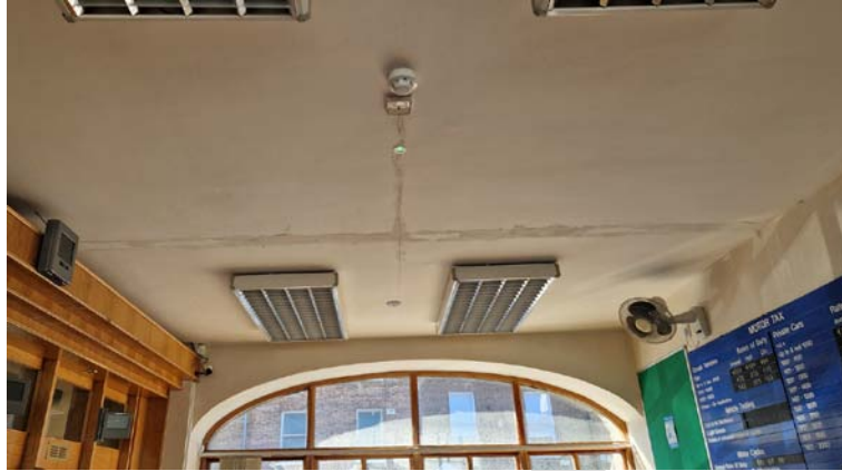
Photograph 25 – cracked ceiling
