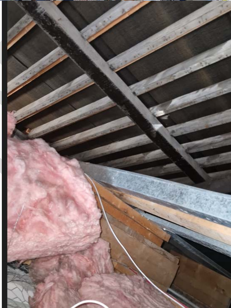
Photograph 19 – Insulation to attic
