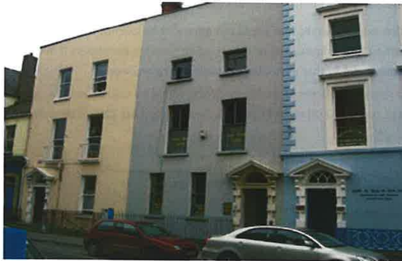
Figure 1: Front Façade – 29 St. Laurence Street, Drogheda
