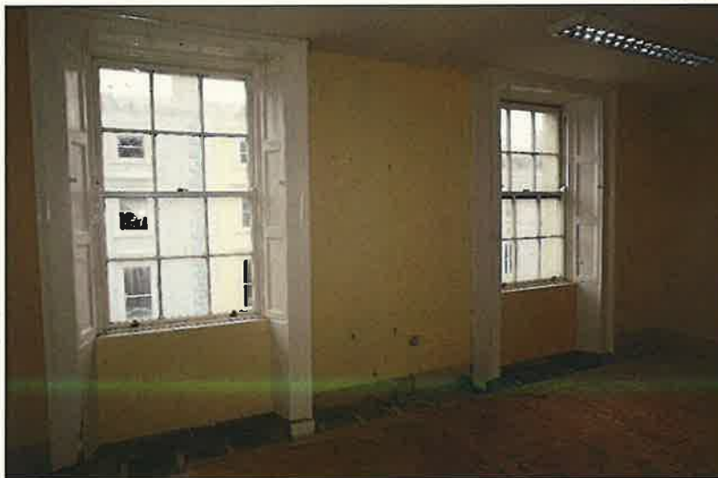
Photograph 4 -View of the Second floor front windows and historic fabric
