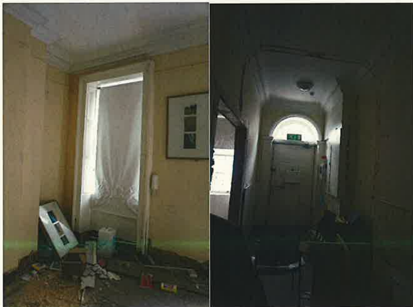
Photograph 8 - View of the ground floor front room and entrance area
