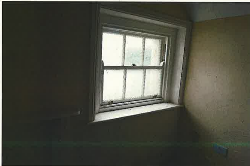
Photograph 2 - View of the existing window
