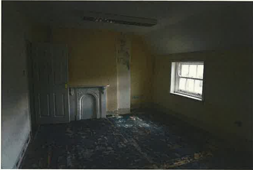
Photograph 1 – Internal View of the third floor – front room
