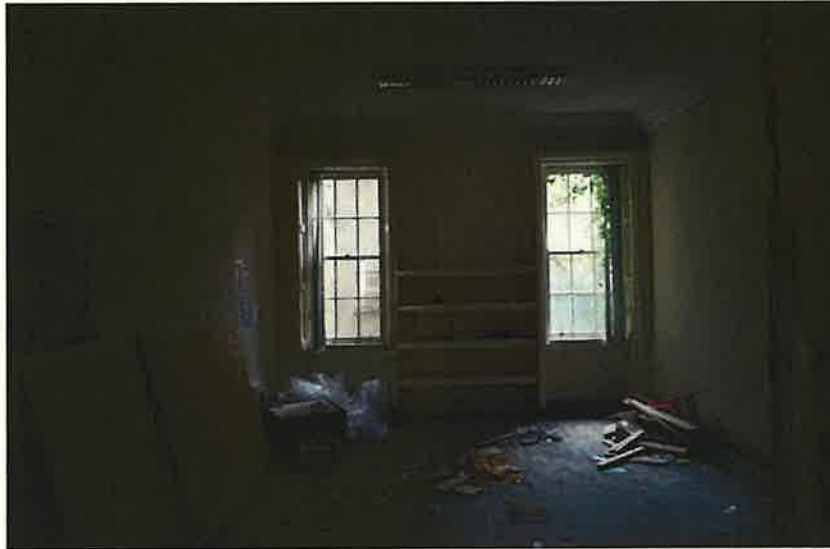
Photograph 7 - View of the ground floor fabric and existing windows
