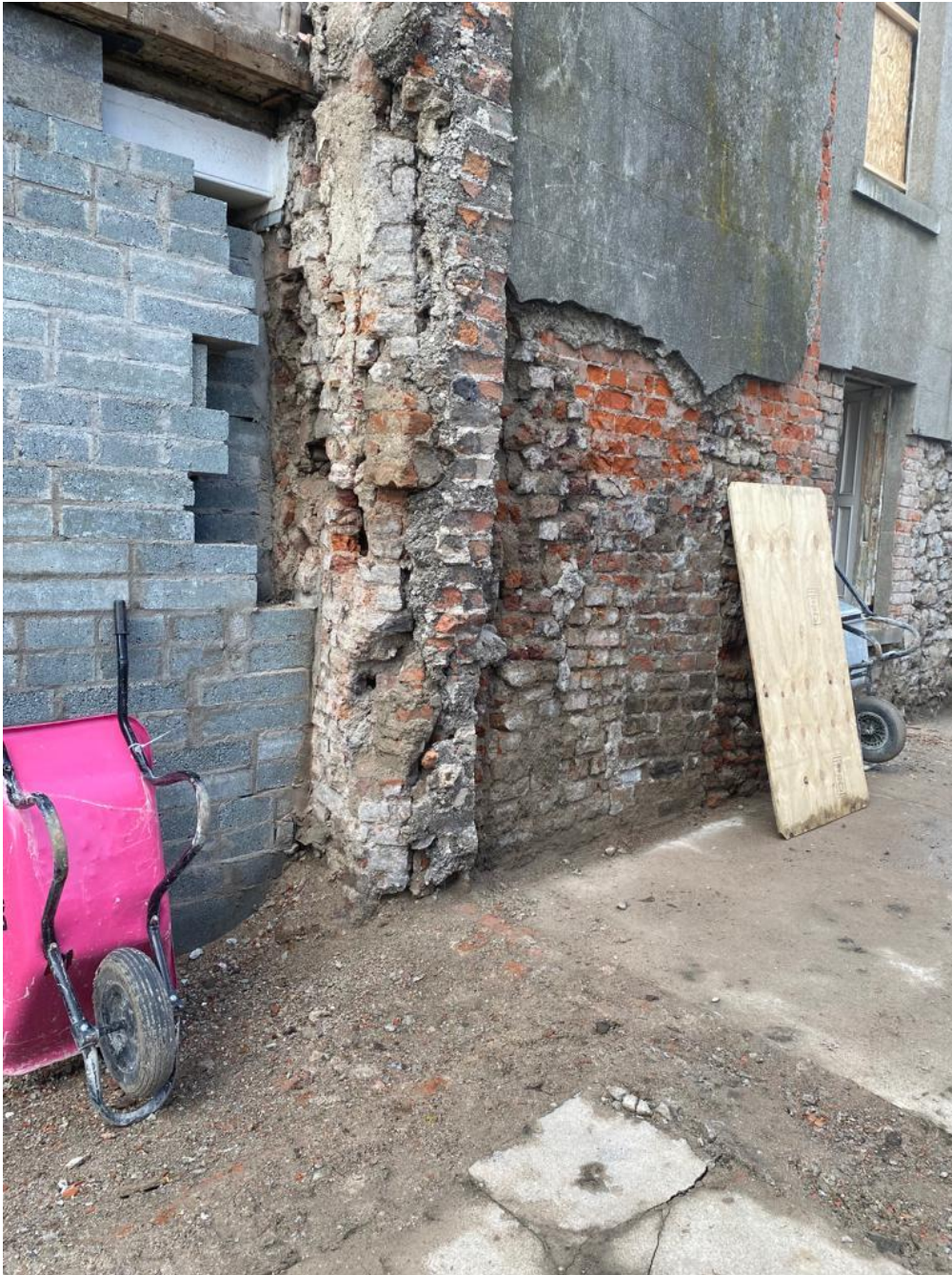
Figure 5 - View of the base of the wall(East – South)
