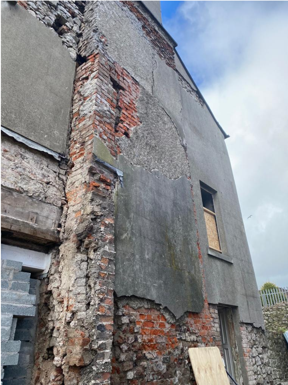
Figure 4 -View of the gable wall (East – South)
