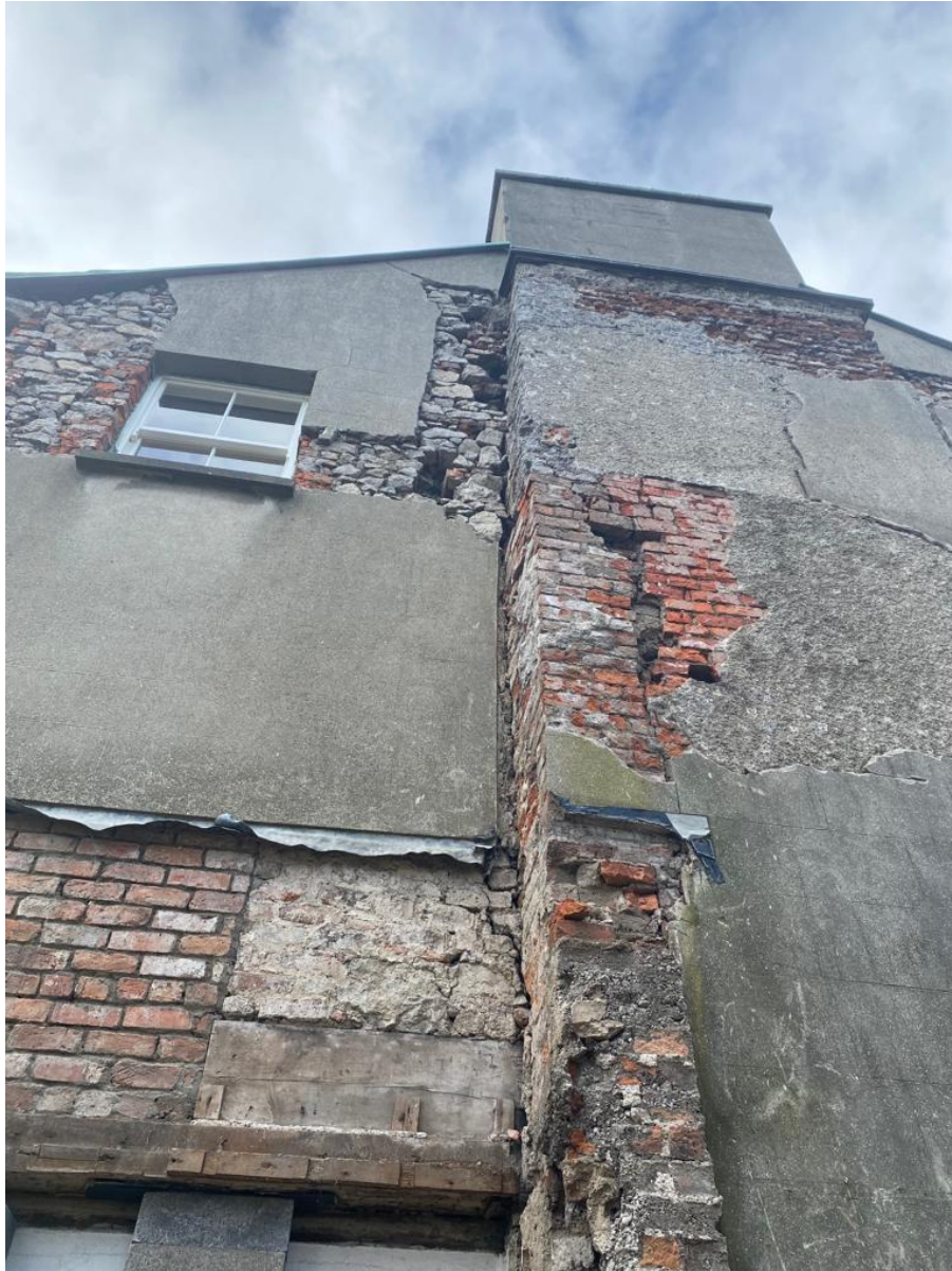
Figure 1 – View of the top of the Gable Wall (East – South)
