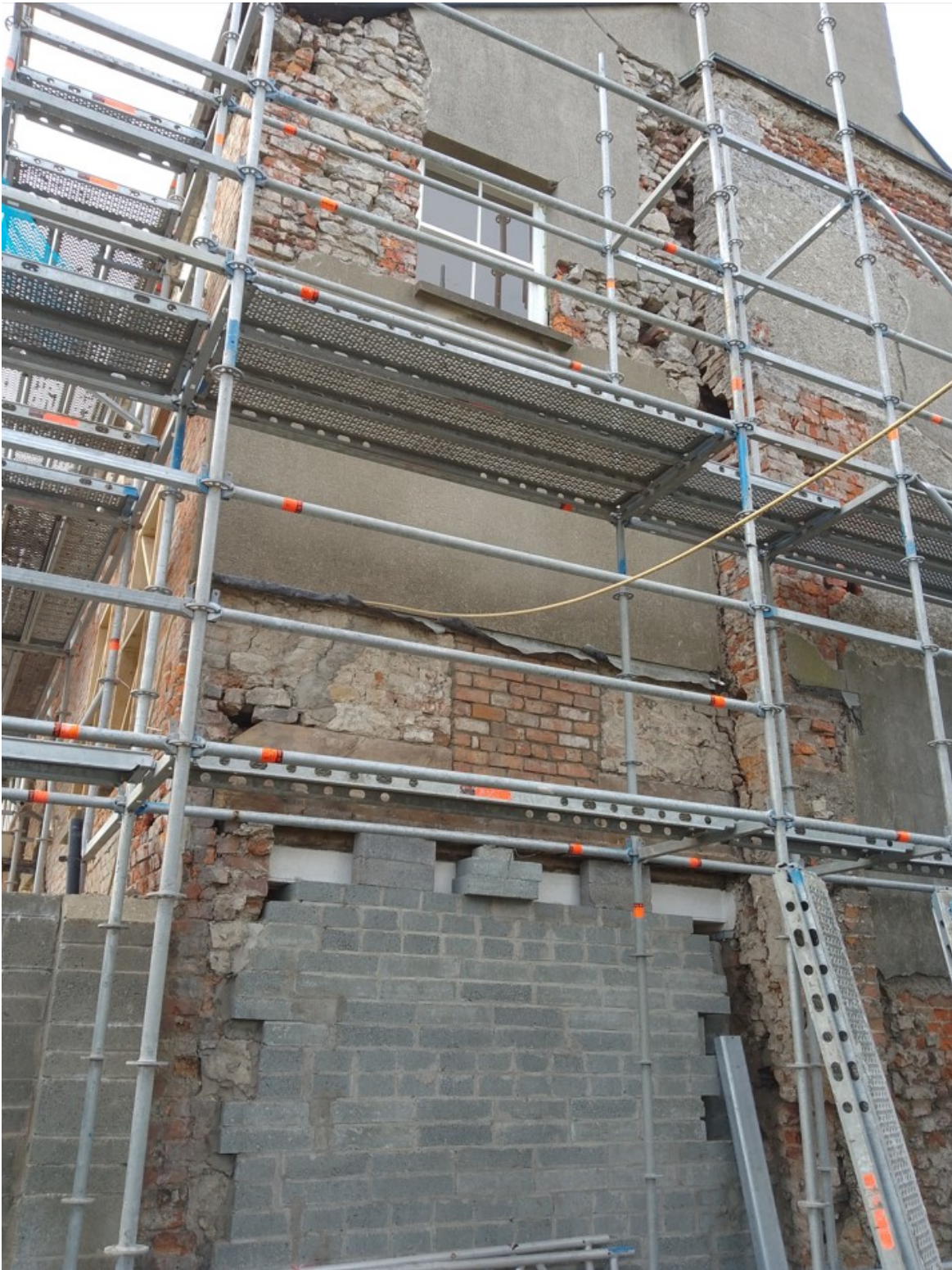
Figure 1 Southeast corner and gable wall
