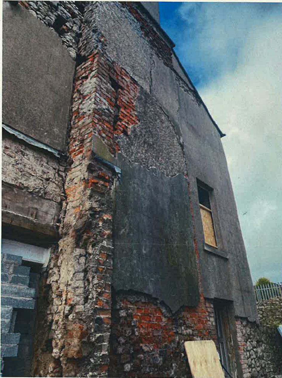
Figure 4 - View of the gable wall (East - South)
