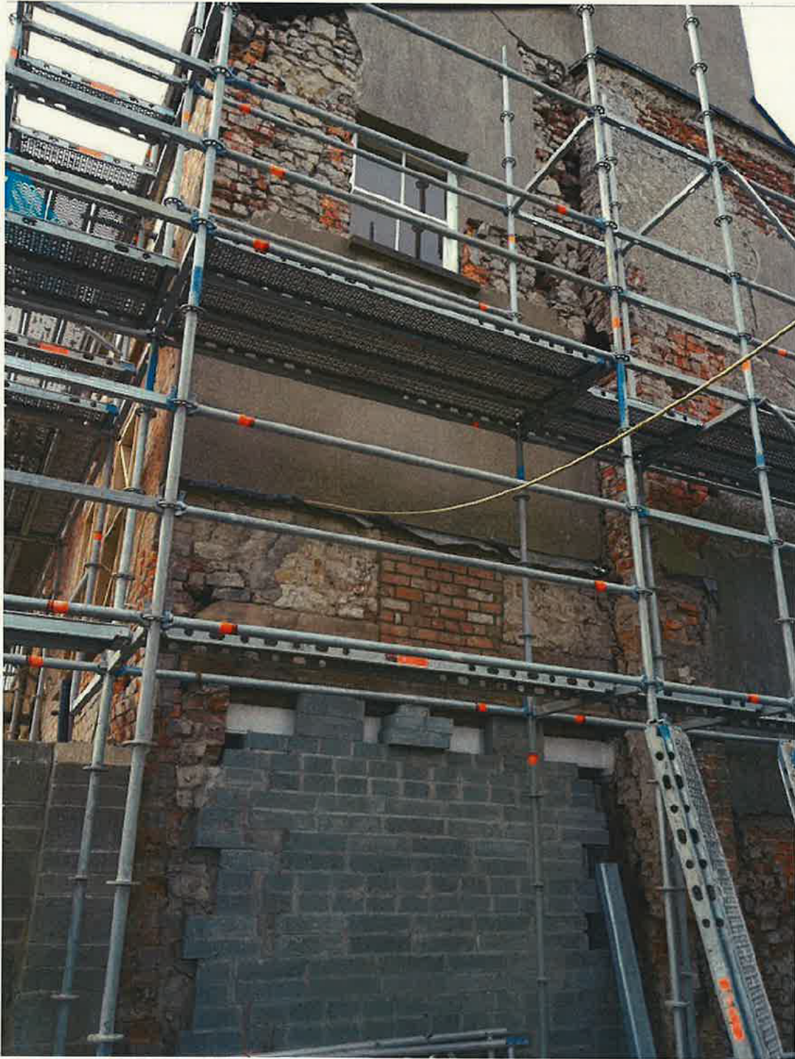
Figure 1 Southeast corner and gable wall
