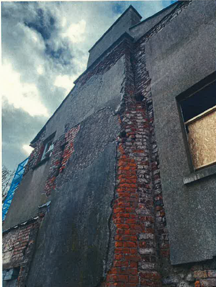
Figure 2 - View of the top of the Gable Wall (East – North)
