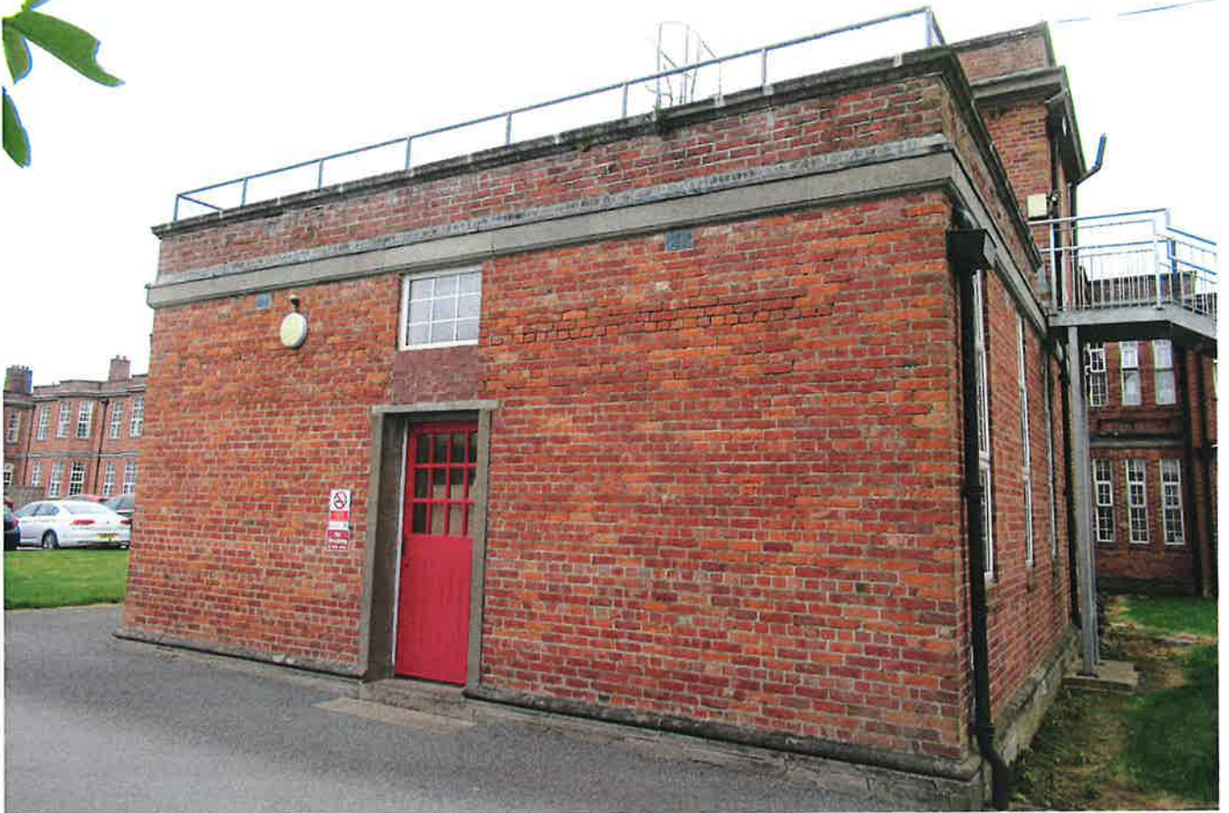
General view of roof 2
