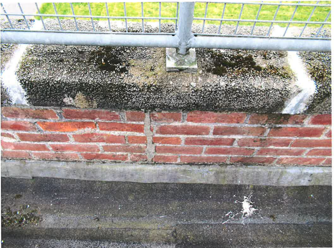
Interior view of parapet wall flat roof
