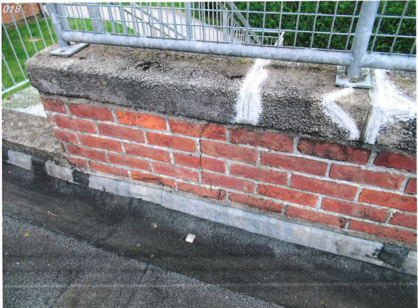
View of patch repairs to deteriorated lead work to flat roof 2
