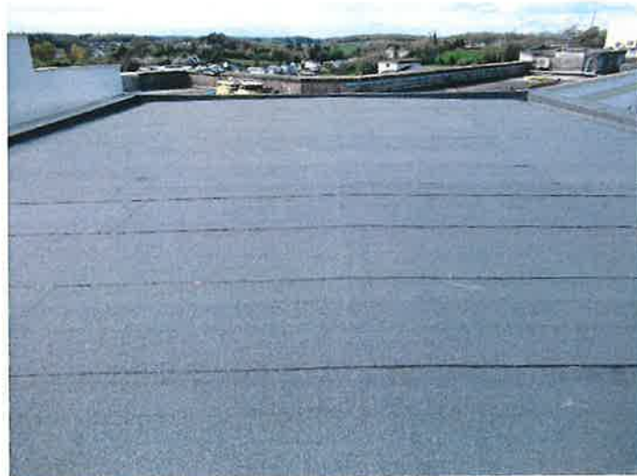
Typical image of newly felted flat roof when complete.
