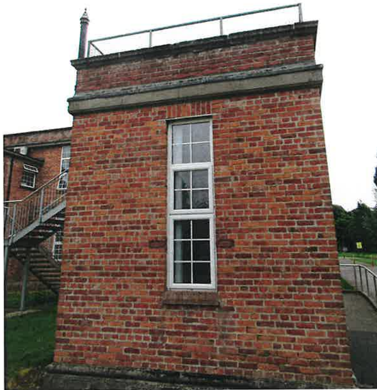
General view of roof no. 3
