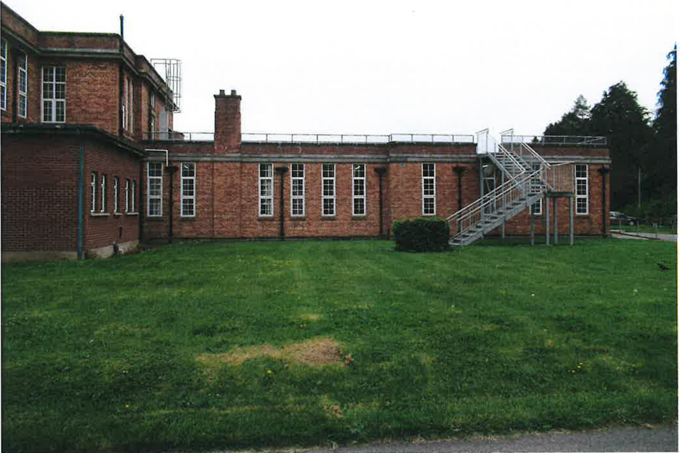
General view of roof 1
