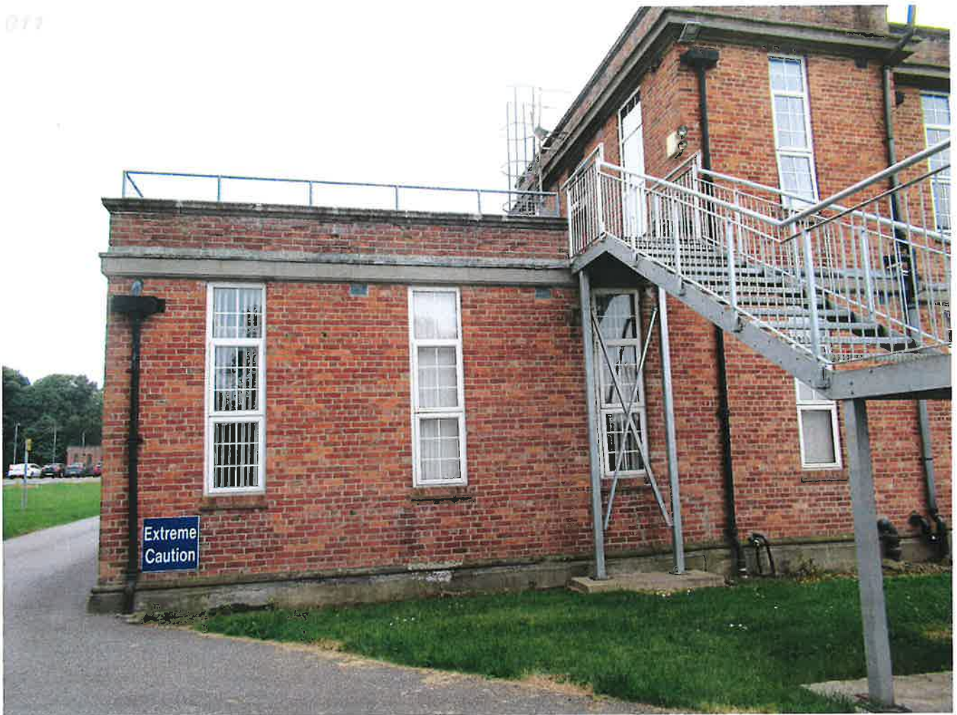
View of roof no. 2
