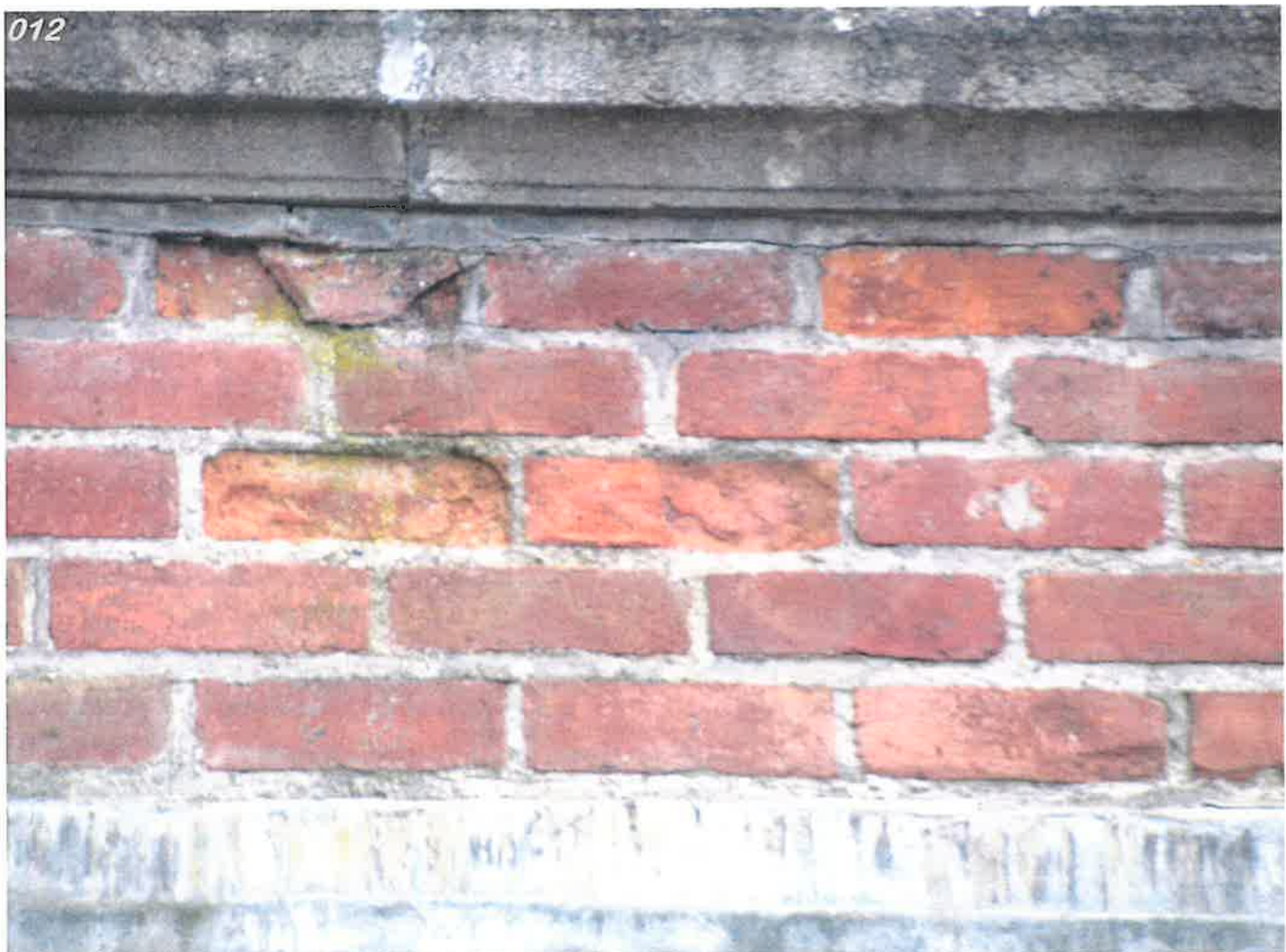
View of parapet wall to roof 2
