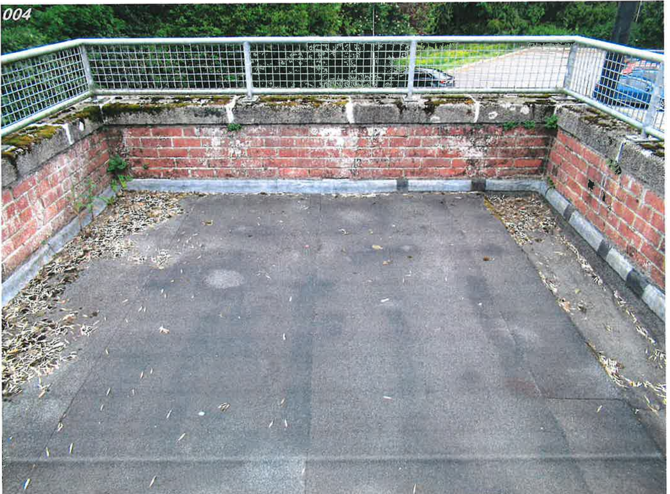
View of flat roofs inside parapet walls
