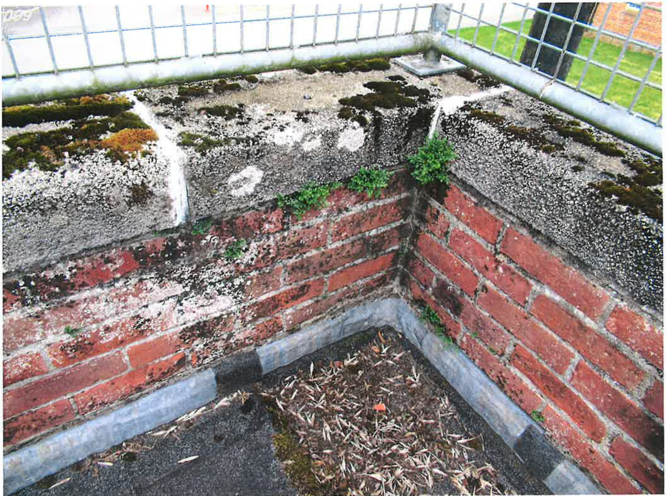
General view of brick work parapet walls and concrete cappings
