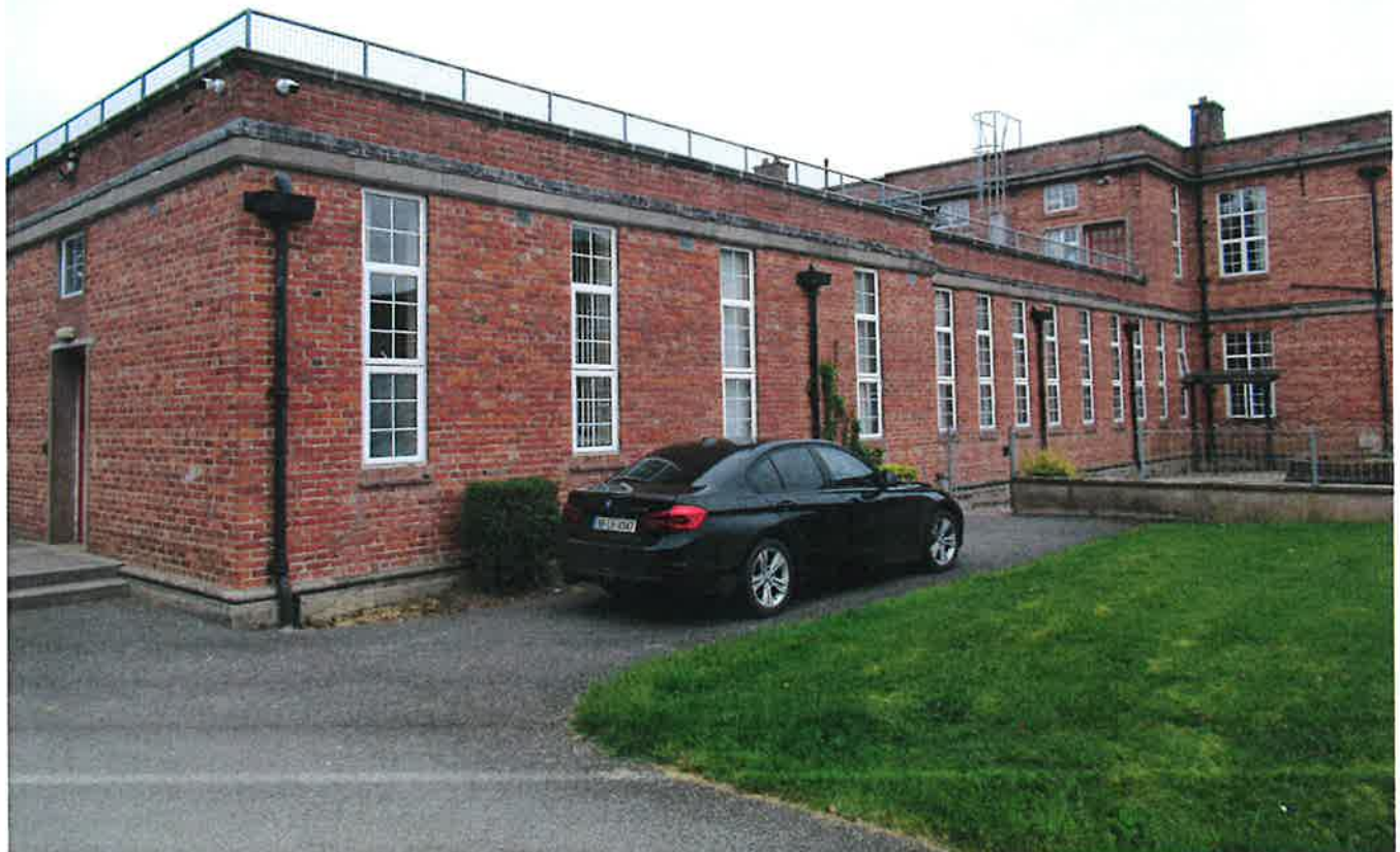
View of roof 1
