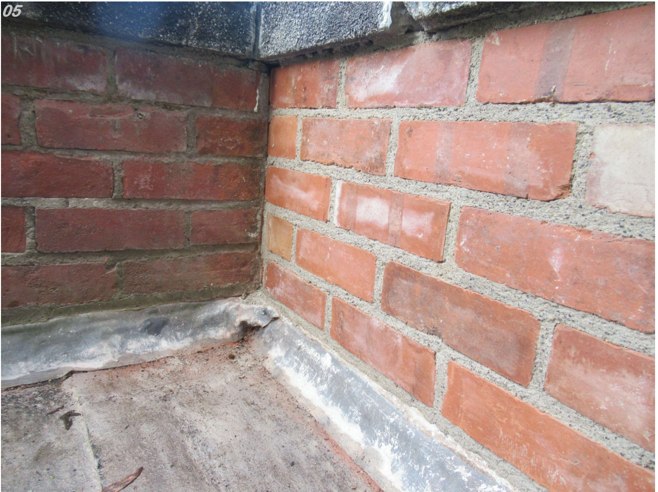
General view of newly constructed brick parapet using 'normanton brick'
