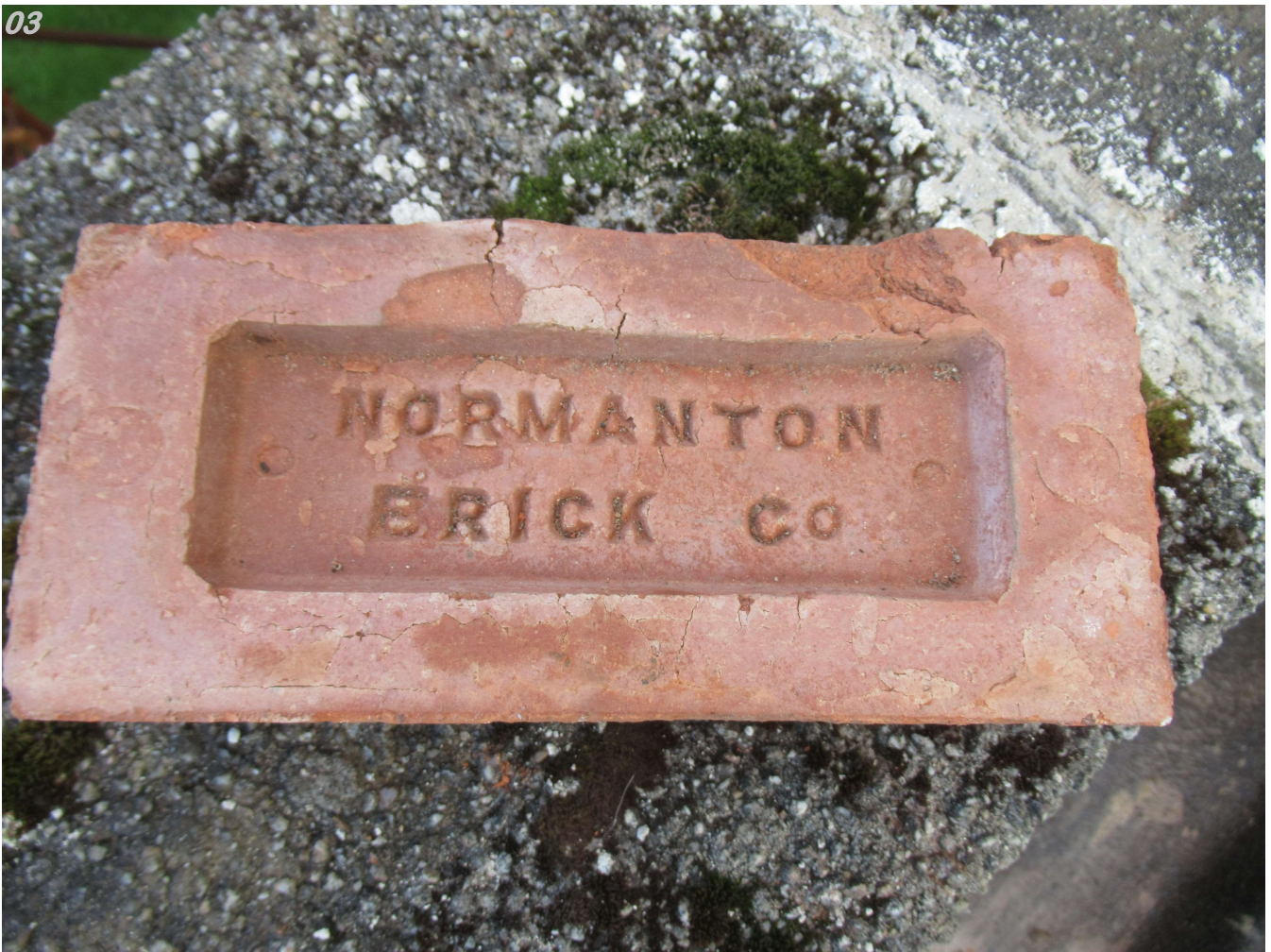
View of salvaged brick used in sample parapet
