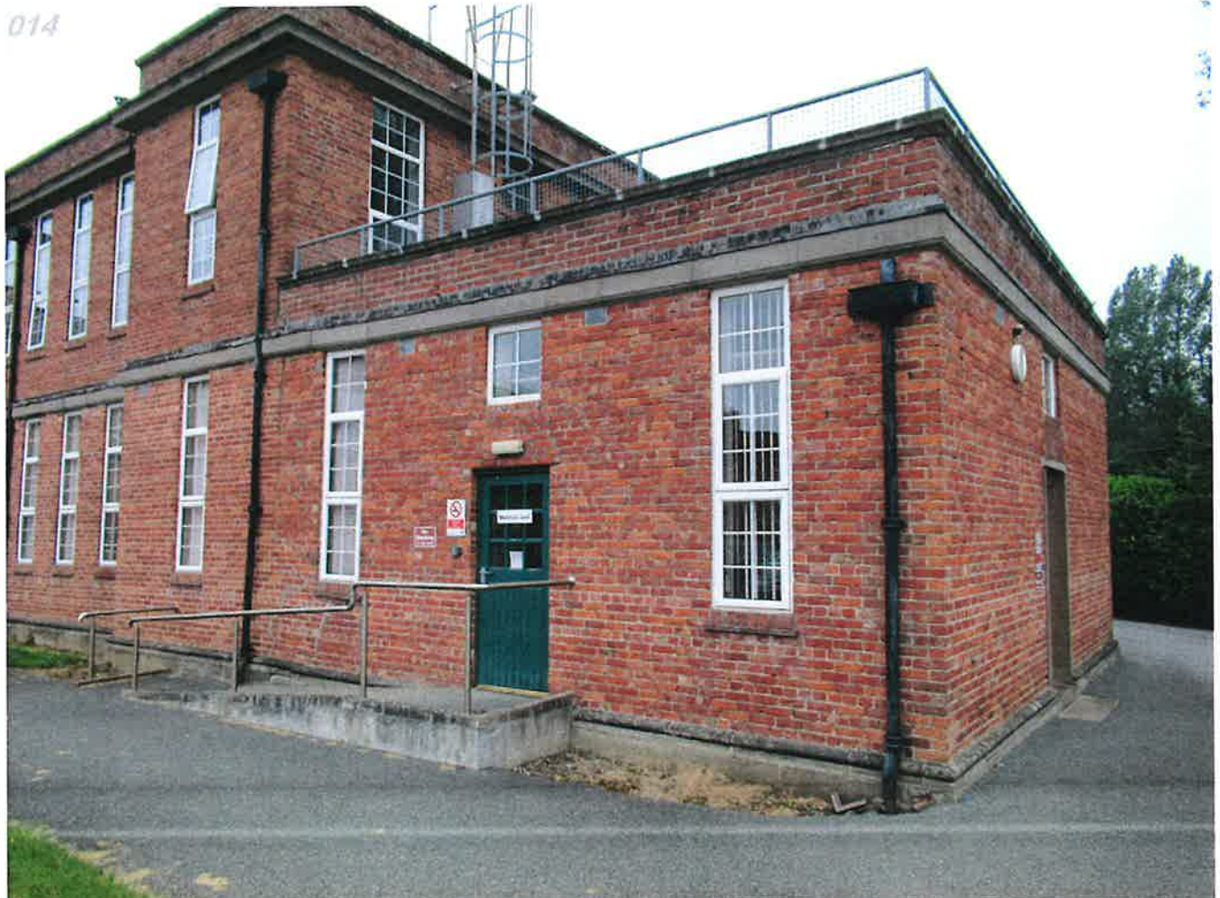
General view of roof 2
