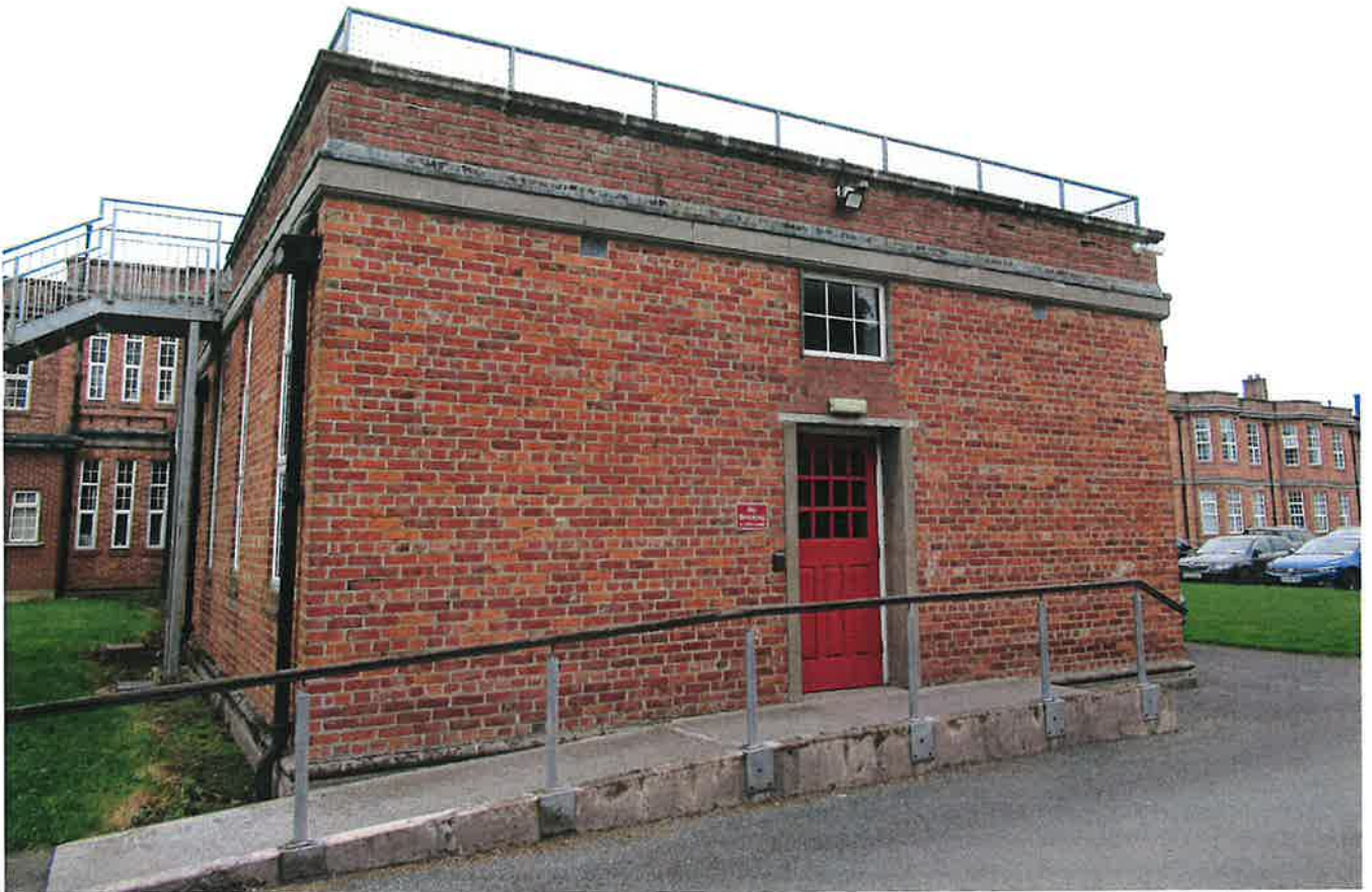
View of roof 1
