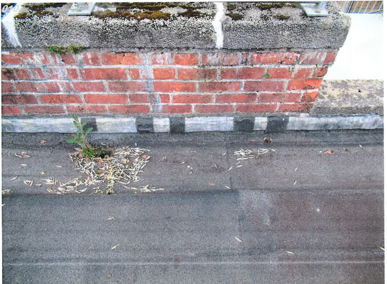
Various patch repairs to lead cavity trays
