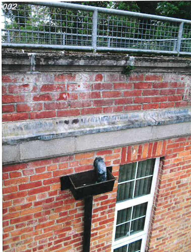
Parapet walls above lead line to be taken down and rebuilt
