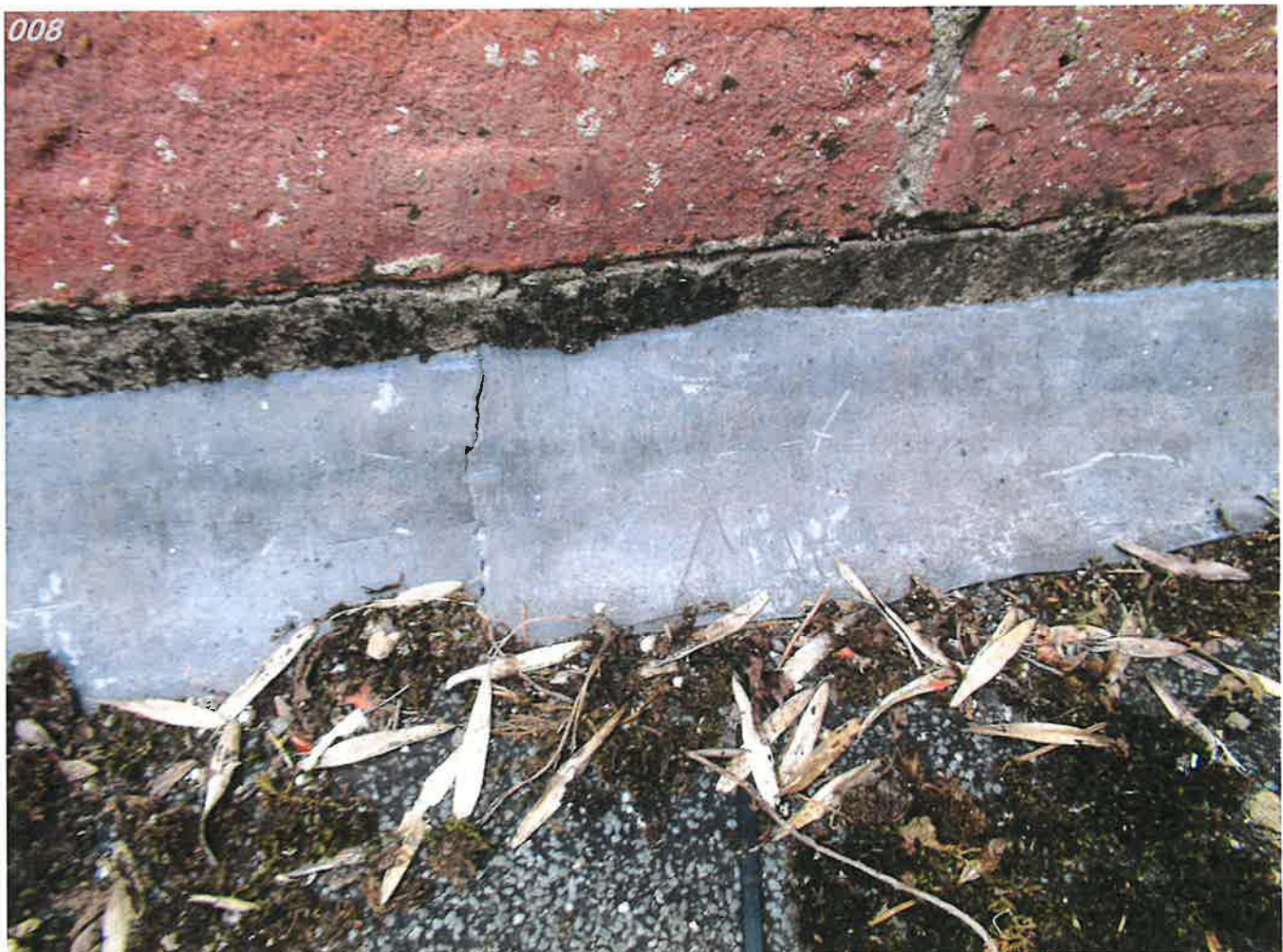
Tears to lead roof no. 3
