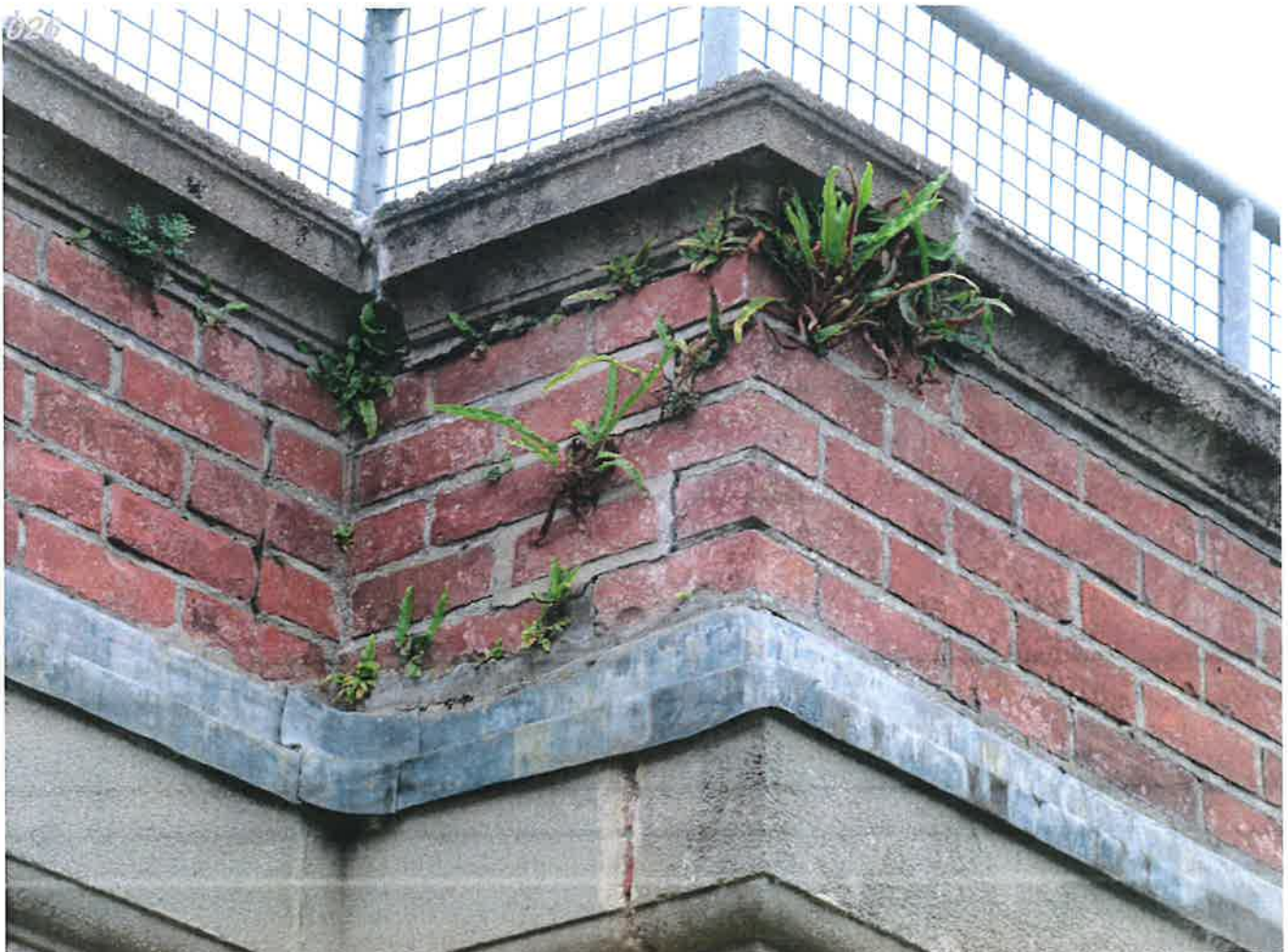
View of parapet walls
