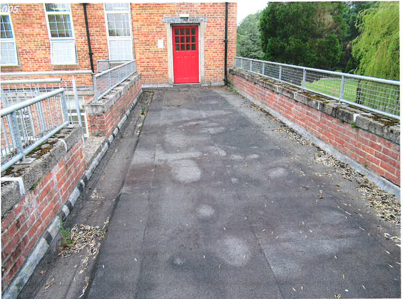
Interior view of flat roofs with perimeter parapet walls
