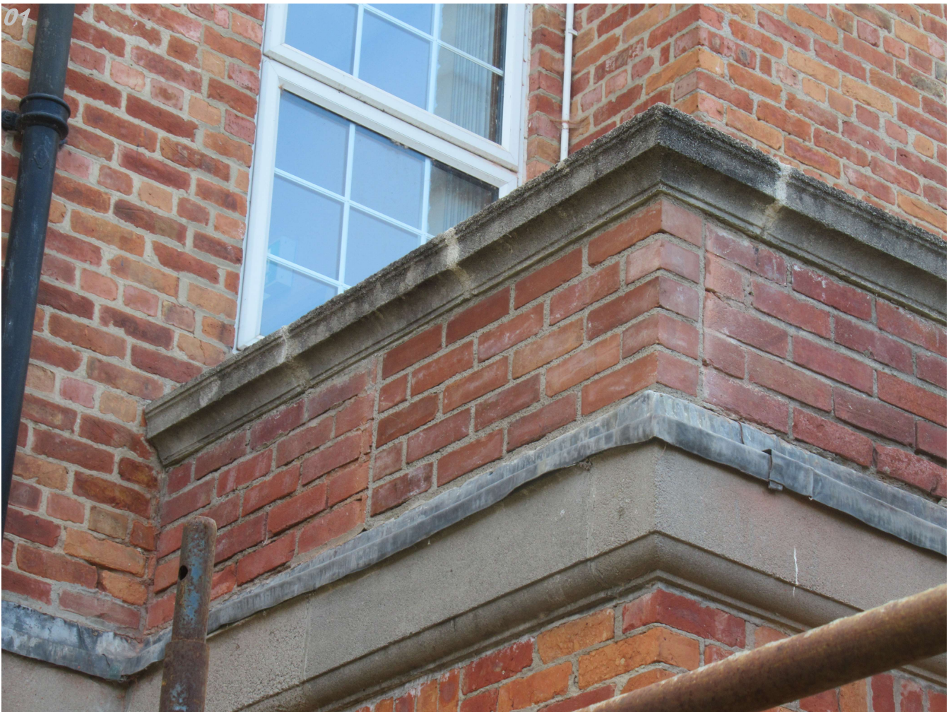
General view of newly constructed parapet wall with 'normanton brick'
