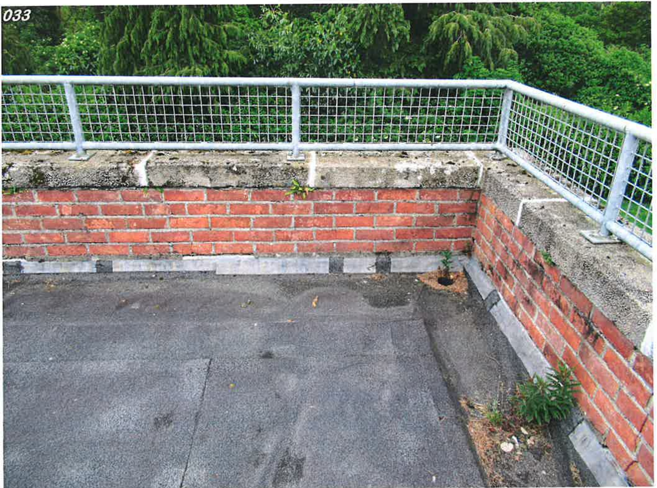
View of patch repairs to lead work
