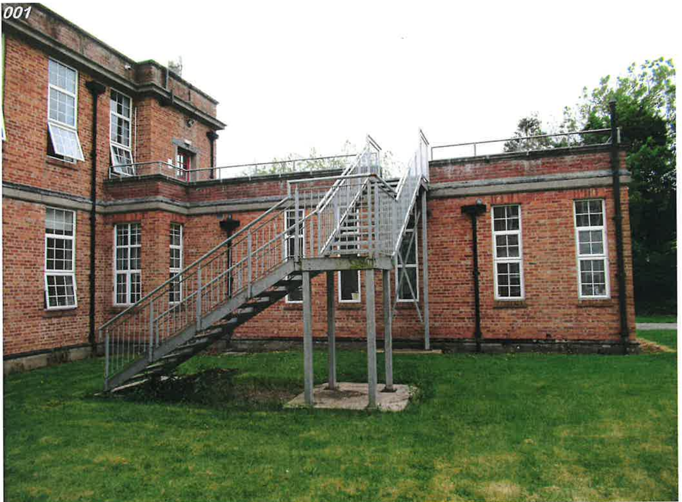
General view of roof 3 parapet walls
