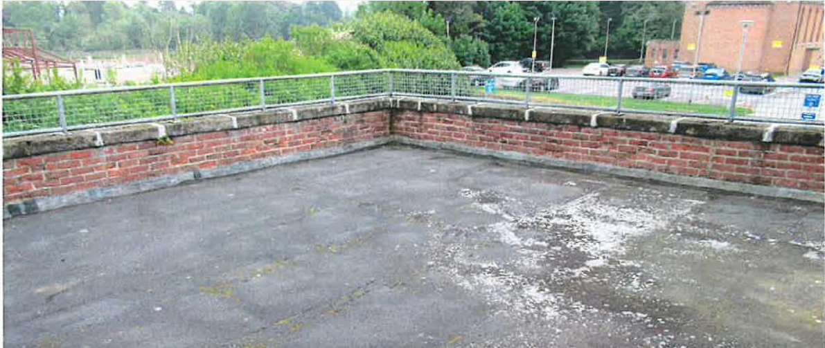
Current condition of roof 2.
