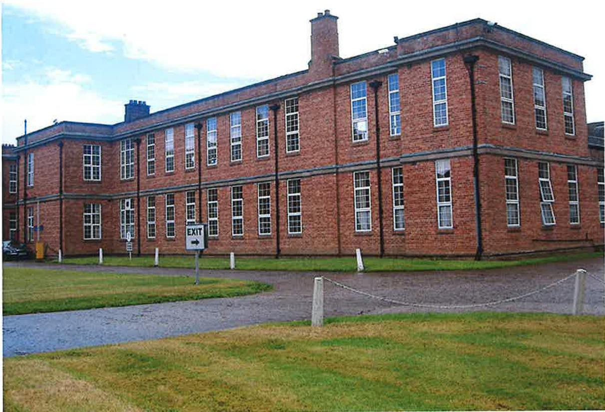
General elevation view of Saint Brigid's
