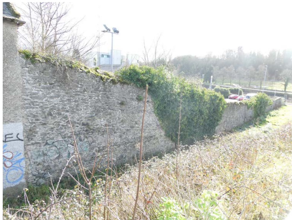
View of Town Wall from George's Street
