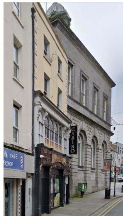
Shop Street 2025, Potential surviving upper level of historic shopfront
