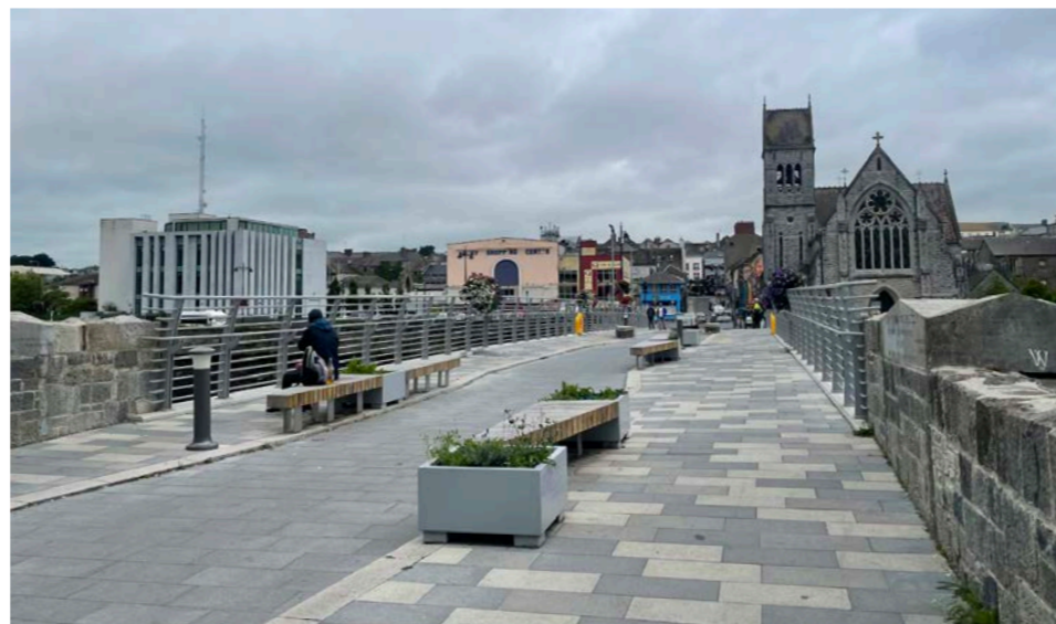
A number of modest scale interventions at Old Abbey Lane have transformed this special and unique place, making it attractive to visit and walk through, where previously it was somewhat of a backwater.
