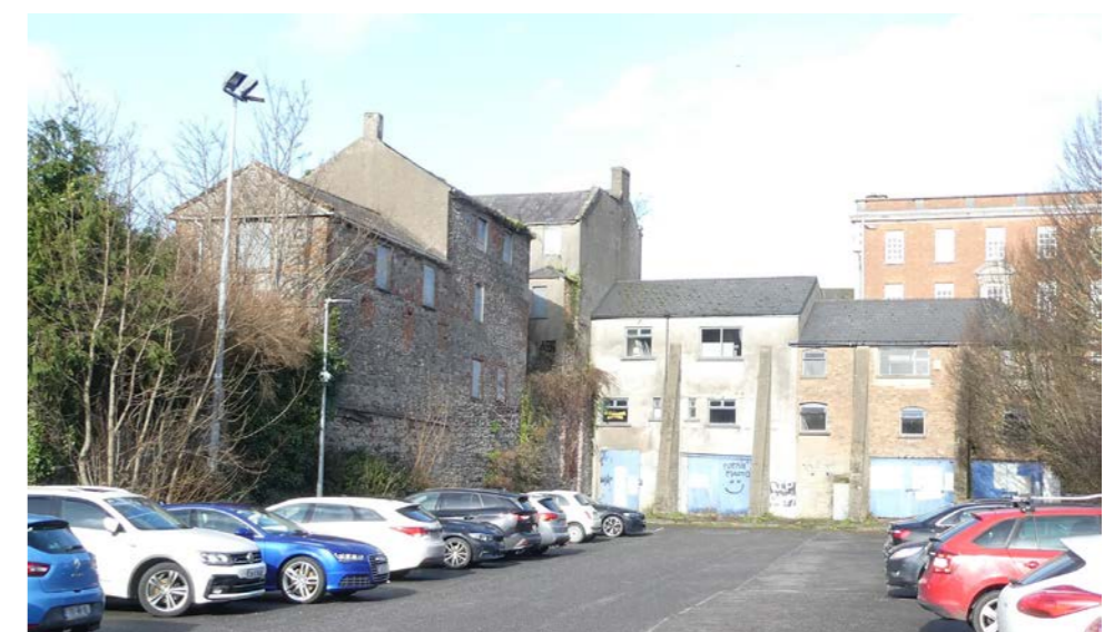
View from Murdock's Yard Carpark
