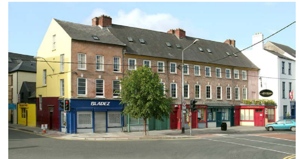
Fenns Quay Cork - Repair of 18th Century Buildings and Streetscape
