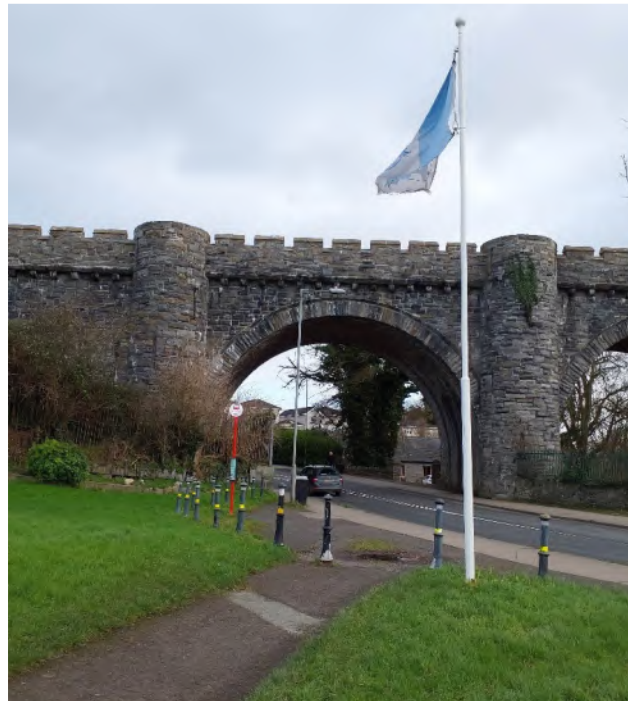
Plate 9. Ground photograph of the Newfoundwell Railway Viaduct bridge which is located approximately 103m east from the site boundary
