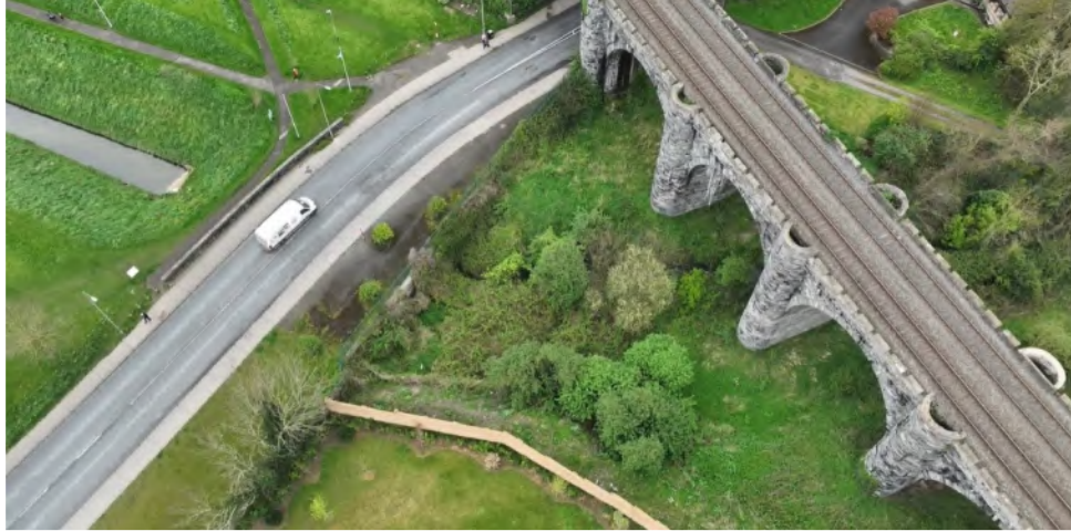
Plate 8. Aerial photograph taken in April 2024 at 60m elevation overlooking the Glen stream, which is culverted under the R166 and re-emerges under the Newfoundwell Bridge
