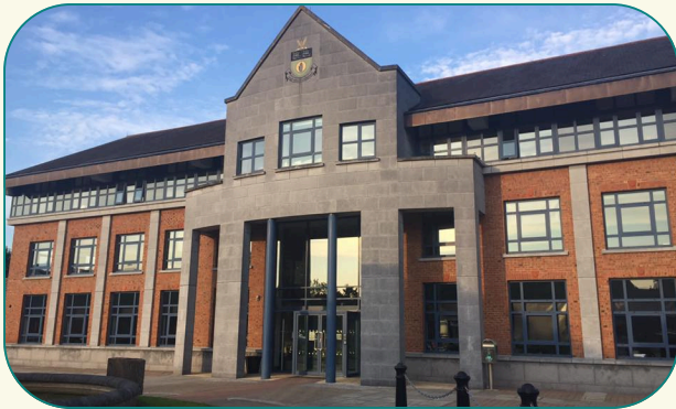
County Hall – Millennium Centre, Dundalk, Co. Louth (A91 KFW6)
