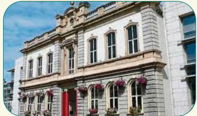
Townhall – Crowe Street, Dundalk, Co. Louth (A91 W20C)
