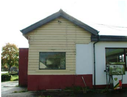
05201_03 AR&R 29/10/2007 North gable of station building.
