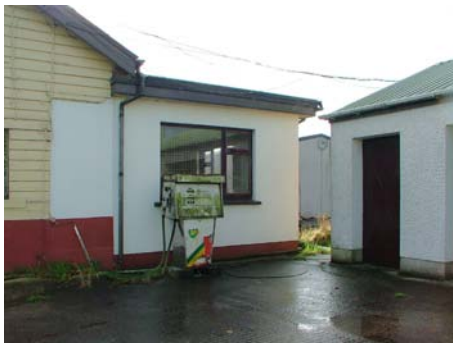
05201_04 AR&R 29/10/2007 Extension to rear of station building.
