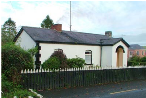
04201_17 AR&R 29/10/2007 Station house from SW.
