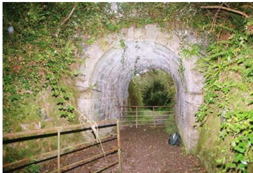
06210_01 FWH 20/09/2007 North-west elevation.
