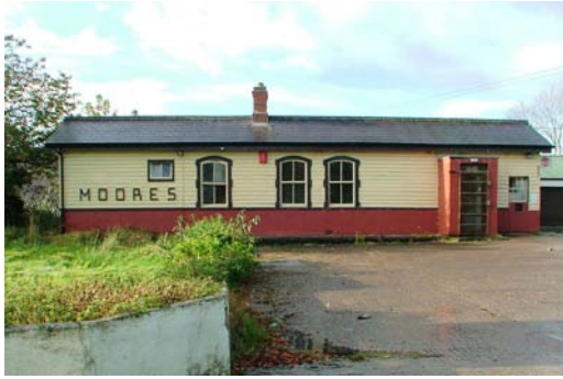
05201_01 AR&R 29/10/2007 View of station building from east.
