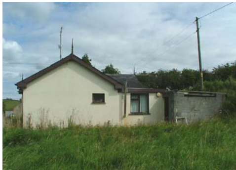
06201_23 AR&R 28/08/2007 Railway house 1: SW elevation.
