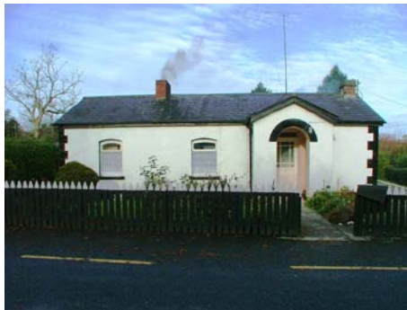
04201_16 AR&R 29/10/2007 Station house: front (SE) elevation.
