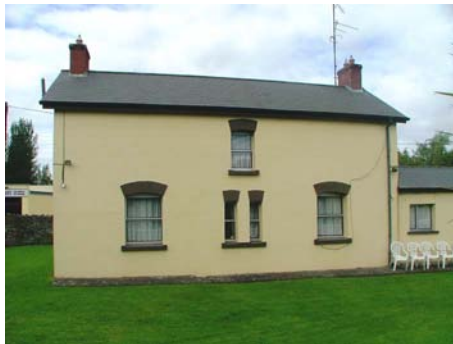
04301_41 AR&R 16/08/2007 Station house: south elevation.
