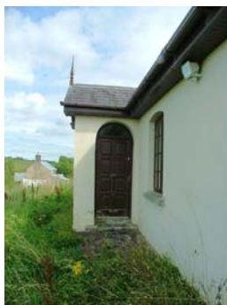
06201_24 AR&R 28/08/2007 Railway house 1: porch to front elevation.
