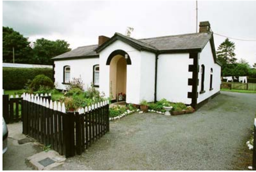
04201_15 FWH 02/07/2007 Station house from south.
