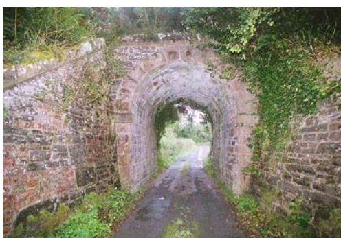
06212_01 FWH 20/09/2007 North-west elevation.
