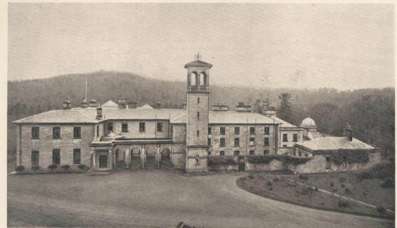
RAVENSDALE HOUSE (Front View).
