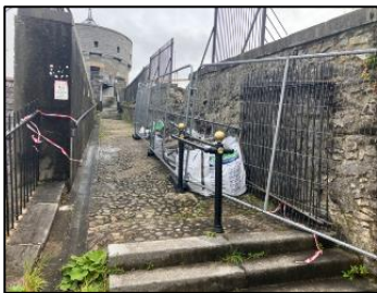
Photo: Wall Repairs at Millmount Drogheda
