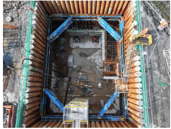
Aerial View of preparation for wall lift 1 concrete pour northern Bascule Chamber.
