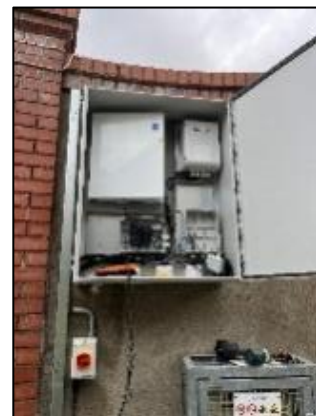
Photo: New Electrical Supply for Automated Gates at Fair St Machinery Yard Drogheda
