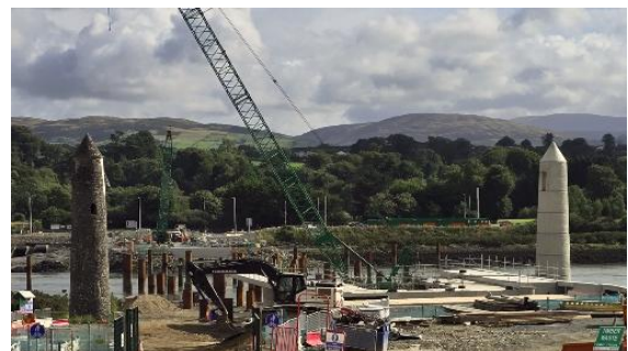
Installation of navigation beacon tower
