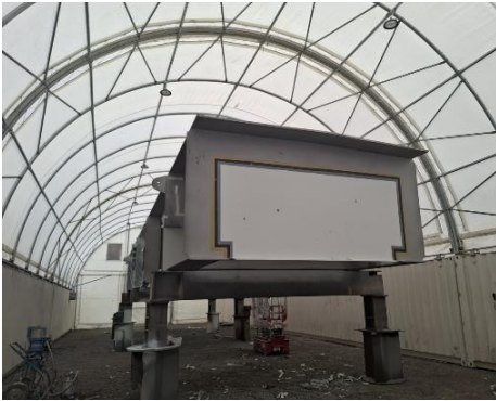
Commencement of painting of fabricated Fixed Span Sections.
