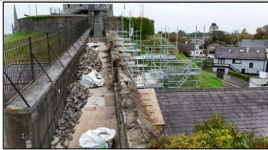
Photos: Repair Works to Walls at Millmount
