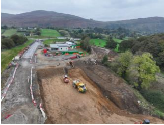
Temporary works for Crawler Crane platform have commenced, southern embankment.
