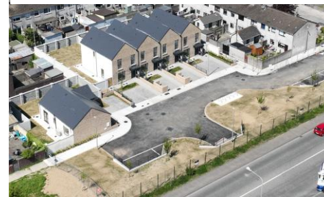
Muirhevnamore Infill, Dundalk – LCC Direct Build 11 Units
