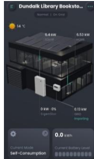
Graphic: Power use at the Bookstore at the County Library – 6.53KW is being used in total, of which 6.4KW is being generated from the new SPV and 0.13KW is being imported from the national grid – demonstrating reduced demand from the national grid.
