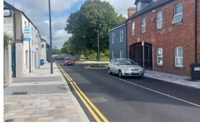
New road surfacing on Linen Hall Street.
