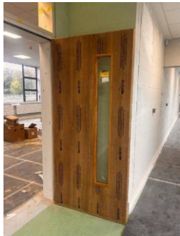
Internal dooring ongoing.
