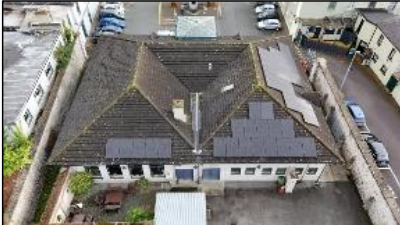
New solar PV at Ardee Library and Carlingford Library and Courthouse
