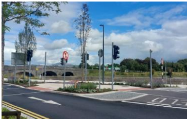
New road surfacing and traffic lights at the Tain Apartments.
