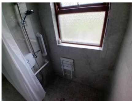
Bathroom Adaptation completed in Drogheda, with funding provided with a HAG
