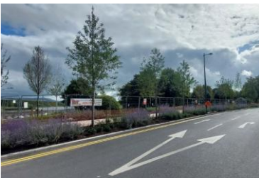
New road surfacing and traffic lights at the Peace Park.
