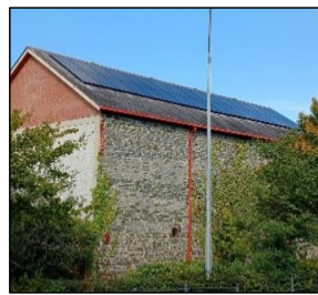
Photo: Installing Solar PV at Dundalk Library Bookstore
