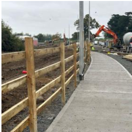
Progress on Footpath and road works ongoing.
