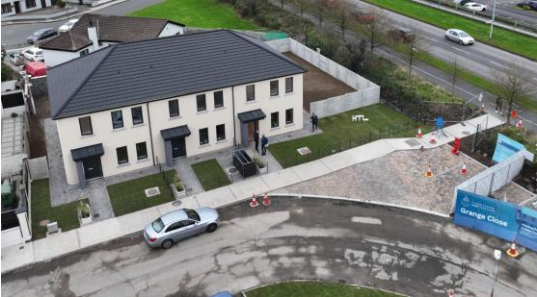
Grange Close, Dundalk – 3D Concrete Printed Houses – LCC Direct Build
