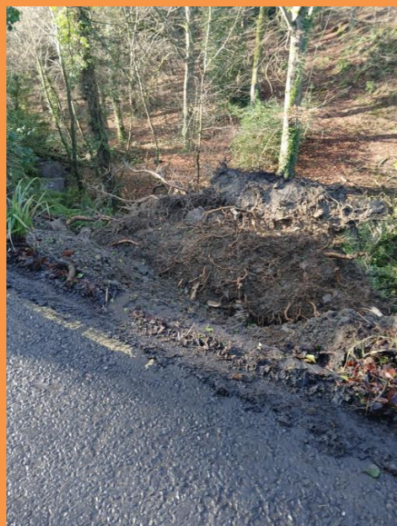
Photo – prior to works
