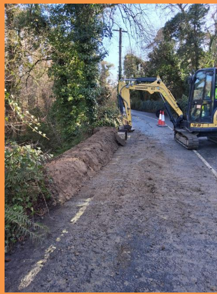
Photo – works completed
