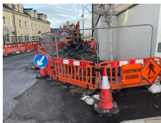
Works ongoing to Bridge St. Phase C (RHS)
