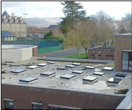
Photo: A View from the training tower showing 19 of 23 (total) new A+ Energy-Rated Rooflights at Dundalk Fire Station.
