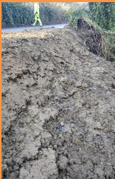
Photo – during works
