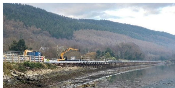
Substructures complete between border and Rough Island
