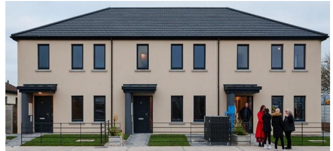
The 3DCP houses at Grange Close, Dundalk
