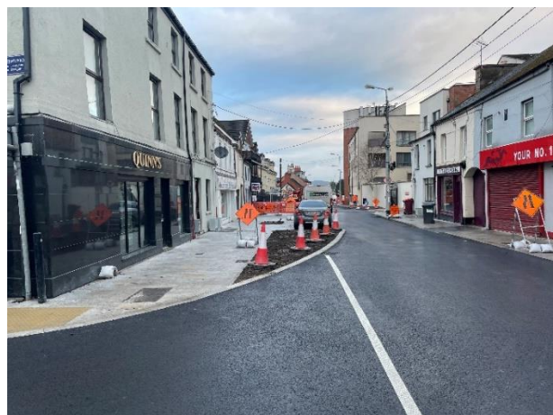
Works Complete to Bridge St. (Phase B)
