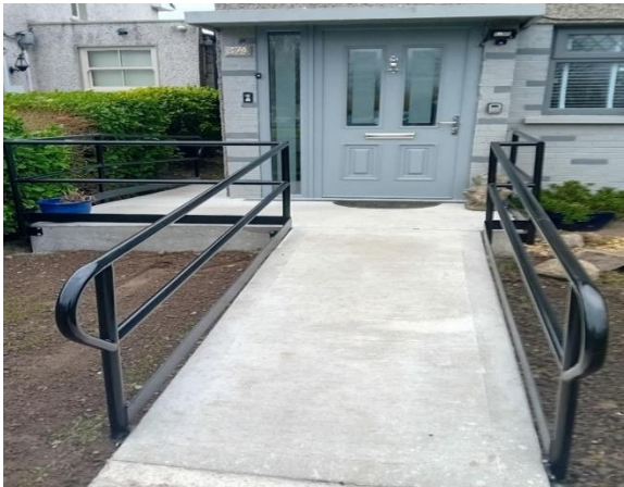
Access Ramp completed in February 2025 in Drogheda, part-funded with a HAG
