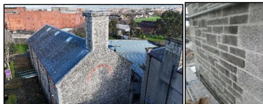
Photos: New Works to reduce Water Ingress at Oriel Centre Dundalk
