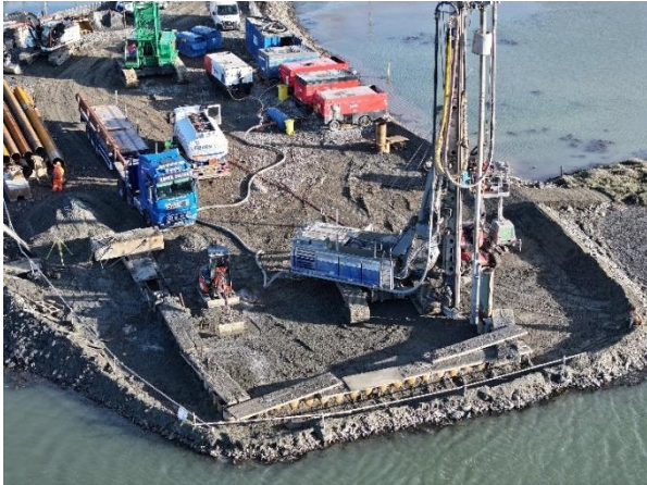
Piling Platform Northern Embankment
