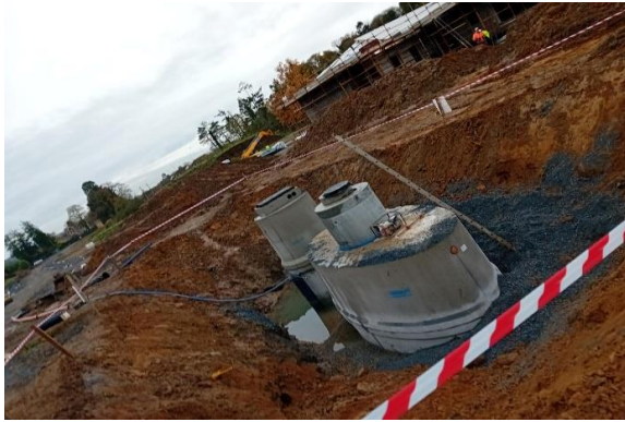
Sewage Pumping Station under construction
