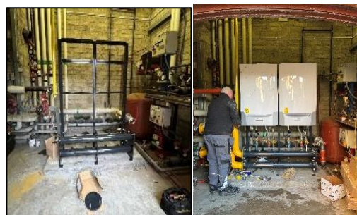
Works in progress to replace the gas boiler at Dundalk Museum with a temporary gas boiler system
