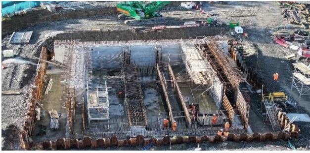
Southern Abutment ongoing R.C. works
