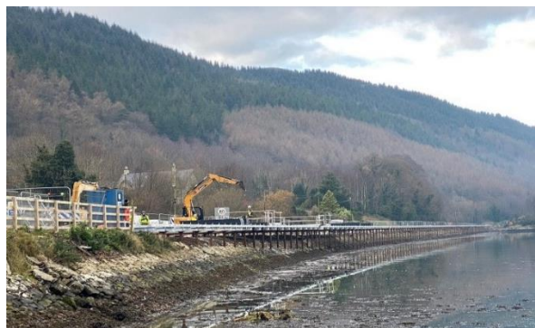
Substructures complete between border and Rough Island
