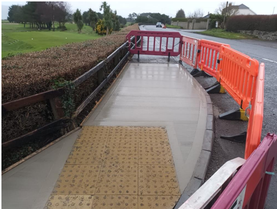
Footpath improvement works at Greenore
