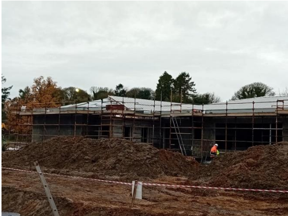
School Roof under construction
