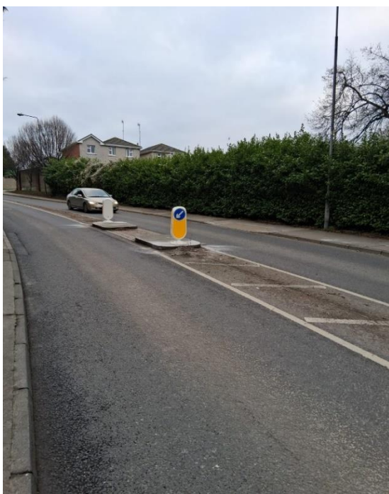
Bollards replaced at Termonefeckin
