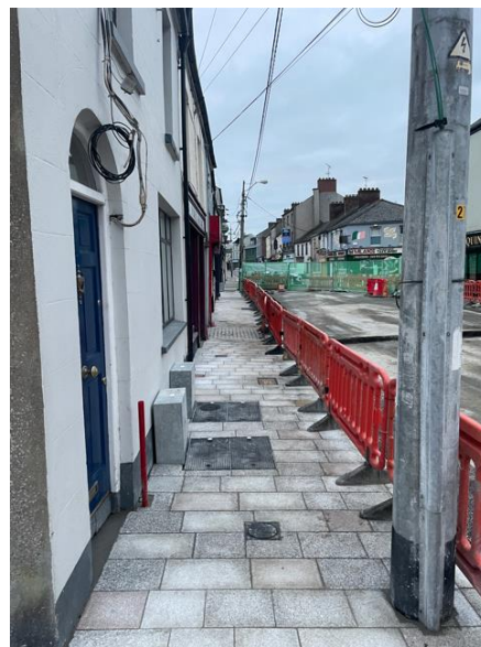
Works as they are being completed to Bridge St. (Phase B)
