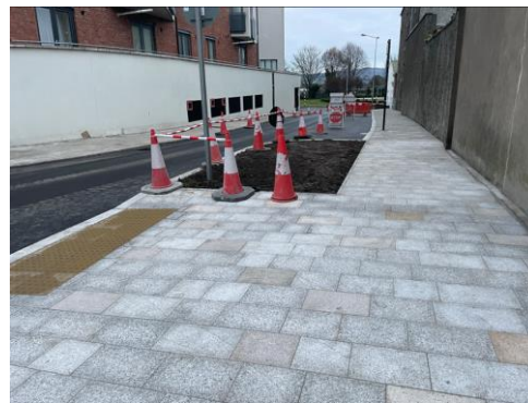
Works as they are being completed to Northgate St. (Phase D)
