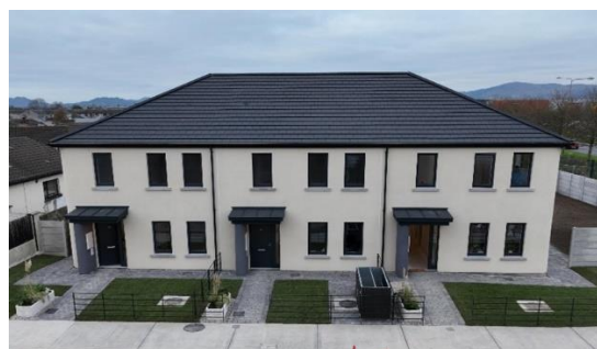
Grange Close, Dundalk – completed 3D Concrete Printed Housing
