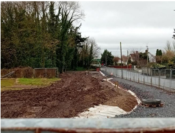
Access Road under construction
