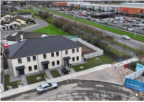
Grange Close, Dundalk – completed 3D Concrete Printed Housing
