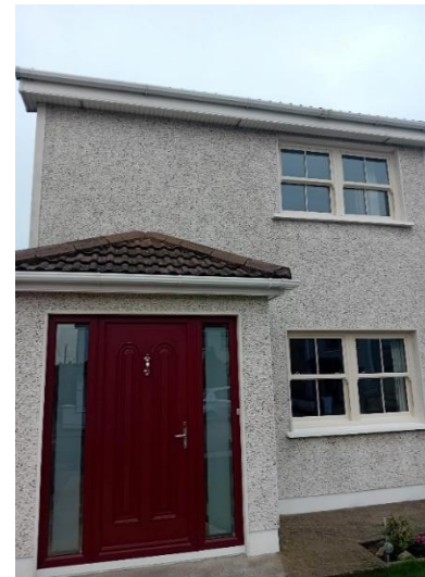
New Windows and door completed in Drogheda, with funding provided with a HOP
