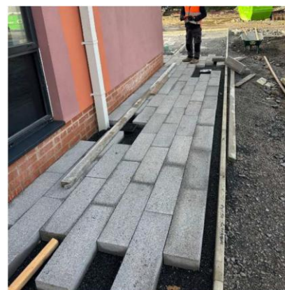
Progress on Footpath ongoing.
