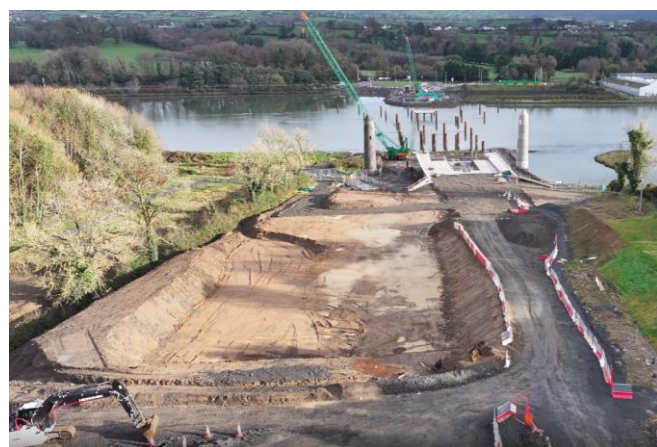
Temporary works for Crawler Crane platform ongoing, southern embankment.
