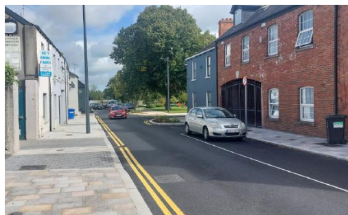
New road surfacing on Linen Hall Street.
