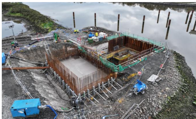
Aerial View of northern Bascule Chamber and commencement of the concrete for the Plant Room.
