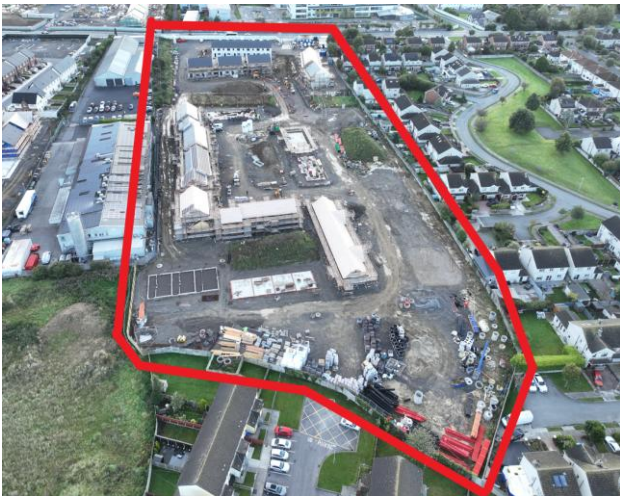
Bakery View, Drogheda – LCC Direct Build 97 Units
