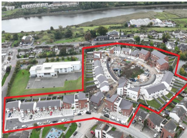
Boice Court, Drogheda – LCC Direct Build 72 Units
