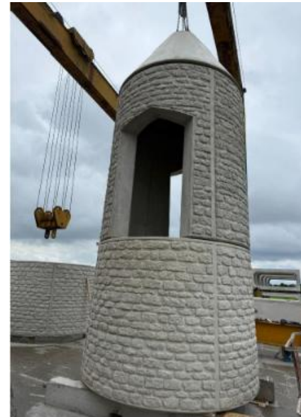
Offsite Fabrication of top section of the navigation beacon tower
