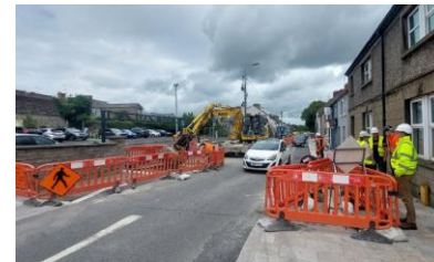
Utility works ongoing to Linenhall St.
