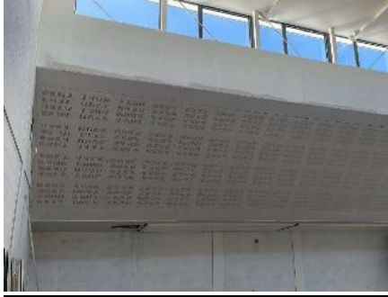
Commencement of internal Painting
