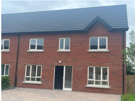
Part V Housing in a residential development, Ballymakenny Area, Drogheda
