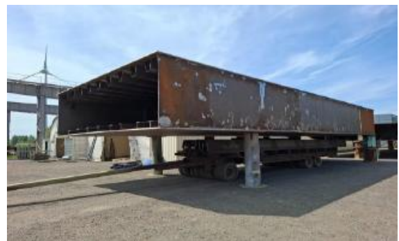
Offsite Fabrication of top section of the navigation beacon tower
