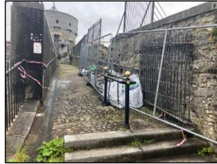
Photo: Wall Repairs at Millmount Drogheda
