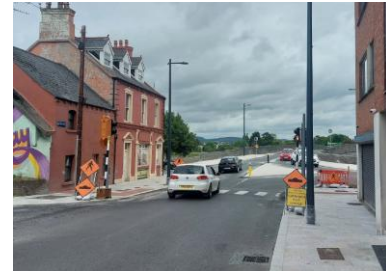
Looking North with Bride Works Complete
