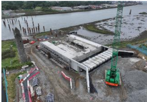
Southern Abutment with Greenway Underpass
