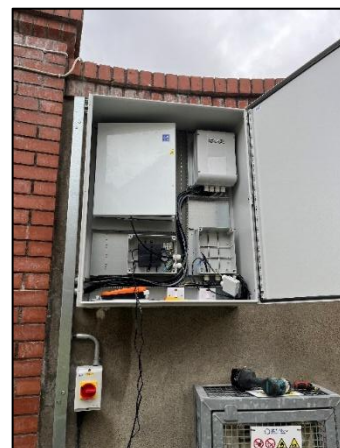
Photo: New Electrical Supply for Automatic Gates
