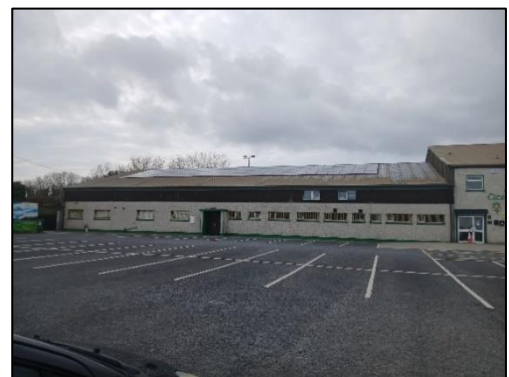
Solar Panels recently installed at the Cooley Kickham's GAA Club.
