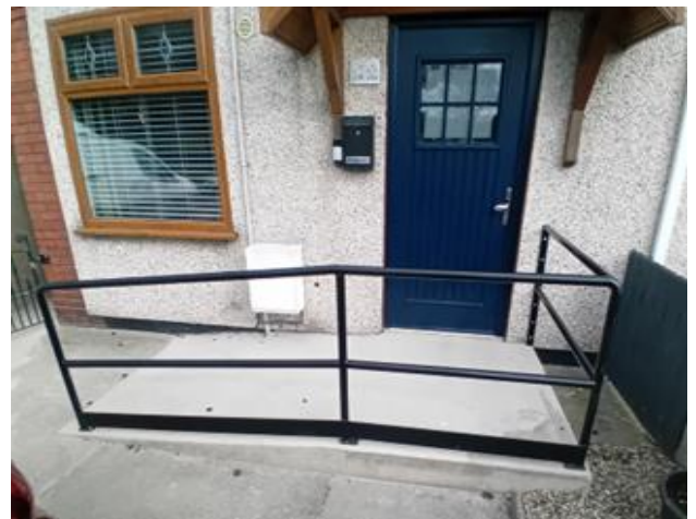
Access Ramp completed in March 2025 in Dundalk, part-funded with a HAG
