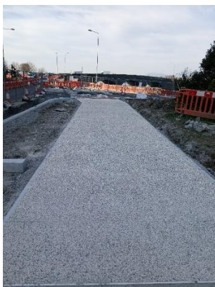
New exposed aggregate concrete at Fairgreen
