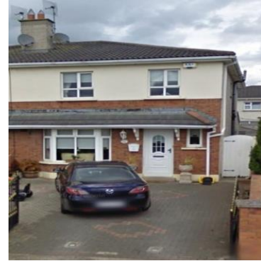
Recently purchased house in Drogheda
