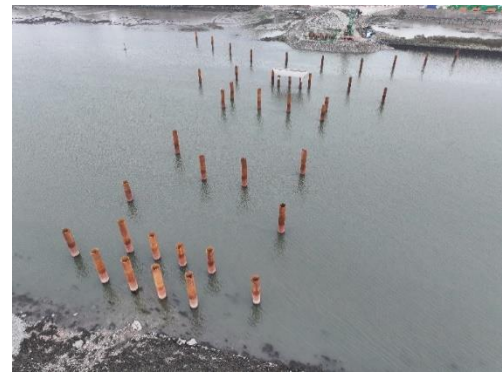
Completed Marine Piling Works
