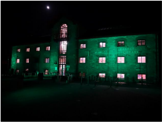
Photo: Dundalk library all dressed in green for St-Patrick's Day using the new lighting system installed as part of their #VisionarySolution 2! #Varcities
