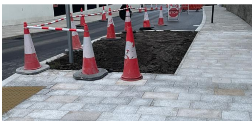
Works ongoing to Northgate St
