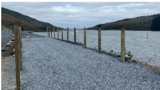
Approaches to boardwalk under construction
