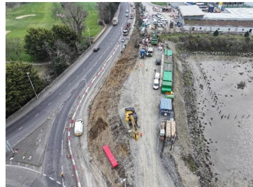
A2 Filter Lane Construction
