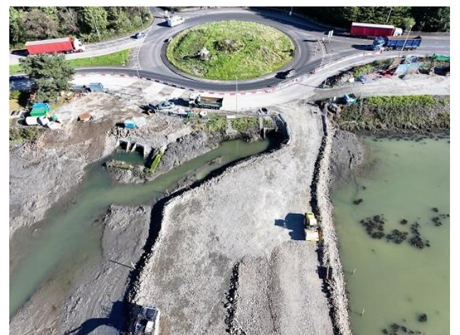
Embankment Works Northern Approach.
