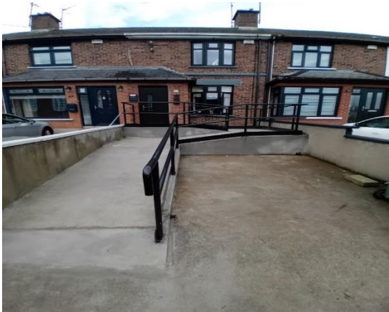
Access ramp in Drogheda completed in October part-funded by a HAG
