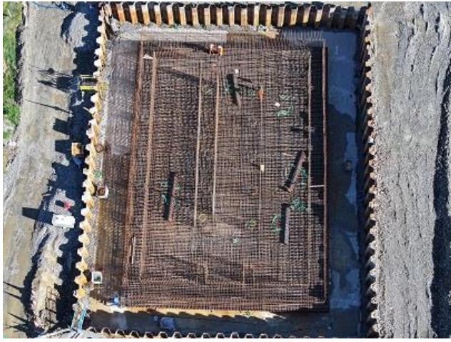
Reinforcement Works Southern Abutment
