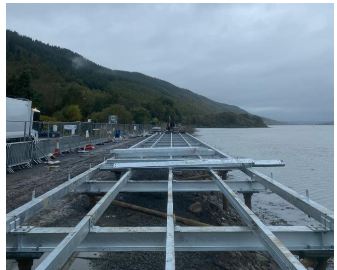
Substructure of Boardwalk being assembled
