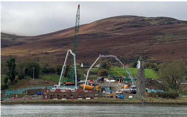
Concrete Pour Operation Southern Abutment
