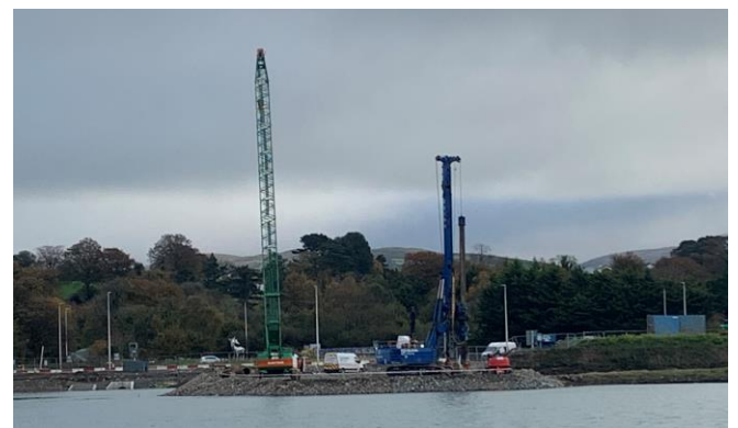
Piling Platform Northern Embankment
