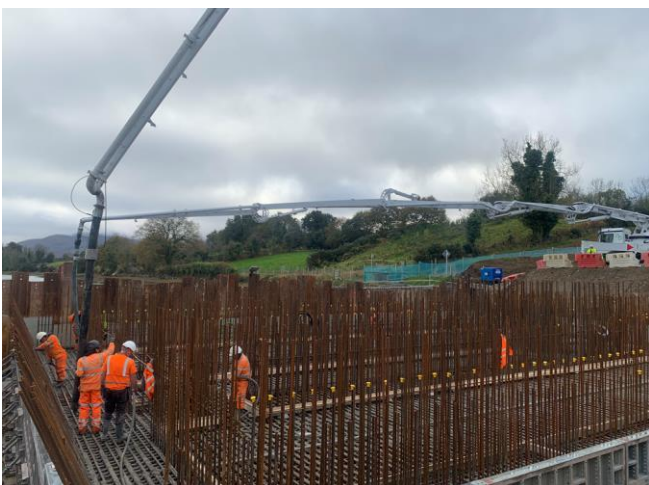
Concrete Pour Operation Southern Abutment
