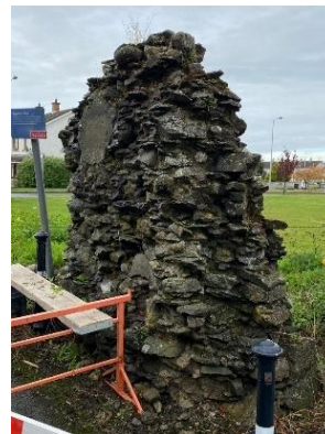
Before (south side)
