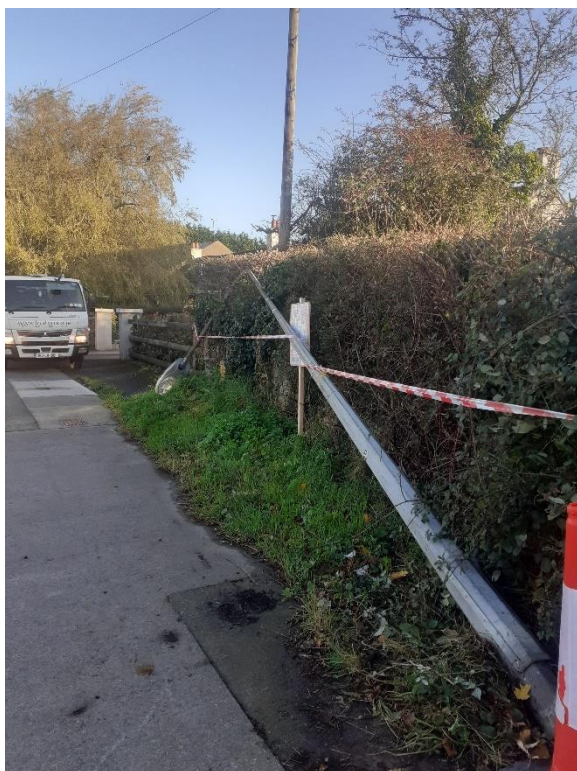
Storm Ashley damage – Ballymakellett Road
