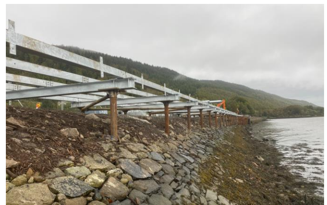
Substructure including Piles
