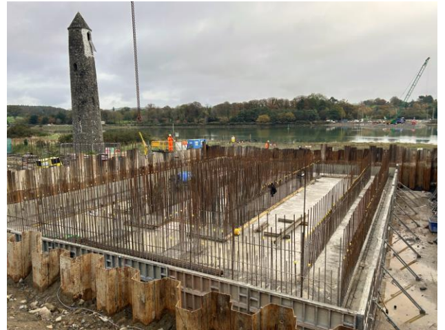
Finished Concrete Pour Southern Abutment Base
