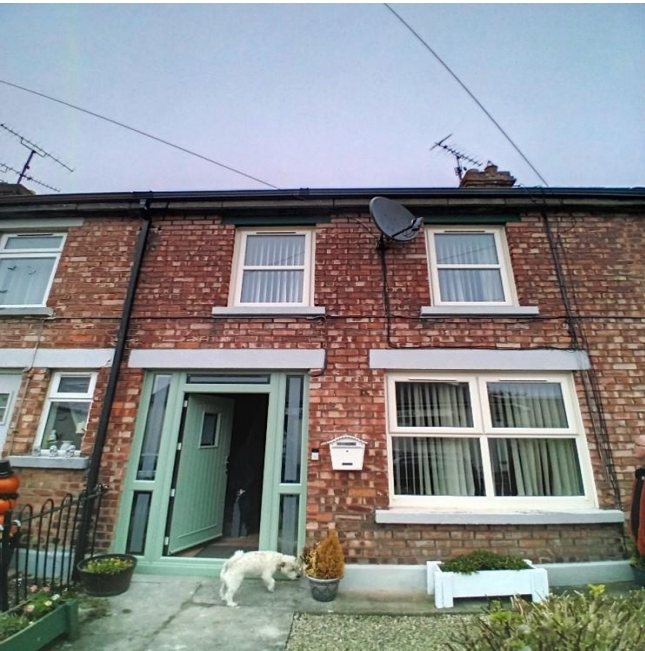
New Windows and door fitted in Dundalk in October funded by a HOPS
