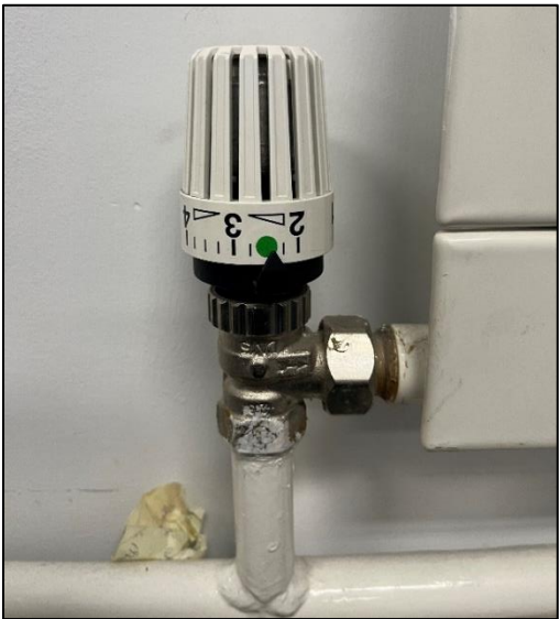
Green mark denotes the optimum setting ('sweet spot') for this radiator
