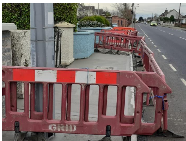
Footpath works at Avenue road, Dundalk
