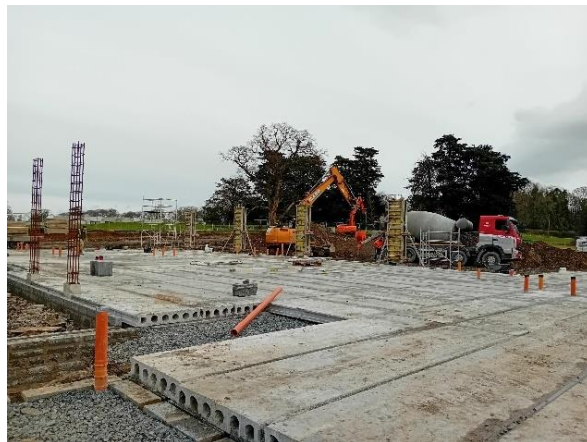
Floor slabs in place in preparation for Radon membrane
