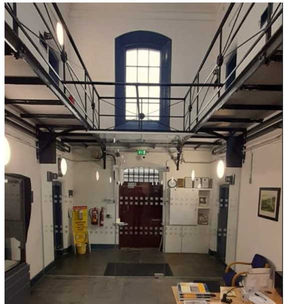
New Draught Lobby at the Council's Archives Building
