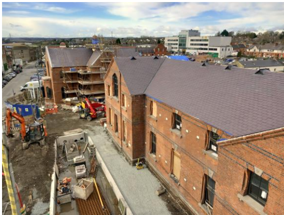
Block C New Roofing
