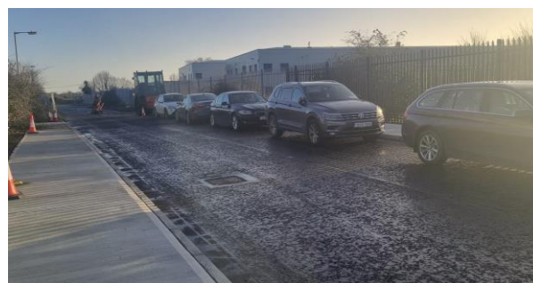
New carriageway with footpaths
