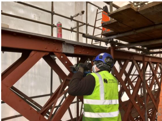
Drilling for repair section to Lattice Members Obelisk Bridge Section of primed steel
