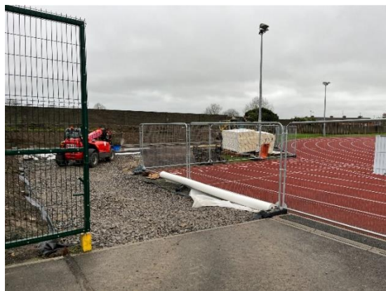
Capital works continues at Lourdes Athletic Stadium
