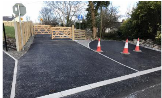
Access control gates installed at culvert/
