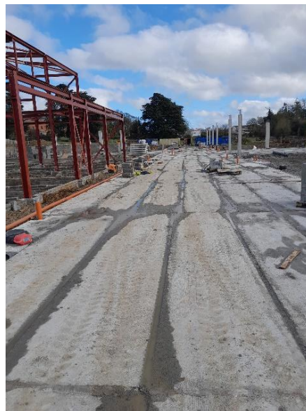
Steel frame to General Purpose Hall
