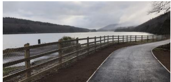
Works Complete in Victoria Lock in NI
