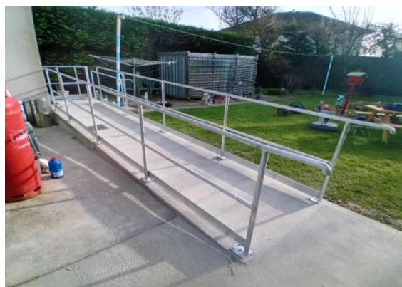
Ramp completed in February in Dundalk, assisted with a Housing Grant for a Disability.
