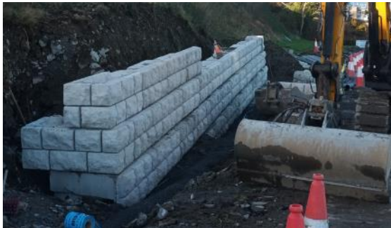
Retaining wall works in Section 1 Carlingford
