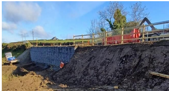
Stabilisation works the R132 at Mullary near the Village Inn
