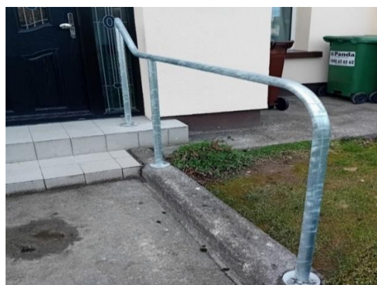
Handrail installed in February in Drogheda with the support of a Housing Adaptation Grant.
