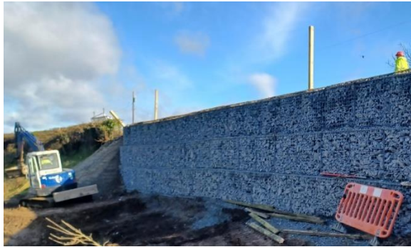
Stabilisation works the R132 at Mullary near the Village Inn
