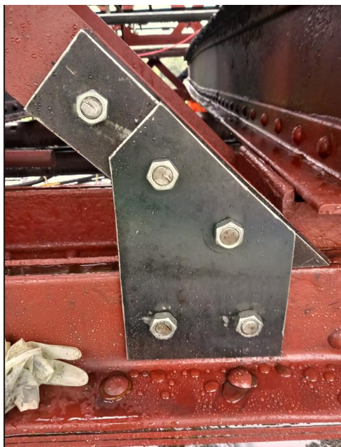
Template for Lattice Repairs
