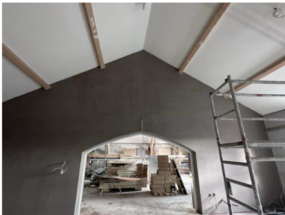
Block C Internal Fit out
