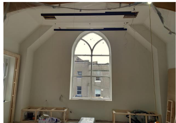
Fitout of New MD Meeting Room ongoing
