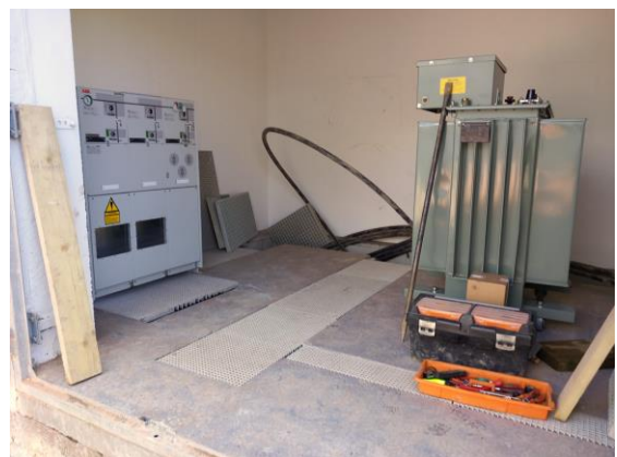
ESB switch gear now installed
